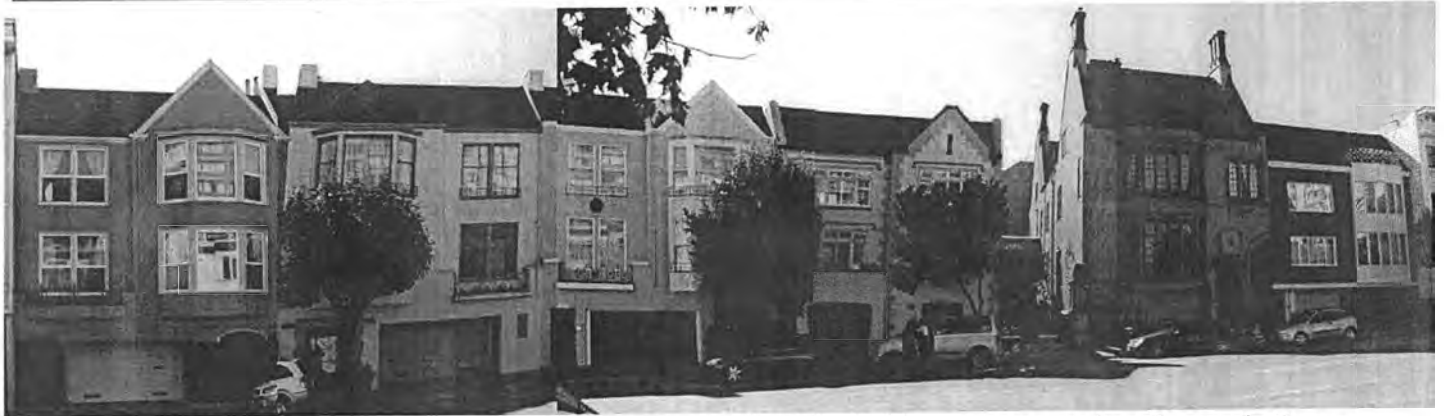
South side of California Street showing the Tobin house and all of the buildings constructed on former de Young property to the east and west. Note the side gables, stucco cladding, bay windows, chimneys, and arched entrances. Photo by Carey & Co., October 2007.
