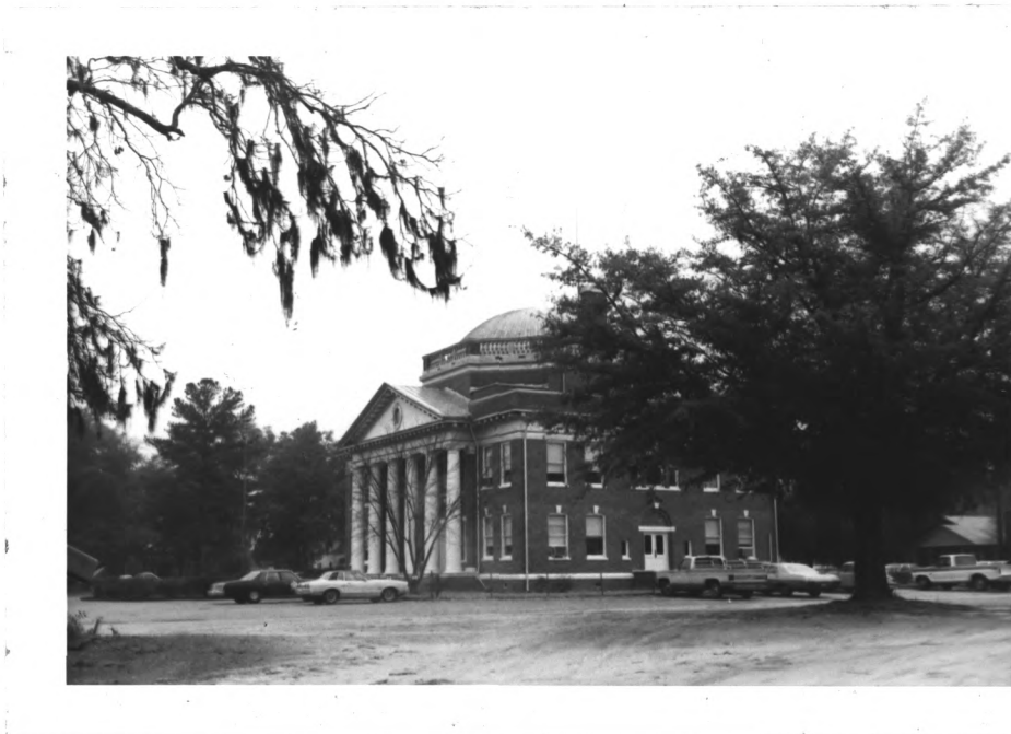
EFFINGHAM COUNTY COURTHOUSE
