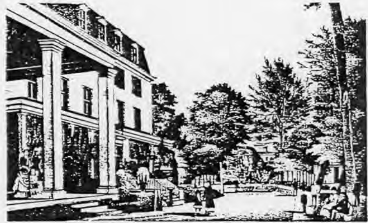
AVENUE LOOKING SOUTH
