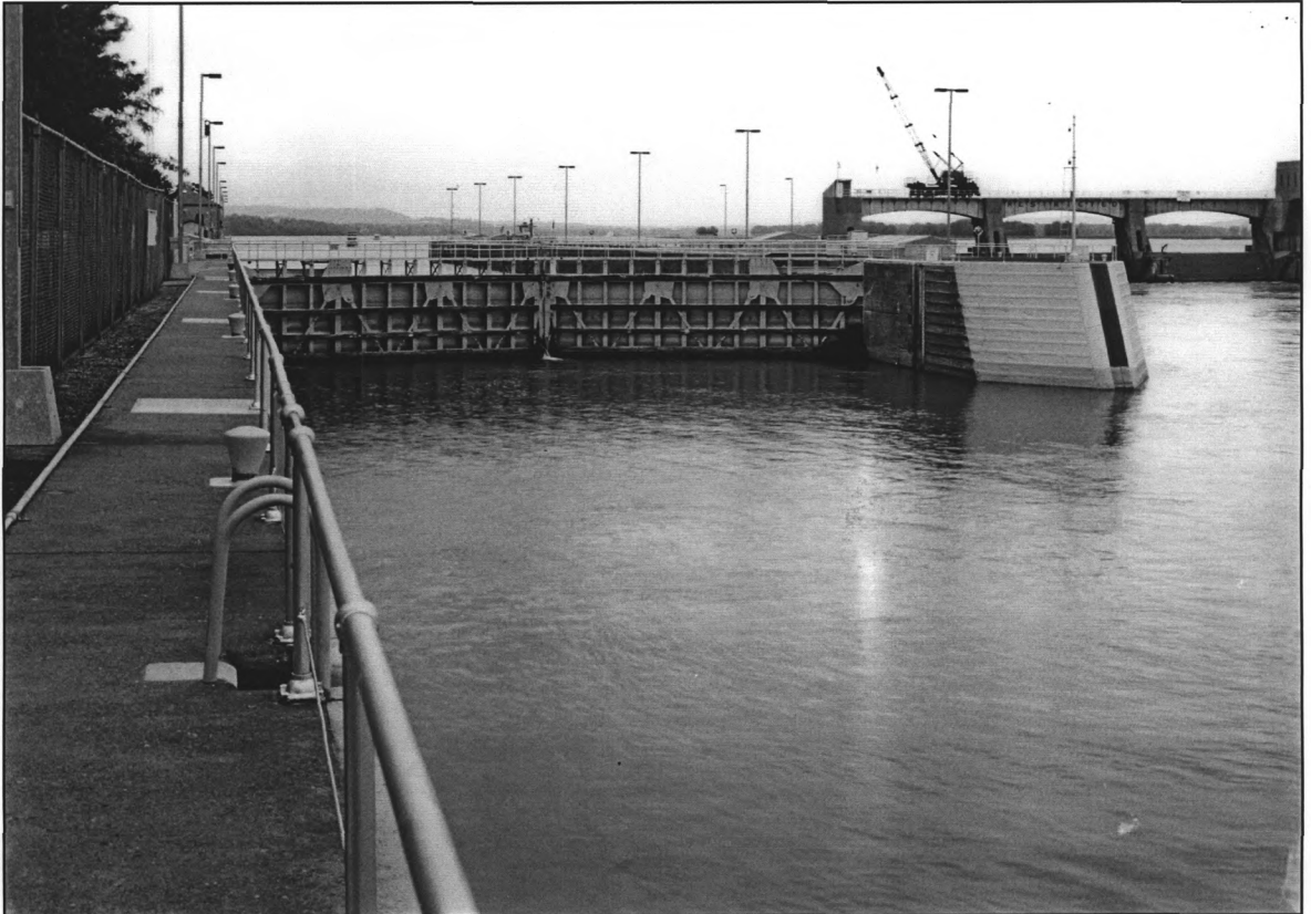
PHOTO 2. General View of Lock, Downstream Side. Photographer: Peter A. Rathbun Date of Photograph: September 1987 Location of Original Negative: IA-24-3, HAER, IOWA, 49-BEL,1- HAER Collection, Prints and Photographs Division, Library of Congress, Washington, D.C. View: From downstream guide wall of lock, looking north
