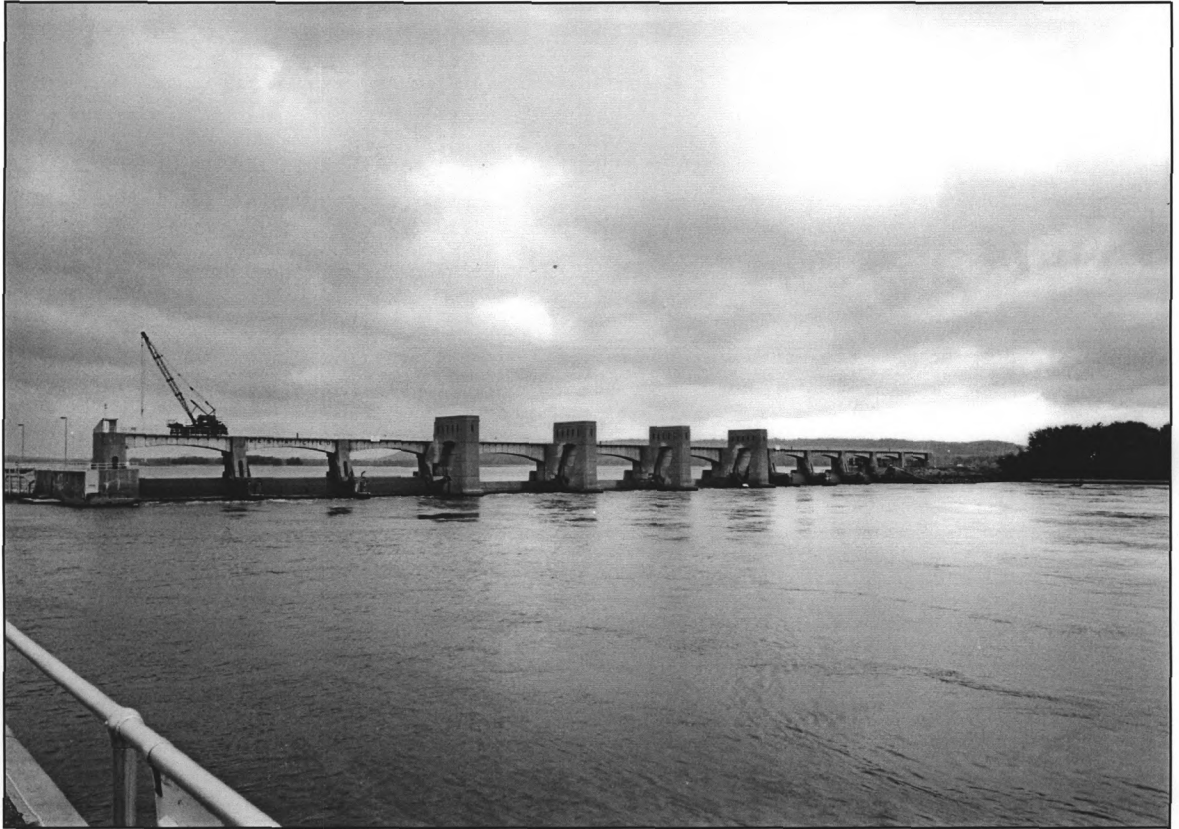
PHOTO 3. General View of Dam, Downstream Side. Photographer: Peter A. Rathbun Date of Photograph: September 1987 Location of Original Negative: IA-24-2, HAER, IOWA, 49-BEL, 1- HAER Collection, Prints and Photographs Division, Library of Congress, Washington, D.C. View: From downstream guide wall of lock, looking northeast
