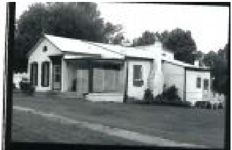
Figure 32 House at 110 Madison St., LaGrange
