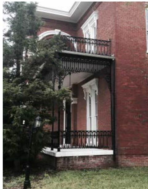
Figure 11. South Porch Balcony w/ Iron Railing
