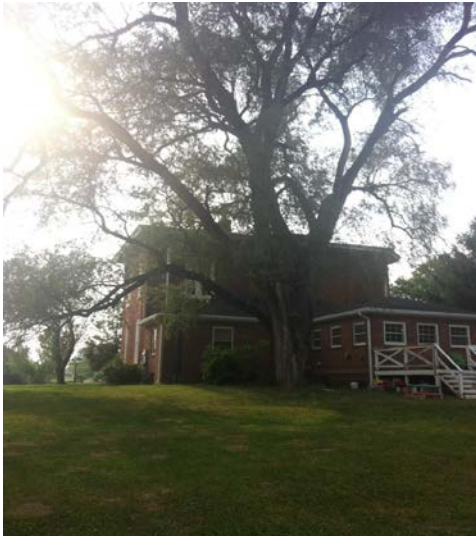
Figure 12. East (rear) side
