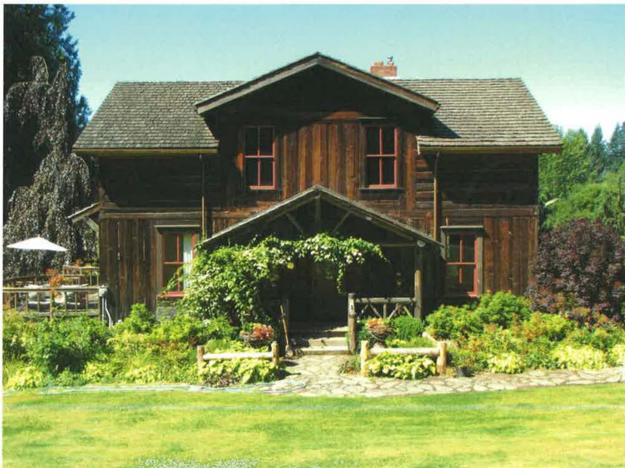
Image # 0001: Main Façade (east elevation)
