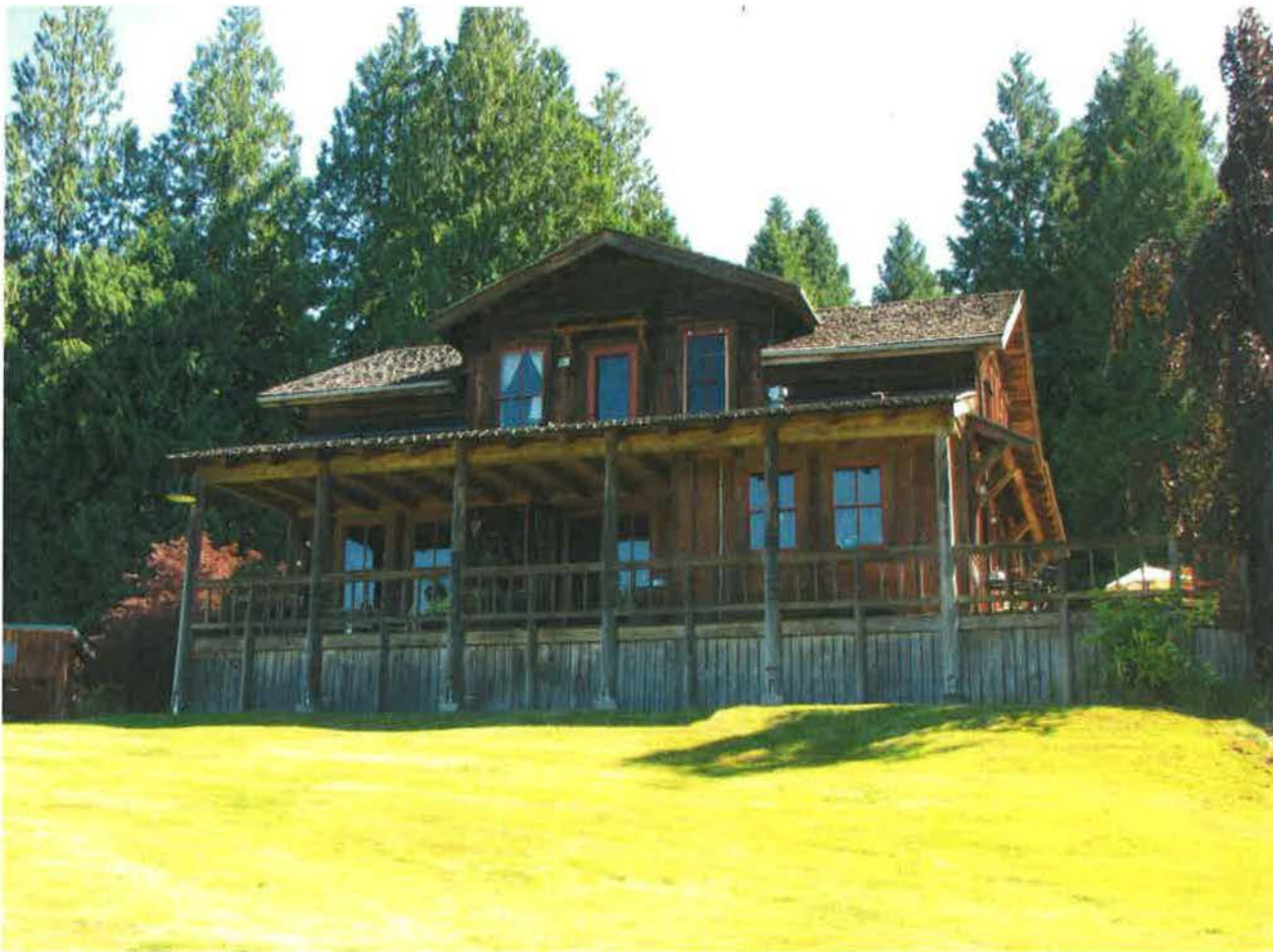
Image #0004: Rear façade (west elevation)
