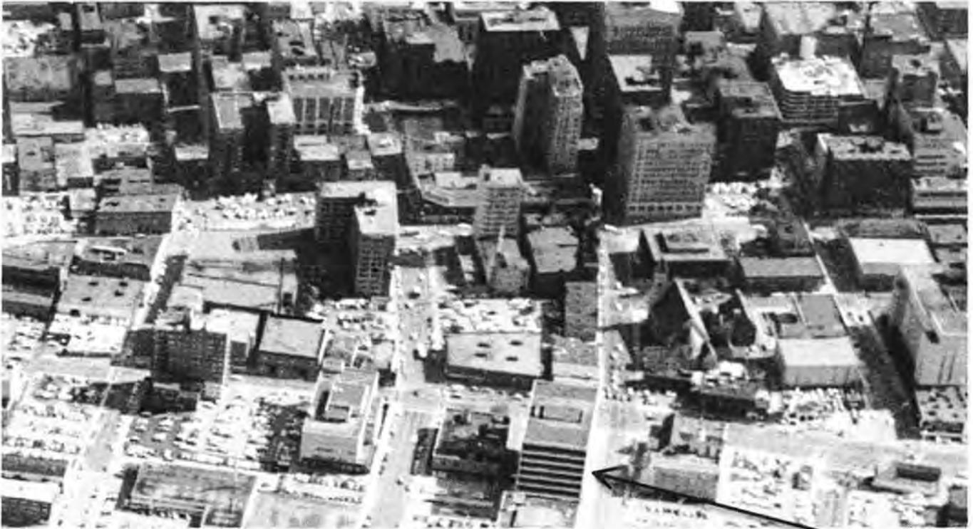
Figure 13. Historic downtown aerial photograph, circa 1965
