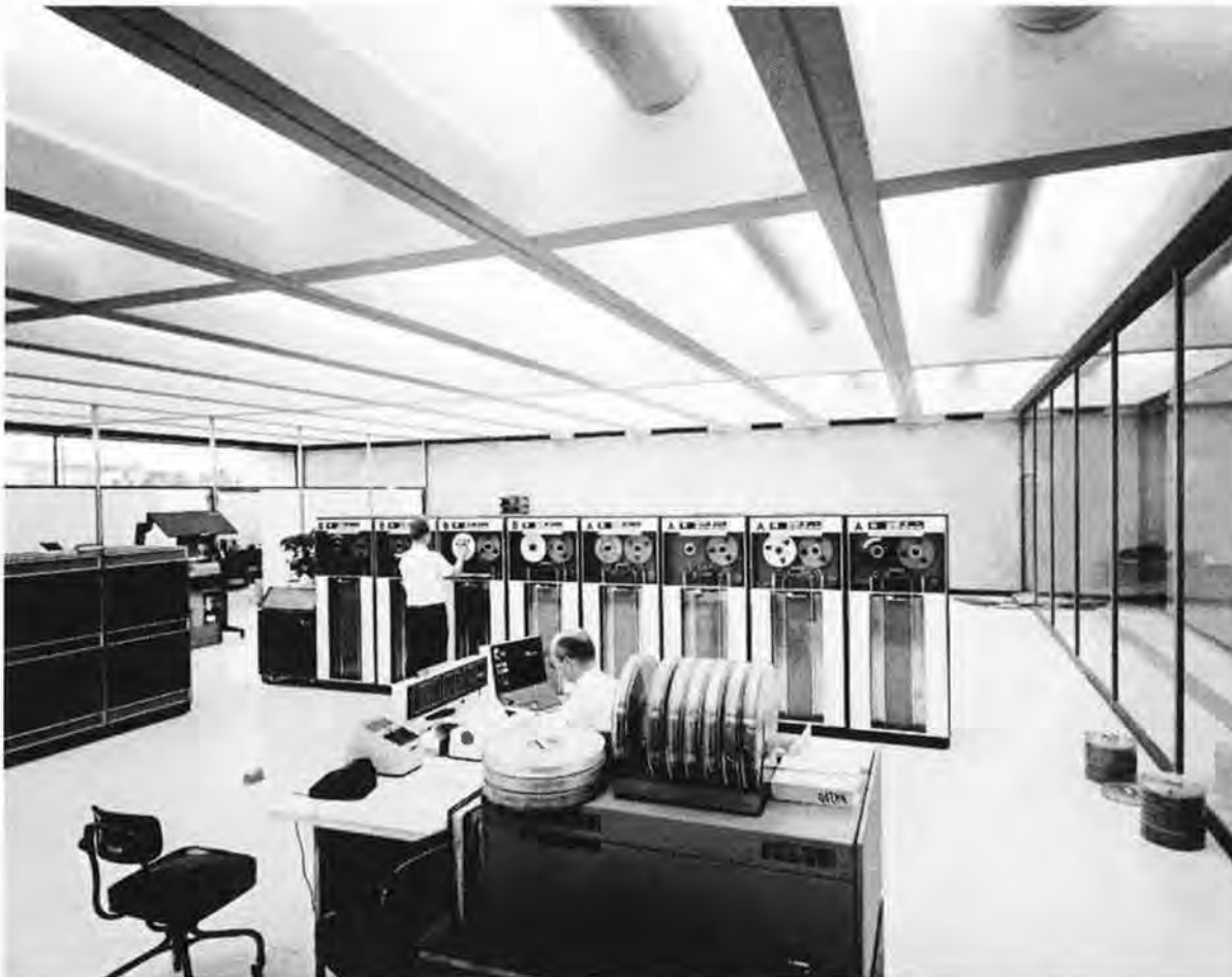
Figure 17. Historic American Republic interior photograph, computer room, circa 1965
