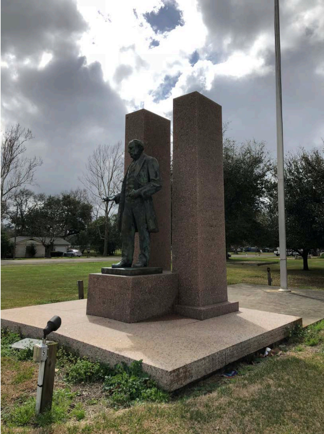
Photo 11: Northeast oblique—camera facing southwest, February 14, 2018.
