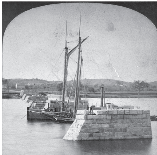
Figure 4.27 Erecting piers in the mid-nineteenth century for a multi-span bridge across the Merrimack River in Haverhill, Massachusetts. Half of a stereograph courtesy of a private collection.
