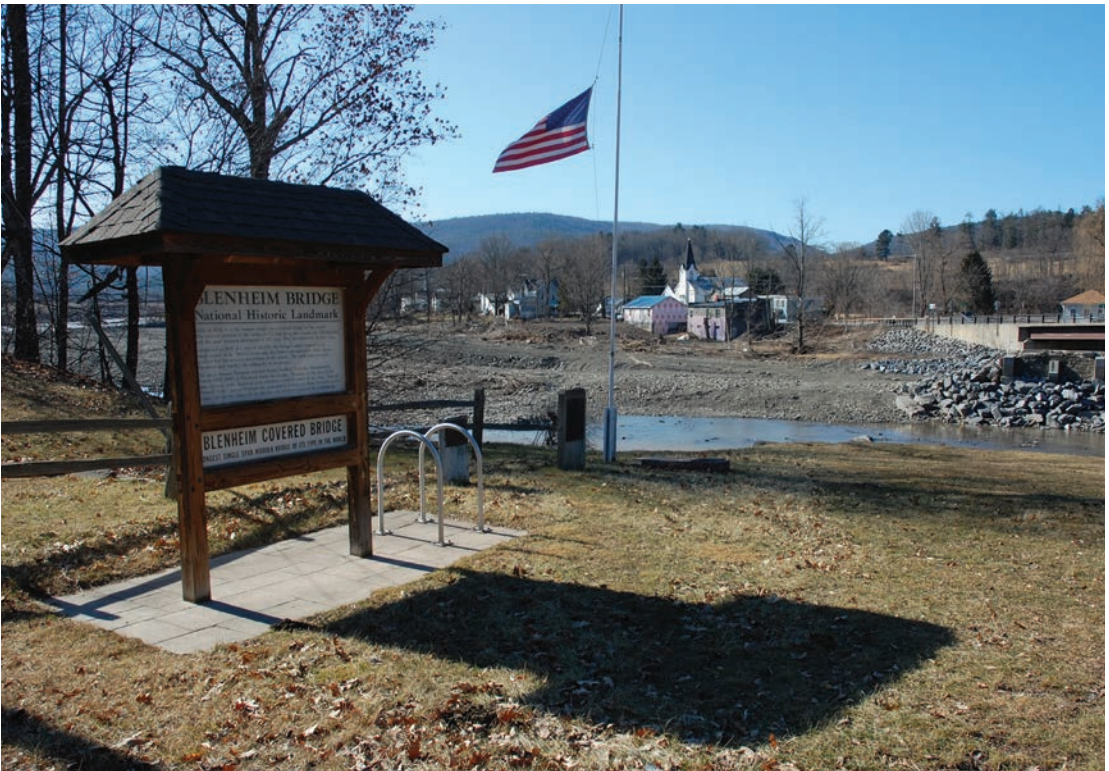
Figure 2.2 Hurricane Irene washed away Blenheim Bridge (1855), a National Historic Landmark, in September 2011. At 210 feet, the bridge had one of the longest clear spans of any surviving covered bridge and was a rare surviving double-barrel Long truss. Top: 2.2a) Before, HAER NY-331-3, Jet Lowe, photographer, 2004. Above: 2.2b) After, Matthew Kierstead, photographer, 2012.
