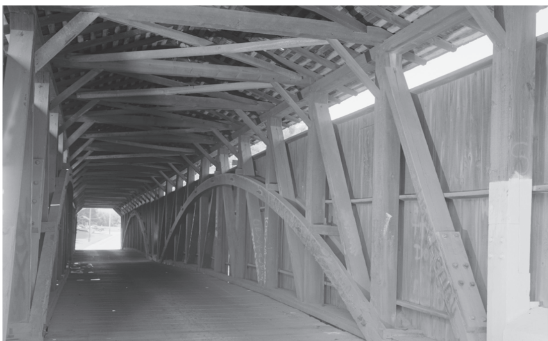
Figure 0.13 Pine Grove Bridge (1884) between Chester and Lancaster Counties, Pennsylvania, is one of eleven bridges by Elias McMellen that still stand. Although it has been rehabilitated, it still exhibits some of the finest examples of Burr-arch truss framing. HAER PA-586-7, Jet Lowe, photographer, 2002.
