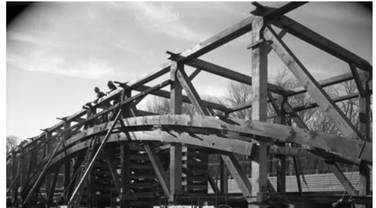
Figure 2.1 Figure 2.1 Gilpin's Falls Covered Bridge (1860) in Cecil County, Maryland, was in danger of collapse due to decaying members. An award of $1,040,000 from the NHCBP program funded a sensitive rehabilitation project in 2009–2010. Left: 2.1a) The deteriorating bridge awaiting repair. Carol M. Highsmith Archive, Library of Congress, Prints and Photographs Division, Washington, D.C., between 1980-2006. Right: 2.1b) Stabilizing the truss during Tim Andrews' rehabilitation. HAER MD-174-4, David Ames, photographer, 2009.
