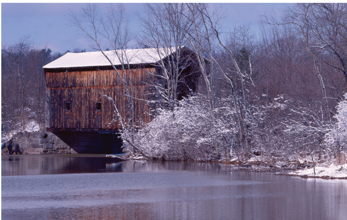
Figure 0.29 Built by the Rutland Railroad in 1897, the 94-foot Howe truss Shoreham Railroad Bridge is now a feature on a picturesque recreational trail in Addison County, Vermont. HAER VT-32-9 (CT), Jet Lowe, photographer, 2003.
