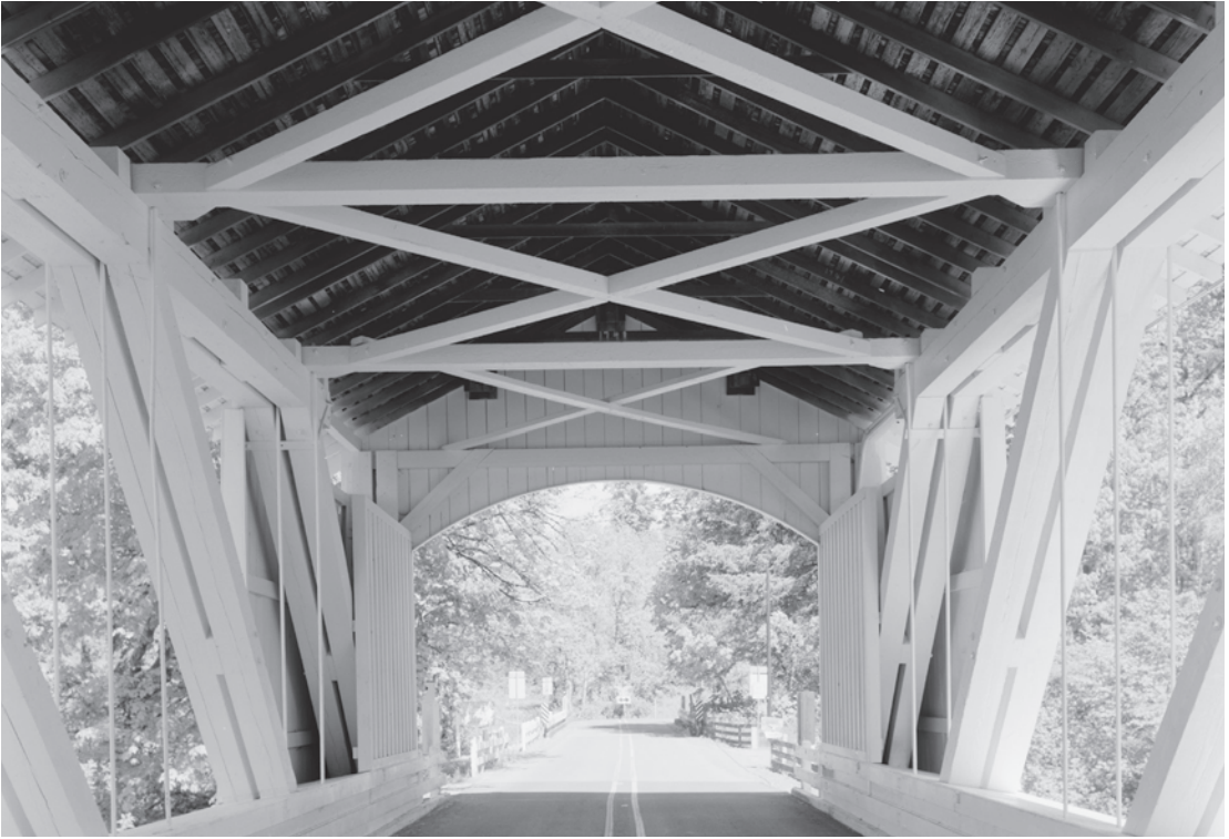
Figure 0.32 Larwood Bridge (1941) was one of several covered bridges built by the Linn County, Oregon, Engineering Department from 1920 through the 1940s from a standard Howe plan. The open-sided housing used throughout Linn County provided increased visibility and reduced wind resistance. HAER OR-124-25, Jet Lowe, photographer, 2004.
