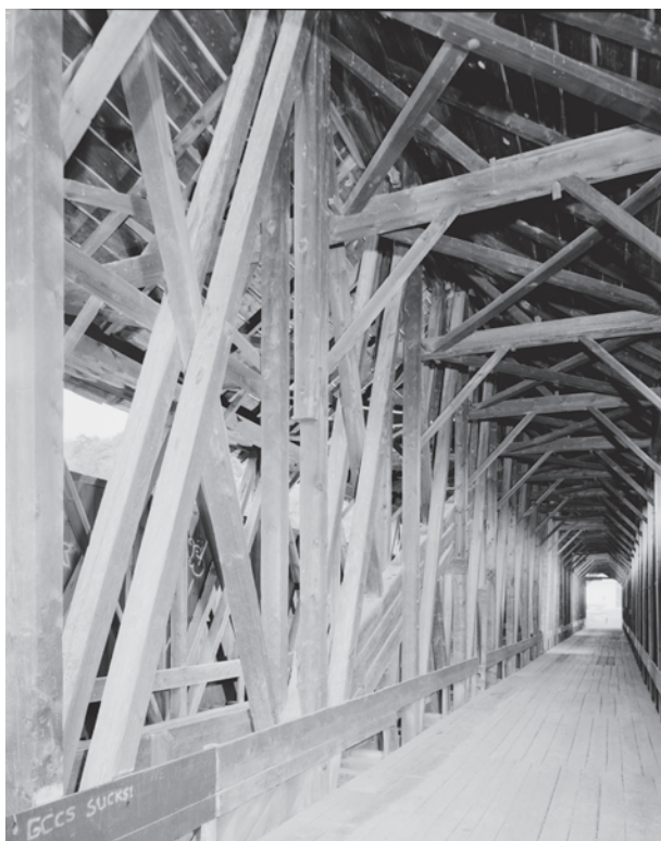
Figure 0.23 To span the Schoharie River, Nichols Powers used a double-barrel Long truss with arch for the Blenheim Bridge (1855) in Schoharie County, New York. In 1964, it was the first covered bridge to be designated as a National Historic Landmark. The bridge was destroyed by flooding in 2011. HAER NY-331-9, Jet Lowe, photographer, 2004.
