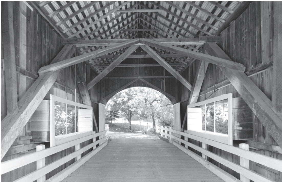
Figure 0.4 Located in Douglas County, Oregon, Neal Lane Bridge (1939), a 42-foot-long kingpost-truss bridge, features paired 1 3/4-inch-diameter iron rods as its center posts. It is the only kingpost design surviving of the many wood trusses built from standard plans by the Oregon State Highway Commission. HAER OR-126-5, Jet Lowe, photographer, 2004.
