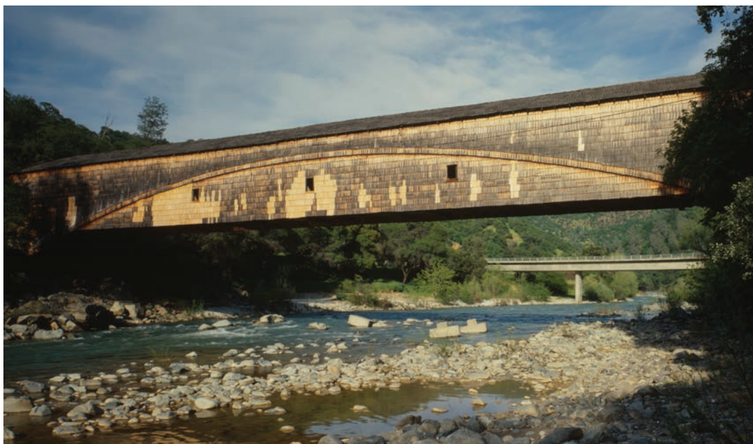
Figure 0.25 A Howe truss with arch carries the 233-foot span of the Bridgeport Bridge (1862) in Nevada County, California, built during the Comstock Lode Gold Rush by the Virginia City Turnpike Company. Massachusetts millwright William Howe introduced iron tension members into American bridge trusses. HAER CA-41-9 (CT), Jet Lowe, photographer, 1984.
