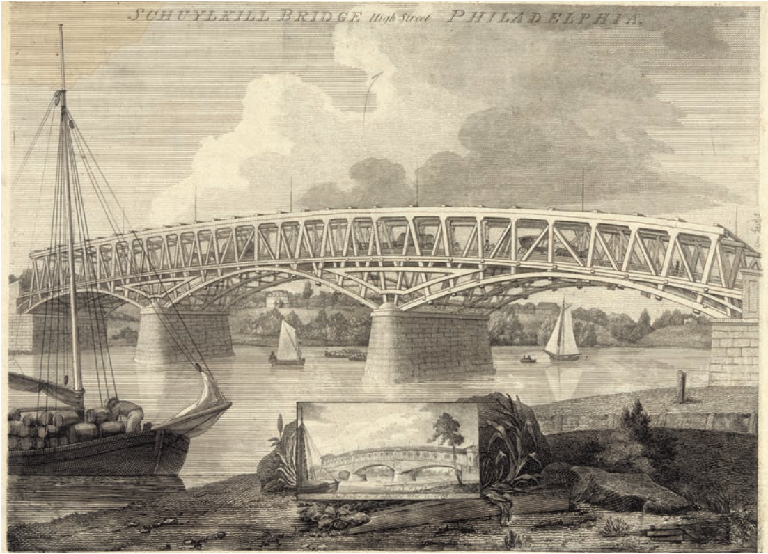
Figure 3.5 Schuylkill Bridge, High Street, Philadelphia, engraving by William Russell Birch, ca. 1804. Completed in 1805, the Schuylkill Permanent Bridge is the first documented covered bridge in the United States. It stood for forty-five years until replaced in 1850. This image depicts the bridge prior to being covered, with the completed structure shown in the inset. Courtesy of Library of Congress, Prints and Photographs Division, Washington, D.C.
