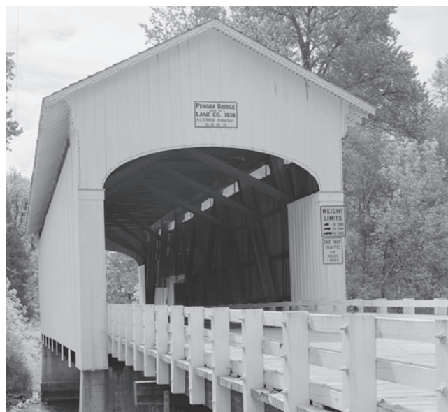
Figure 6.20 Pengra Bridge (1938) is typical of the many bridges built in the 1930s in Lane County, Oregon, under the supervision of A. C. Striker. HAER OR-119-4, Jet Lowe, photographer, 2004.
