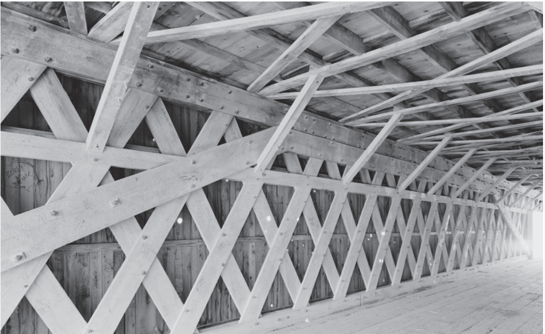
Figure 0.17 One of the bridges of Madison County, the Roseman Bridge (1883) is a Town lattice truss bridge with auxiliary queenpost trusses. HAER IA-95-6, Jet Lowe, photographer, 2004.
