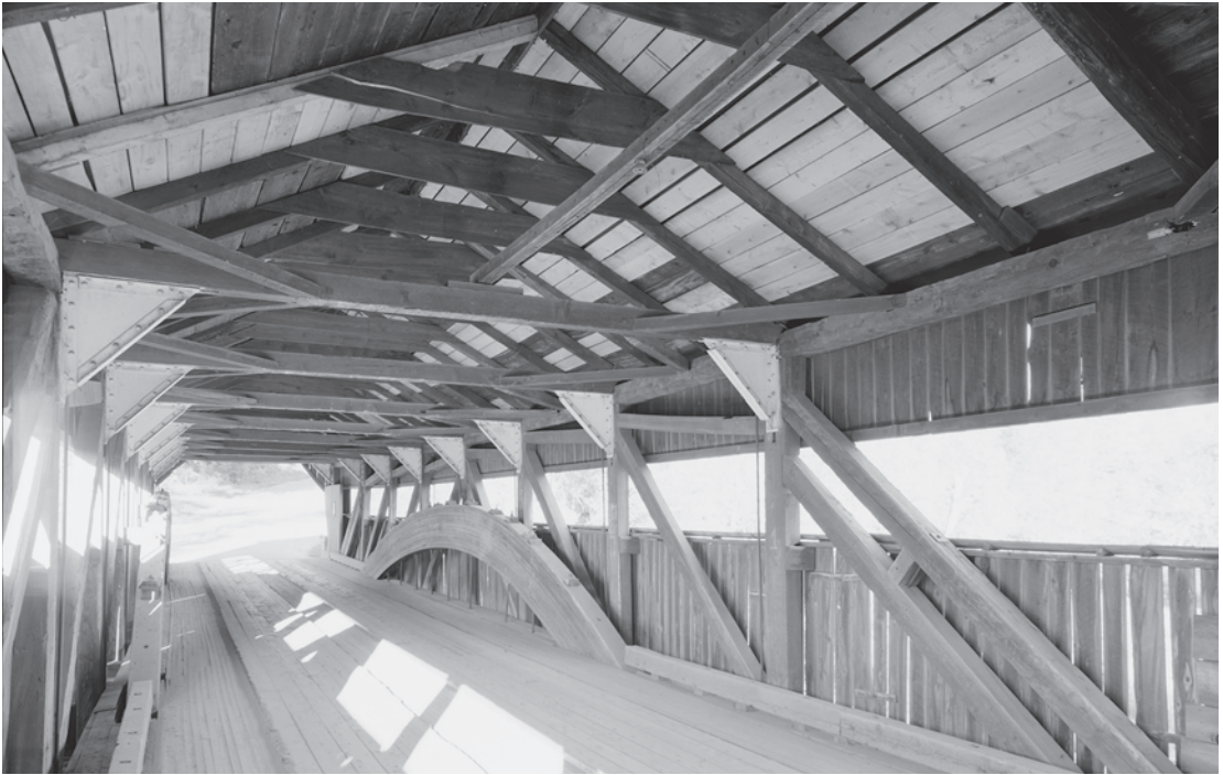
Figure 0.6 A variant of the multiple kingpost with later modifications, Taftsville Bridge (1836) displays aspects of an early craftsman tradition such as the multiple braces at the end of the trusses as seen in the foreground. HAER documented the Windsor County, Vermont, bridge prior to its rehabilitation after Hurricane Irene. HAER VT-30-8, Jet Lowe, photographer, 2003.
