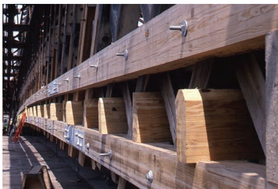
Figure 7.8 The introduction of glulam lower chords and floor beams on the Cornish-Windsor Bridge, although opposed by many preservationists, helped achieve the positive camber required to keep the bridge in use. James Garvin, photographer, December 1988 and June 1989.
