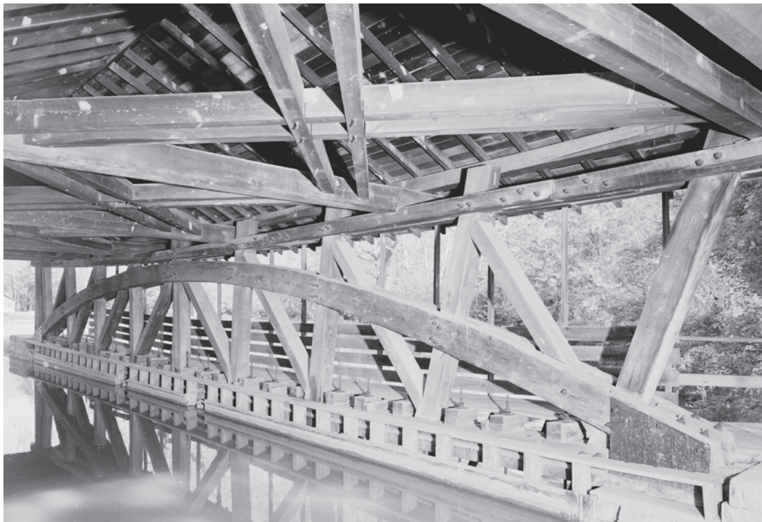
Figure 0.10 The Burr-arch truss on the Duck Creek Aqueduct (1846) in Franklin County, Indiana, features flared posts and is the sole remaining covered wood aqueduct in the country. It was designated a National Historic Landmark in 2014. HAER IN-108-2, James Rosenthal, photographer, 2004.
