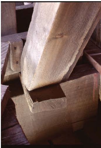
Figure 5.23 Left: 5.23a) Detail view of one of the wedges hammered into the base of each counterbrace on the Eldean Bridge. William G. Keener, photographer, 1998. Courtesy of Ohio History Connection. Right: 5.23b) Interior elevation of Eldean Bridge’s Long truss. The wedge connection details are out of view, just below the deck. HAER OH-122-14, Jet Lowe, photographer, 2002.
