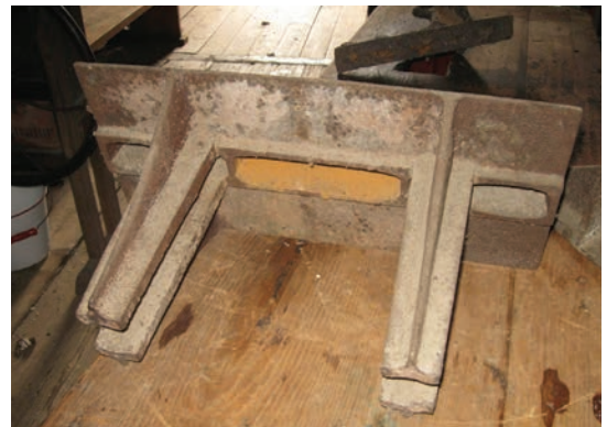
Figure 5.32 Casting with sleeves that transferred rod tension forces directly into the casting without causing bearing stresses in the chords and possibly crushing them. Found on the Rexleigh Bridge, a Howe truss dating to 1874 in Washington County, New York. Dario Gasparini, photographer, 2011.
