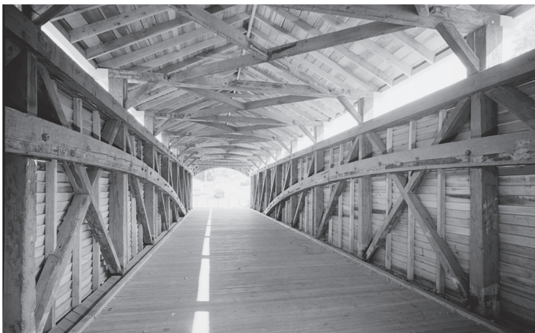
Figure 0.11 Barrackville Bridge (1853) in Marion County, West Virginia, is a 131-foot span Burr-arch truss bridge. HAER documented the bridge following rehabilitation by Emory Kemp in 1999. It is one of three extant bridges completed by West Virginia bridge builder Lemuel Chenoweth. HAER WV-8-23, Jet Lowe, photographer, 2002.
