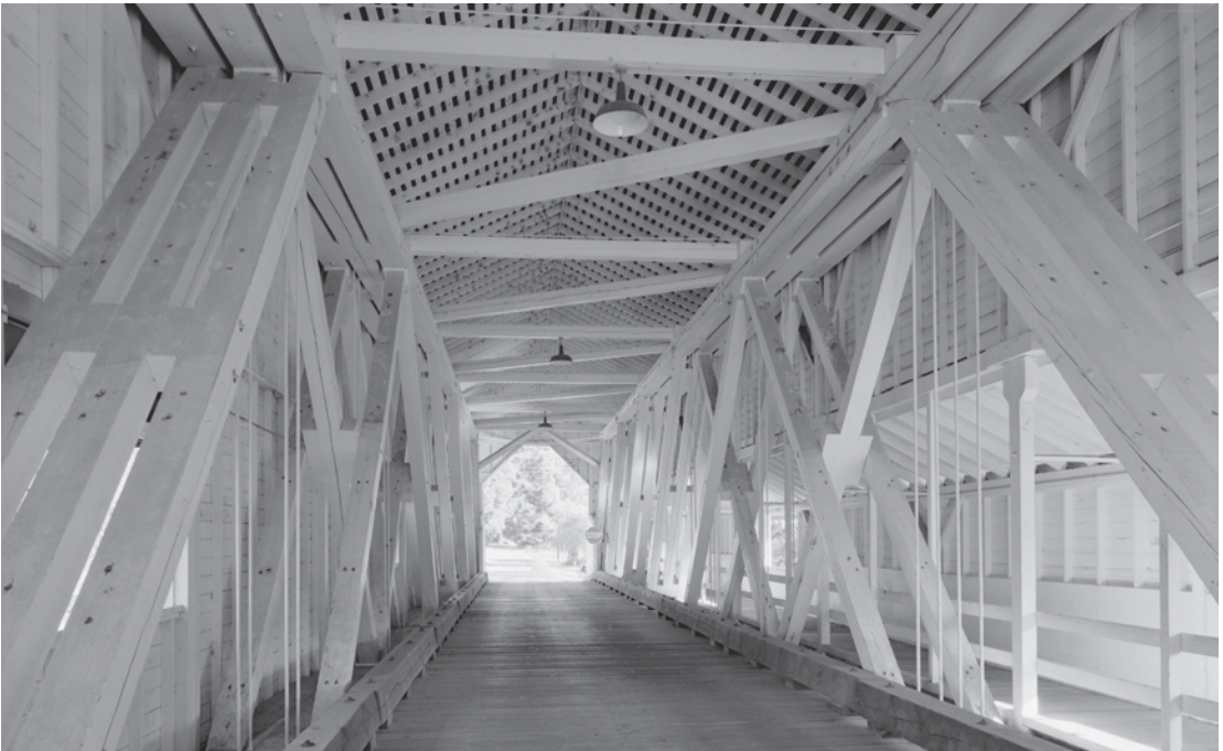
Figure 0.33 The Office Bridge (1944) in Lane County, Oregon, features a 180-foot-long Howe truss with paired braces and single counters measuring 14 inches x 16 inches. The massive bridge carried logging truck traffic for the Westfir lumber mill until the plant closed in 1977. HAER OR-125-6, Jet Lowe, photographer, 2004.
