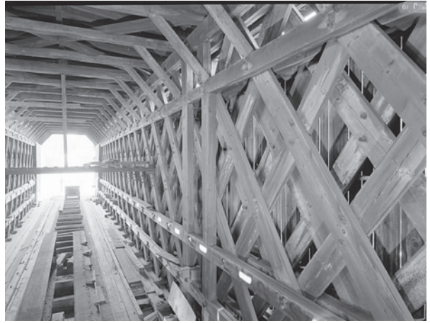
Figure 7.9 The two-span, double-web Town lattice truss Contoocook Railroad Bridge was originally located on the Boston and Maine Railroad. It is one of only eight surviving covered railroad bridges in the United States and remains standing thanks to the multi-year efforts of preservationists working in partnership with the state from 1989 to 2007. HAER NH-38-5, Jet Lowe, photographer, 2003.
