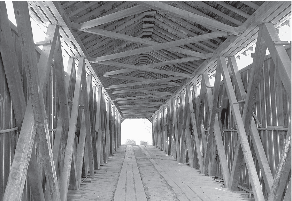
Figure 6.18 The Smith Bridge Company of Toledo, Ohio, shipped the parts for a patented Smith truss to local communities for other contractors to erect. Local contractor W. T. Washer built the Wheeling Bridge in Gibson County, Indiana, in 1877. Joseph D. Conwill, photographer, 2003.
