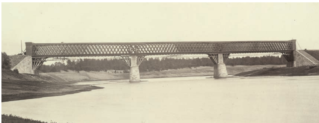
Figure 5.33 Examples of George Washington Whistler's Howe truss bridges on the St. Petersburg–Moscow (Nikolaev) Railway, ca. 1860. Above top: 5.33a) is the nine-span, 1,600-foot Msta Bridge; Above: 5.33b) is the three-span Tverca River Bridge. Courtesy of DeGolyer Library, Southern Methodist University, Dallas, Texas, Views of the Nikolaev Railway.
