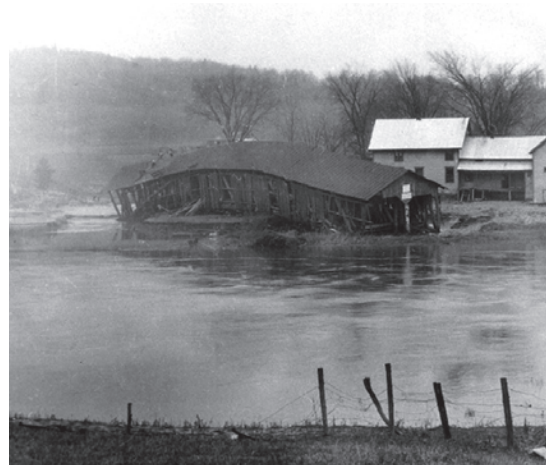
Figure 7.3 Historically, flooding frequently resulted in covered bridges being washed downstream. The North Enosburg Covered Bridge spanning the Missisquoi River in Franklin County, Vermont, floated downstream during a 1927 flood. Courtesy of Richard Sanders Allen Collection, National Society for the Preservation of Covered Bridges.
