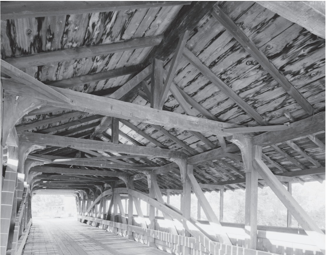
Figure 0.9 The Village Bridge (1833) in Washington County, Vermont, is a Burr-arch truss bridge noted for its hand-tooled knee braces added by Milton Graton during repairs in the early 1970s. The hand-tooled knee braces replaced steel sway braces added during the mid-twentieth century. HAER VT-34-4, Jet Lowe, photographer, 2004.
