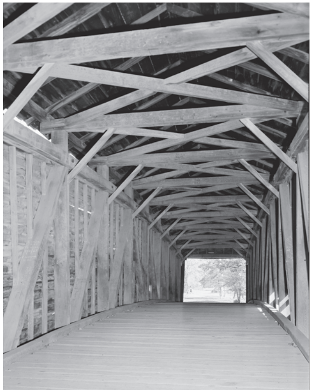
Figure 0.6 A variant of the multiple kingpost with later modifications, Taftsville Bridge (1836) displays aspects of an early craftsman tradition such as the multiple braces at the end of the trusses as seen in the foreground. HAER documented the Windsor County, Vermont, bridge prior to its rehabilitation after Hurricane Irene. HAER VT-30-8, Jet Lowe, photographer, 2003.
