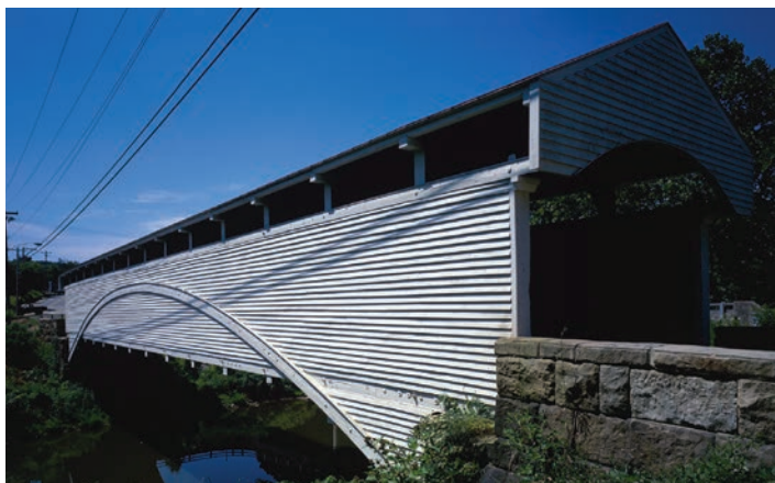
Figure 6.10 Barrackville Covered Bridge (1853), a Burr-arch truss built by Lemuel Chenoweth on the Fairmont and Wheeling Turnpike in Marion County, West Virginia. HAER WV-8-25, Jet Lowe, photographer, 2002.
