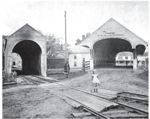
Figure 3.7 This ca. 1880 photograph, taken in Contoocook Village, Hopkinton, New Hampshire, shows the 1849 Concord and Claremont Railroad Bridge on the left; another covered bridge, which still survives, replaced that bridge in 1889. The town of Hopkinton built the roadway bridge on the right in 1853; it was replaced in 1936 with a stone-faced concrete bridge. Courtesy of Hopkinton Historical Society, Hopkinton, New Hampshire.
