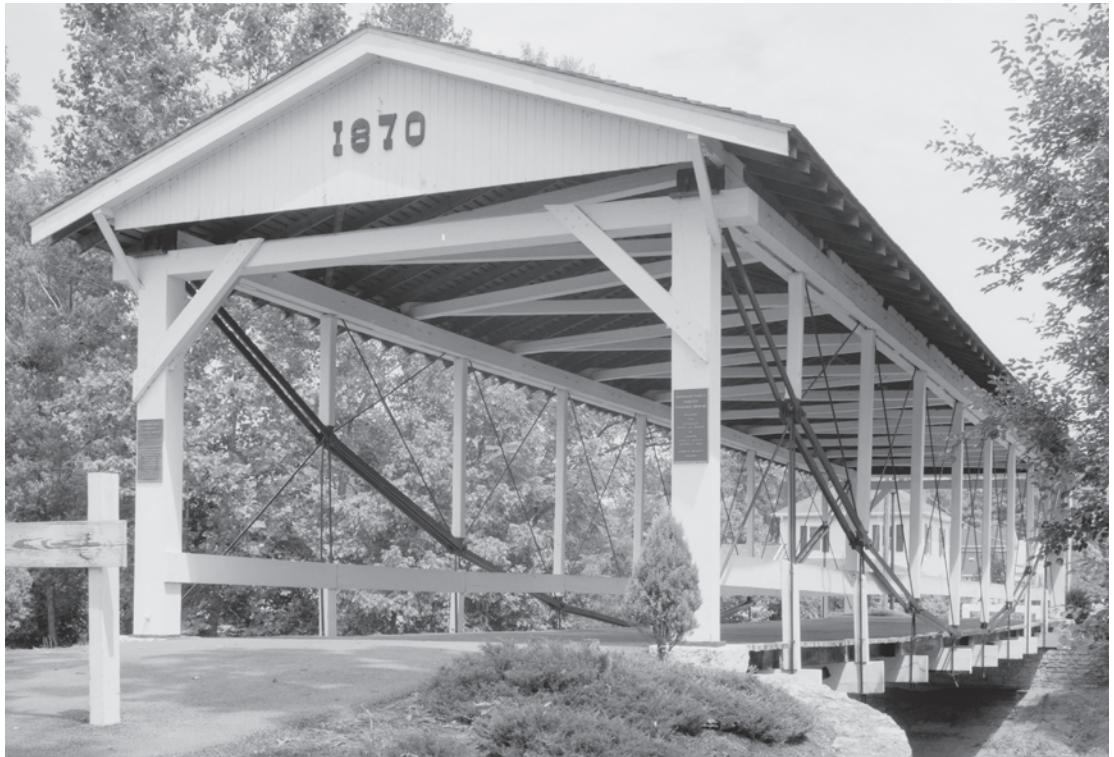
Figure 0.44 The inverted Bowstring truss on the Germantown Bridge (1865) in Montgomery County, Ohio, is a combination wood and iron rigid suspension truss, in which all compression members are wood and the inverted, arched iron suspension chain is in tension. A rare surviving example of the transitional bridge building period from wood to iron, it is an example of the early work of David H. Morrison, founder of the Columbia Bridge Works of Dayton, Ohio. HAER OH-87-2, Joseph Elliott, photographer, 1992.
