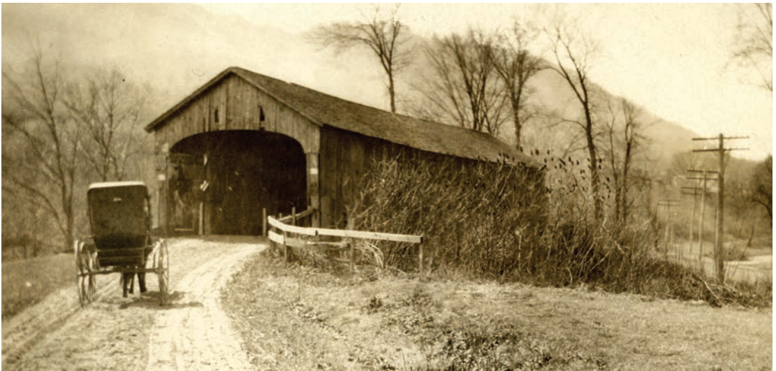
Figure 3.1 Charles Whitney wrote in the introduction to Rosalie Wells's 1931 Covered Bridges in America , "The present generation does not. . . realize the important role which the timber bridge played in the early development of the American continent. But for the abundance of timber and the ingenuity of the American bridge builder, the construction of bridges across the many rivers would have been impossible when bridges were so much needed to carry the highways and railways into undeveloped country." Fort River Bridge (1840) in Hampshire County, Massachusetts, carried vehicular traffic until it was lost to arson in 1962. The structure was captured around the turn of the twentieth century by renowned local author and photographer Clifton Johnson. Courtesy of Jones Library, Inc., Amherst, Massachusetts.
