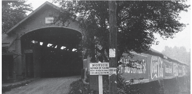
Figure 3.21 In the late nineteenth and early twentieth centuries, advertisements were sometimes painted on the exteriors of covered bridges in prominent locations. As a consequence, the Portland-Columbia Bridge (1869) spanning the Delaware River between Pennsylvania and New Jersey was known as the “Coca-Cola Bridge” in the early twentieth century. Hurricane-related floods in 1955 destroyed the bridge. Edward Hungerford, photographer, 1916. Courtesy of Thomas E. Walczak Collection.
