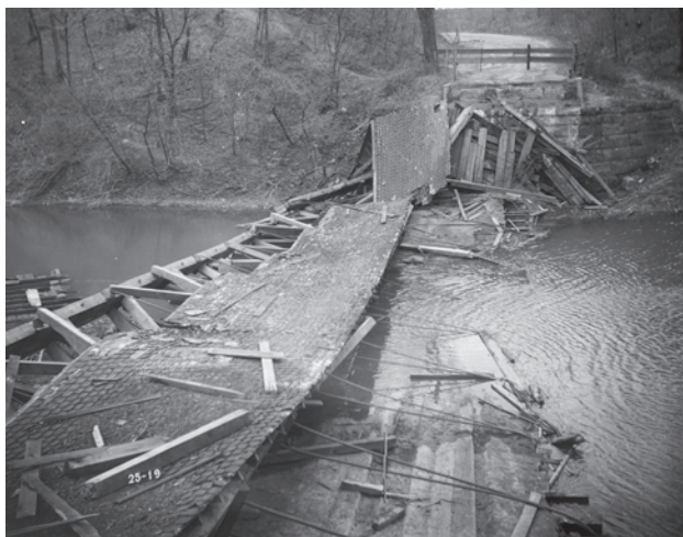
Figure 7.6 HABS architects measured the Howe truss bridge spanning the Salt Fork River in Champaign County, Illinois, only days before its collapse. HABS photographer Chauncey Buck captured the remains of the bridge on April 13, 1934. “It makes my hair stand on end when I think of how we galloped across that bridge, stamping vigorously to keep warm,” said team member Ralph Varney. “It must have come very close to being our ‘Bridge of San Luis Rey.’” HABS IL-25-19, Chauncey Buck, photographer, 1934.
