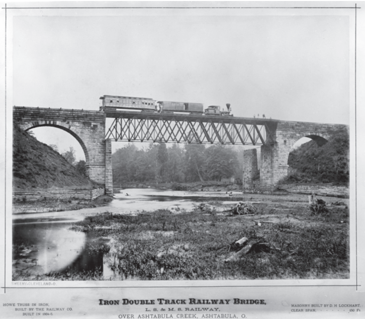
Figure 4.13 Amasa Stone was a highly accomplished railroad contractor of traditional combination wood and iron Howe trusses. After building several Howe trusses with cast-iron webs, he experimented with a Howe design that substituted wrought-iron I-beams for the wooden diagonals. Completed in 1865, the Ashtabula Bridge collapsed during a blizzard in December 1876, resulting in one of the nation’s deadliest bridge disasters. A broken cast-iron bearing block was identified as the immediate cause of the collapse. Thomas T. Sweeny, photographer, 1865. Courtesy of Ohio History Connection.
