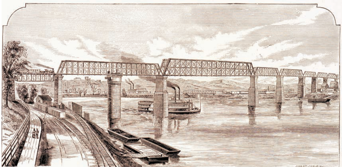
CINCINNATI SOUTHERN RAILROAD BRIDGE ACROSS THE OHIO RIVER.
