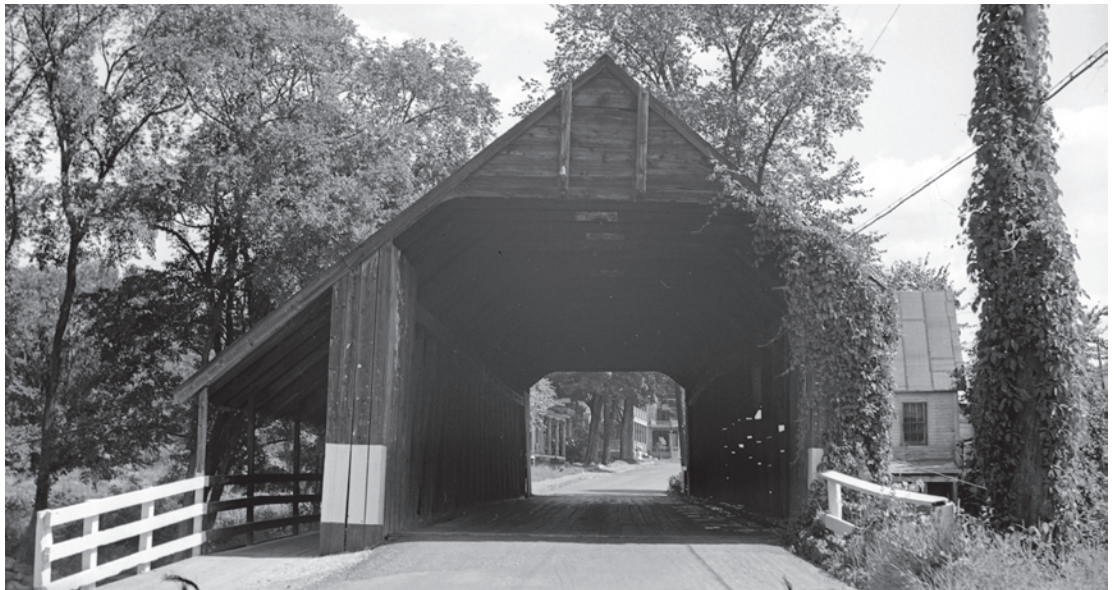
Figure 7.7 Goodhue/Tannery Bridge in Enfield, New Hampshire, was the object of an intense, multi-year preservation battle that ended with its removal. Richard Sanders Allen, photographer, August 11, 1941. Courtesy of Richard Sanders Allen Collection, National Society for the Preservation of Covered Bridges.
