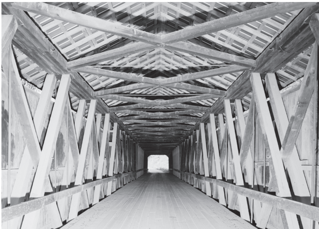
Figure 0.28 Joseph Britton's Pine Bluff Bridge (1886) is one of several Howe trusses built by Britton and his sons in Putnam County, Indiana. HAER IN-103-4, James Rosenthal, photographer, 2004.
