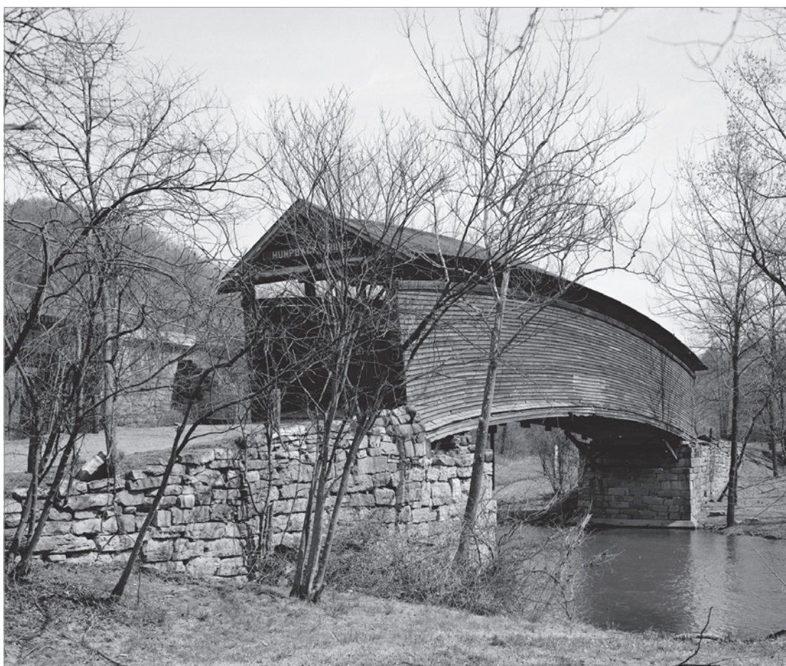
Figure 1.2 HAER documented its first covered bridge, Humpback Covered Bridge in Alleghany County, Virginia, in 1970. So named because of its marked camber, the bridge was designated a National Historic Landmark in 2012 as the best surviving example of a timber multiple-kingpost truss, making it an outstanding example of nineteenth-century bridge construction. HAER VA-1-6, Jack Boucher, photographer, 1971.
