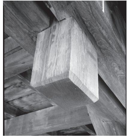
Figure 4.34 Typical detail of a double-notched post connection. Left: 4.34a) From Henry Jacoby, Structural Details, or Elements of Design in Heavy Framing (New York: J. Wiley & Sons, 1909), 135. Right: 4.34b) Detail of Leatherwood Station Bridge (1899), in Parke County, Indiana, HAER IN-40-15, Ed Sels, photographer, 1979.
