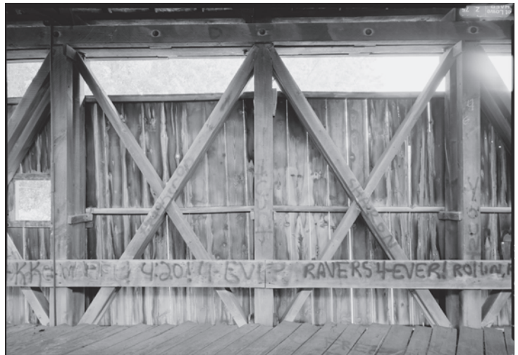
Figure 5.23 Left: 5.23a) Detail view of one of the wedges hammered into the base of each counterbrace on the Eldean Bridge. William G. Keener, photographer, 1998. Courtesy of Ohio History Connection. Right: 5.23b) Interior elevation of Eldean Bridge’s Long truss. The wedge connection details are out of view, just below the deck. HAER OH-122-14, Jet Lowe, photographer, 2002.
