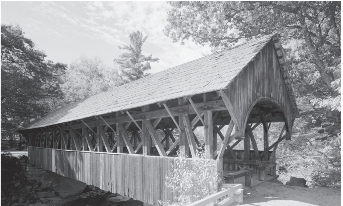
Figure 0.37 Sunday River Bridge (1872) in Oxford County, Maine, is a fine example of a Paddleford truss. Invented by bridge builder Peter Paddleford in the 1830s, the Paddleford truss dominated covered bridge construction throughout much of northern New England for more than half a century. Jet Lowe, HAER ME-69-1, photographer, 2003.
