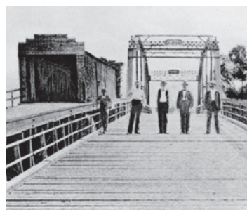
Figure 3.20 Modern spans replaced many covered bridges in the early twentieth century. After fifty years of service, the San Marcos River Bridge (1845) in Gonzales County, Texas, was replaced with a metal-truss span in 1904. Courtesy of Texas Department of Transportation.
