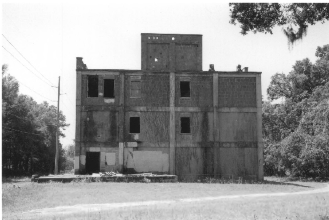
Oblique view of north elevation
