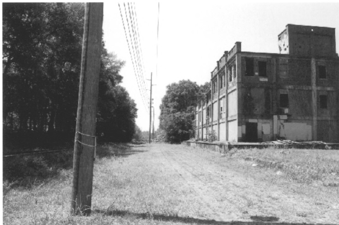
Oblique view of east elevation
