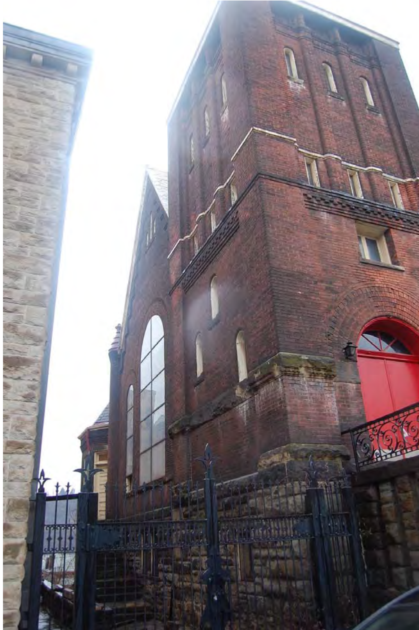
Photo 9. East side facade
