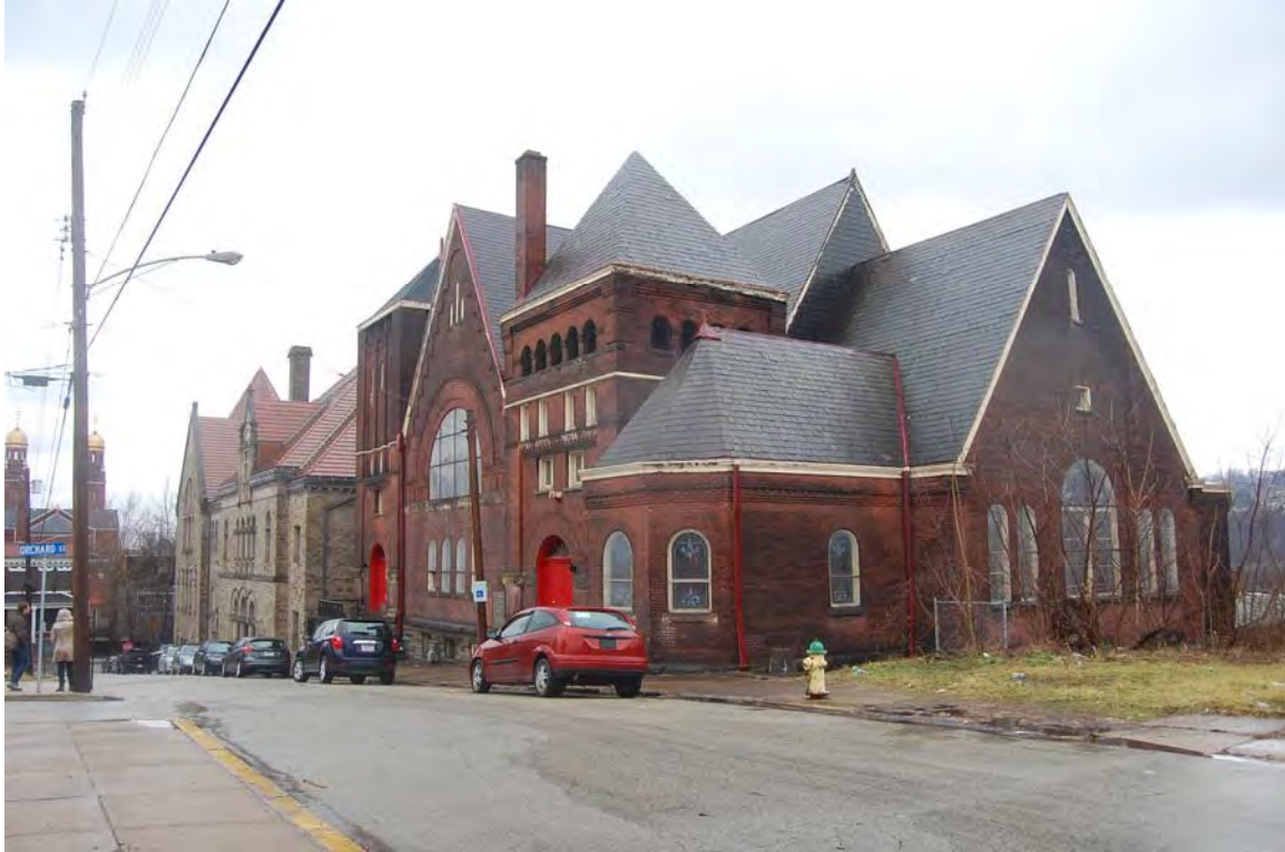
Photo 1. First United Presbyterian Church of Braddock, primary and west side facades
