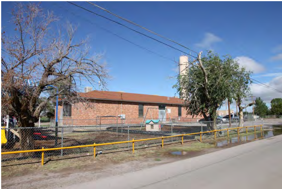
6 of 18. Main and south sides, photographer facing northwest.
