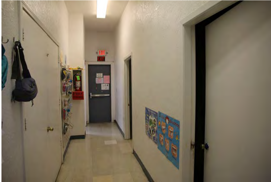
17 of 18. Interior, south corridor, photographer facing south.
