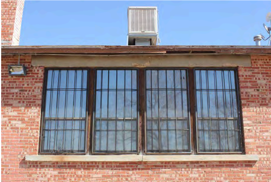
9 of 18. Bank of window on rear façade, photographer facing east.
