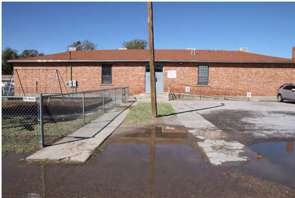
2 of 18. Main façade with historic sidewalks, photographer facing west.
