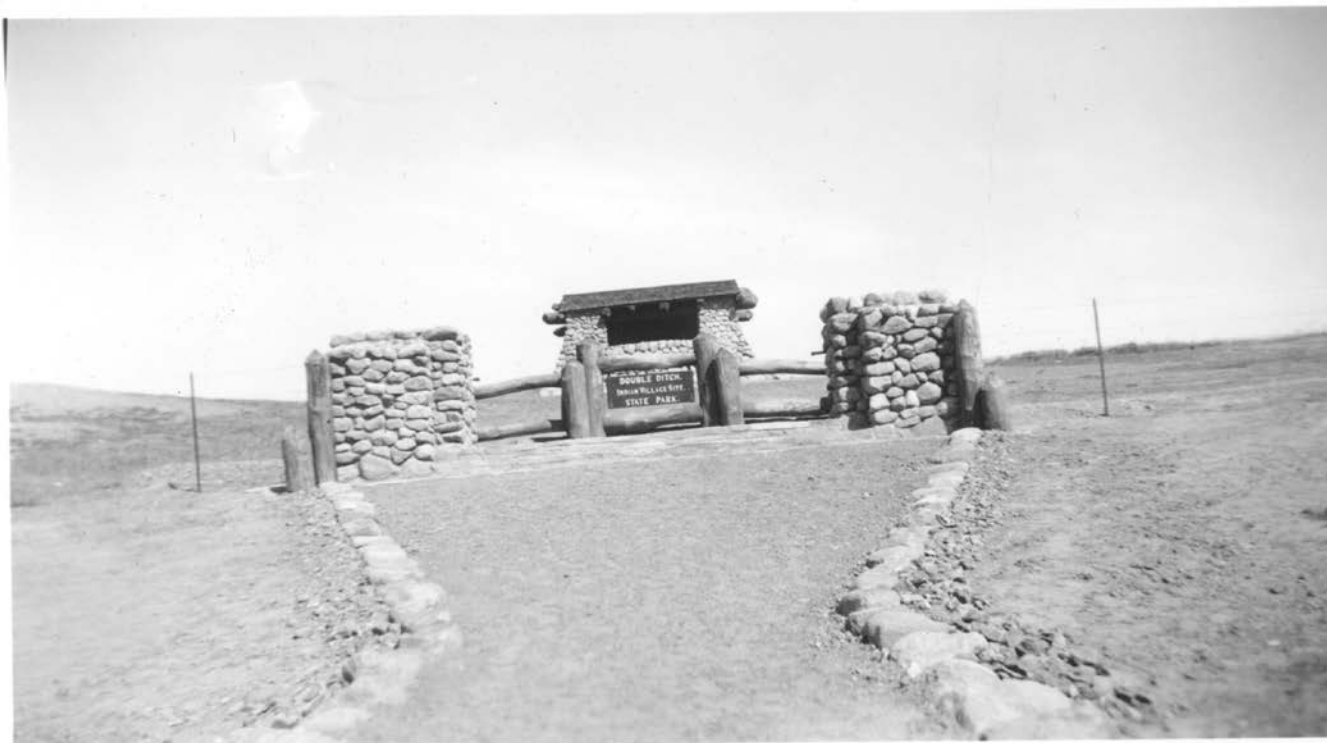
A closer view of the entrance from the west.
