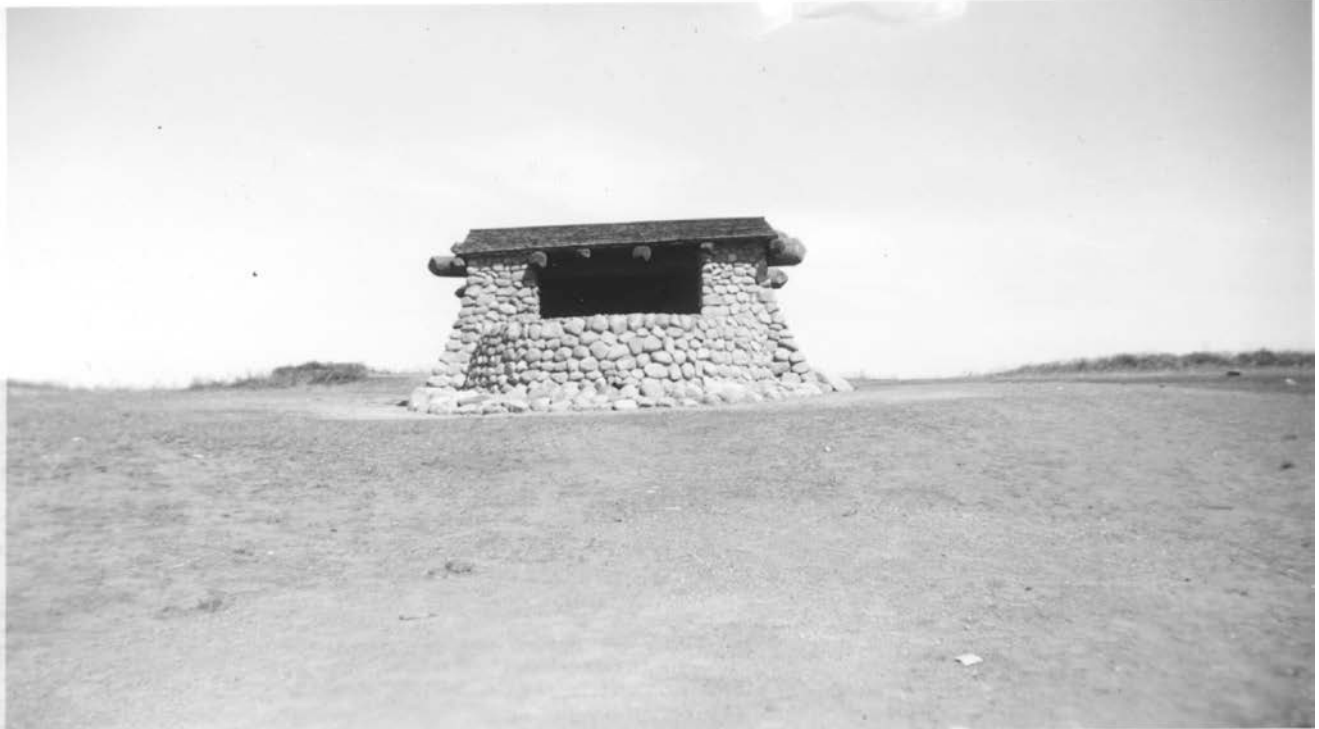
The shelter from the west.
