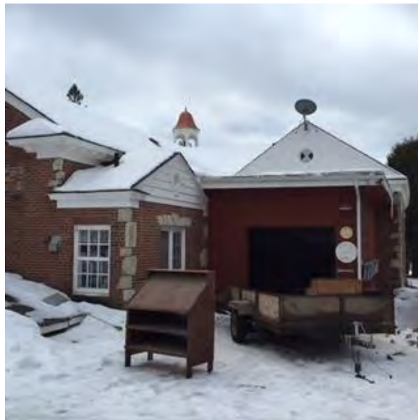
Garage addition on the northwest, 2016. Photograph by Jeff Day.
