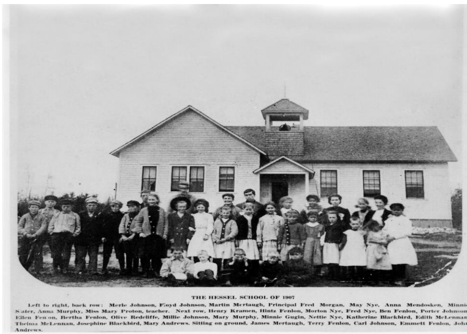
Original Hessel School in 1907. Photograph courtesy of Les Cheneaux Historical Museum.
