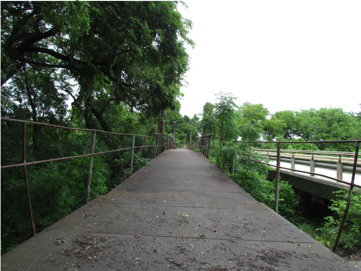
TX_Erath County_Bluff Dale Bridge_0001.tif Barrel view, looking north
