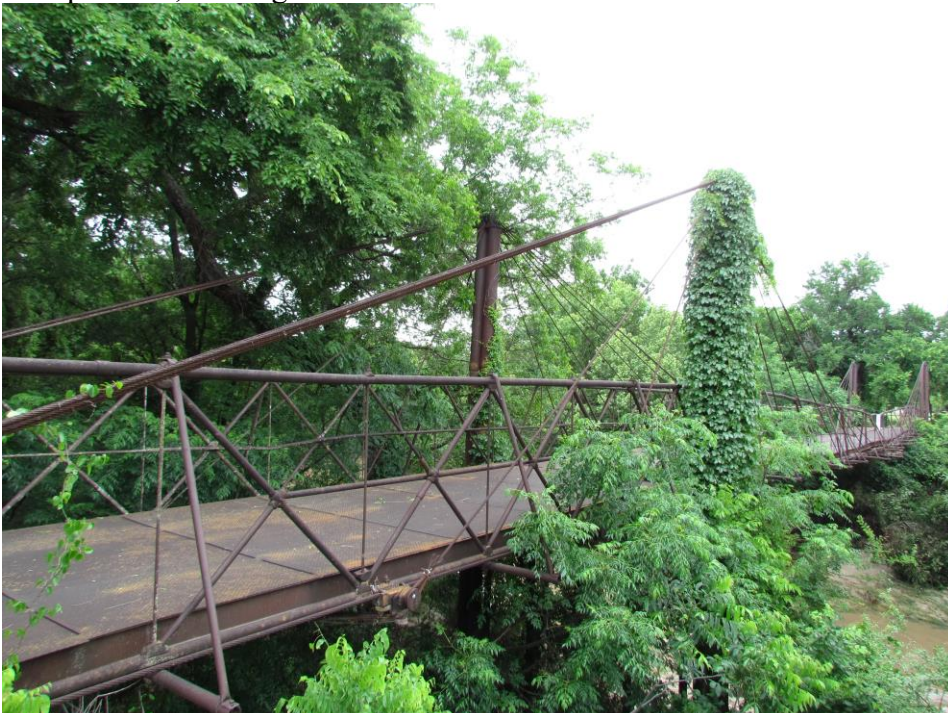
TX_Erath County_Bluff Dale Bridge_0003.tif Oblique view, looking northwest
