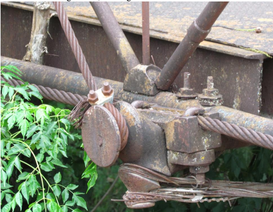
TX_Erath County_Bluff Dale Bridge_0019.tif Deck beam castings detail, looking southwest
