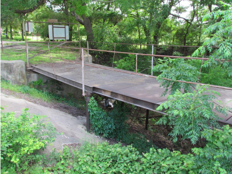
TX_Erath County_Bluff Dale Bridge_0002.tif South approach spans, looking southwest
