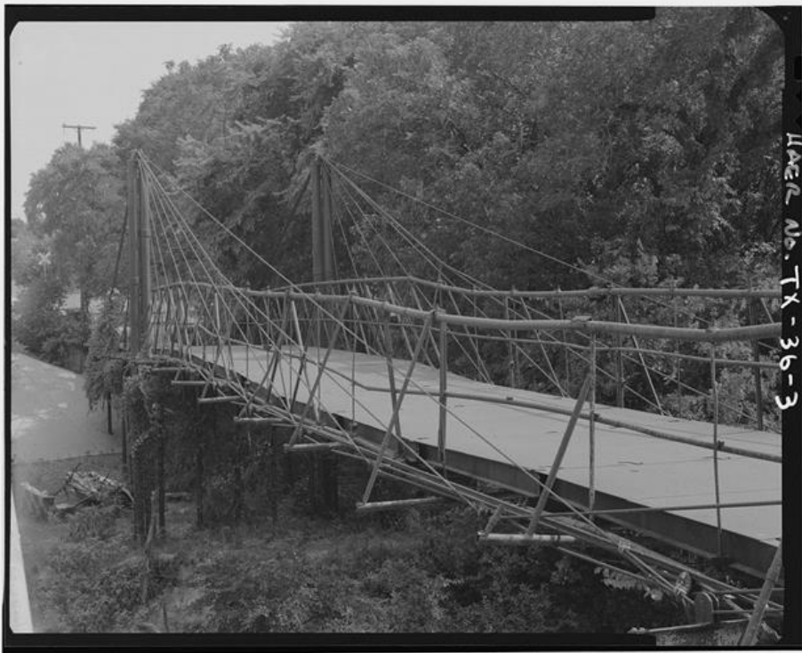
Figure 8: HAER TX-36 Photograph by Joseph E. B. Elliot (1996). 3/4 view, from northeast.
