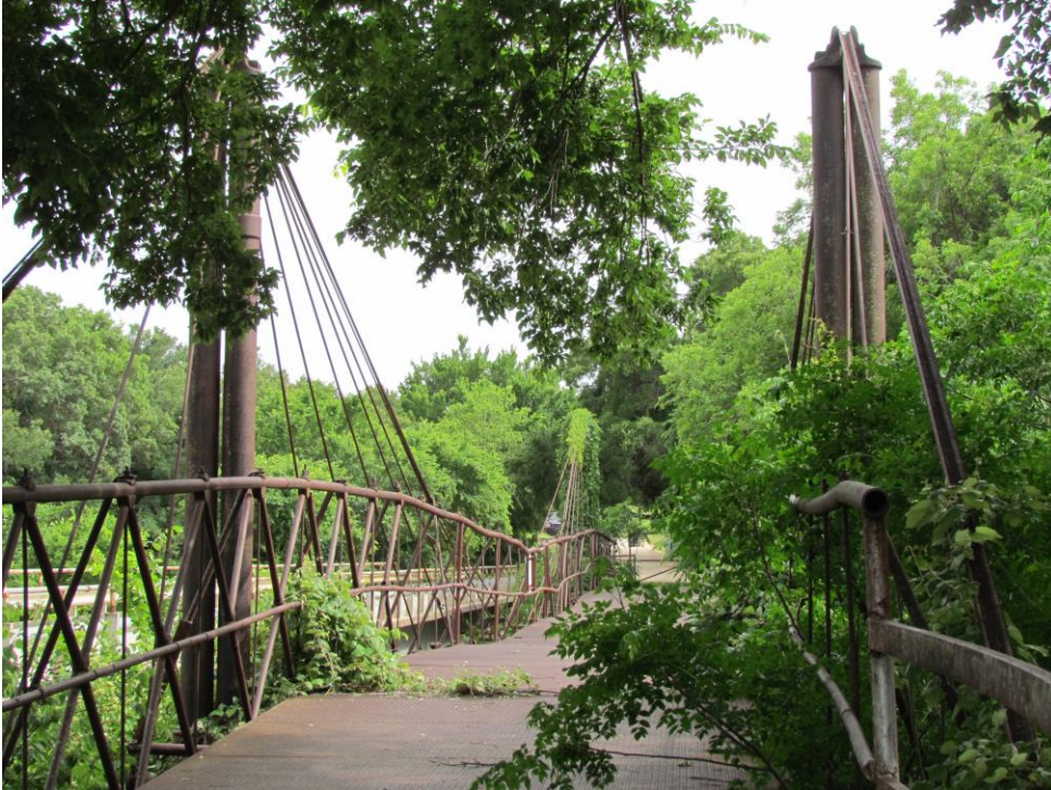
TX_Erath County_Bluff Dale Bridge_0006.tif Barrel view, looking south
