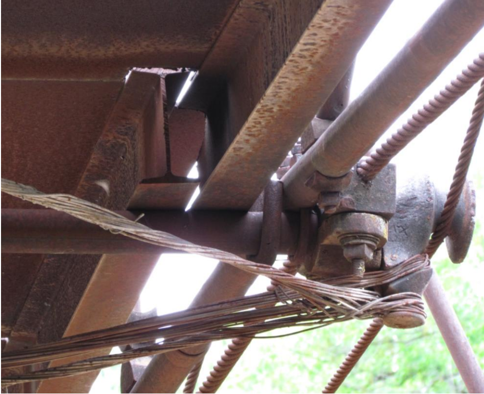
TX_Erath County_Bluff Dale Bridge_0020.tif Deck beam castings detail, looking northeast
