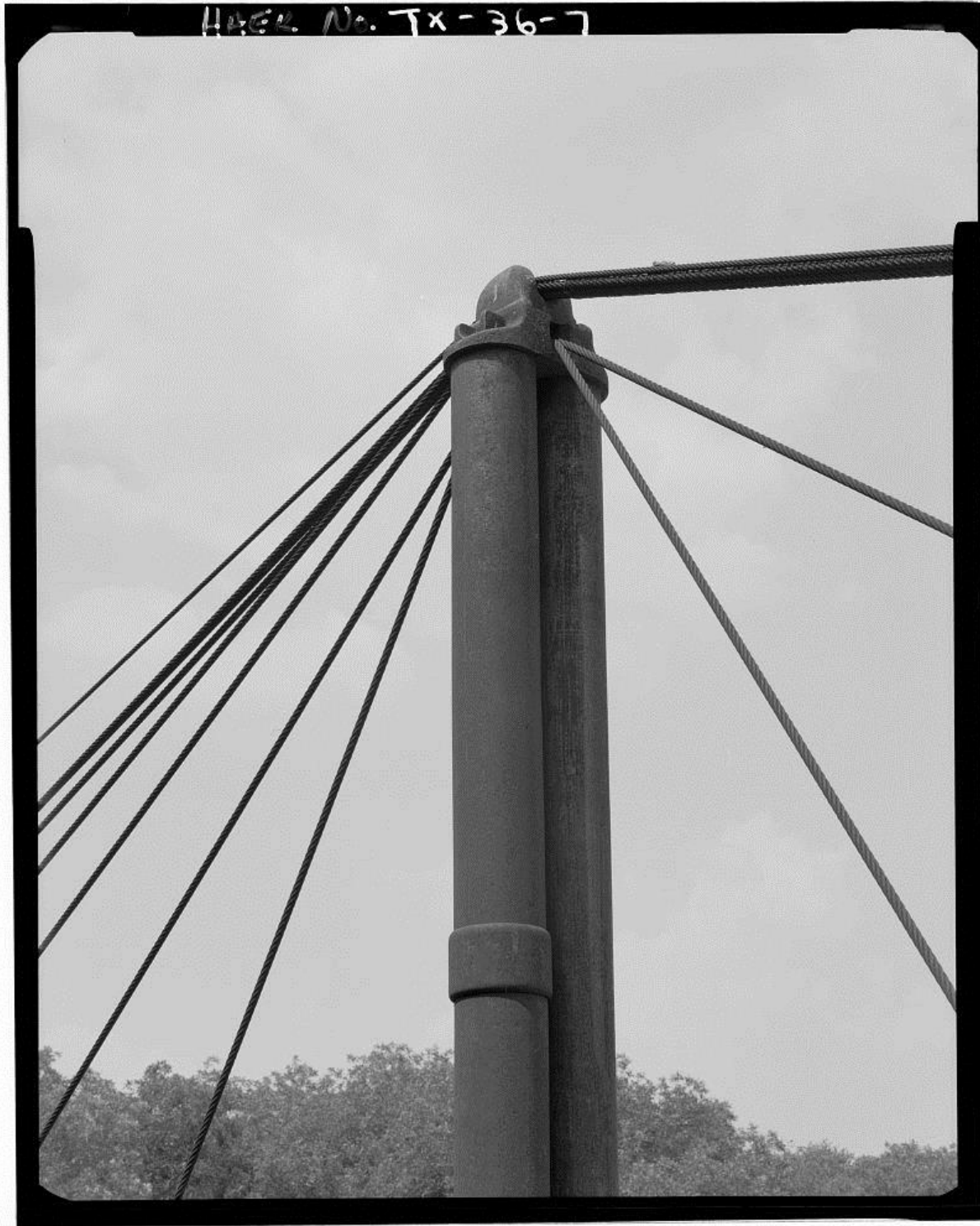
Figure 14: HAER TX-36 Photograph by Joseph E. B. Elliot (1996). Southeast column.
