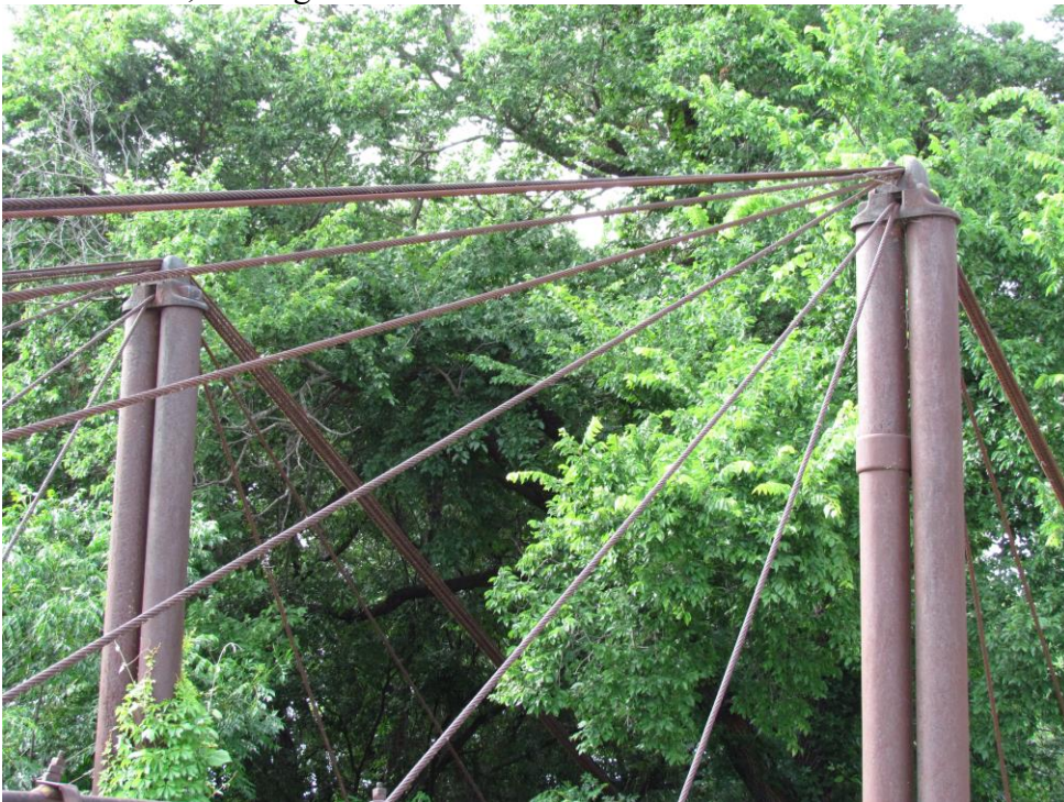
TX_Erath County_Bluff Dale Bridge_0007.tif North towers, looking northwest
