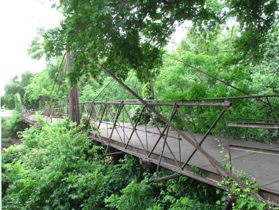
TX_Erath County_Bluff Dale Bridge_0008.tif North approach spans, looking southwest
