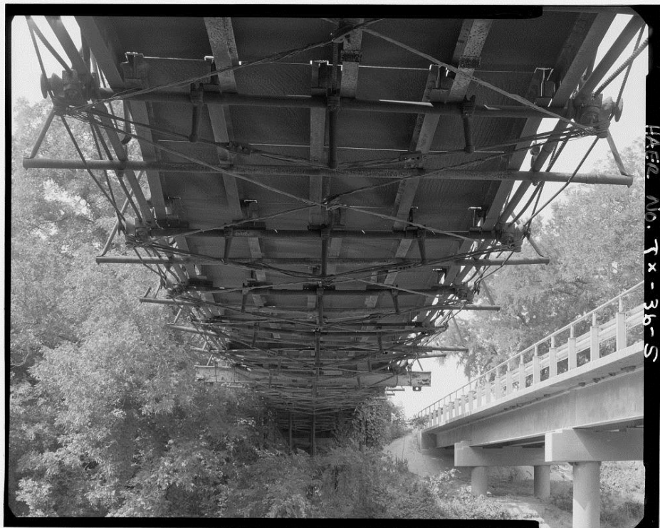
Figure 11: HAER TX-36 Photograph by Joseph E. B. Elliot (1996). Underside, from south.
