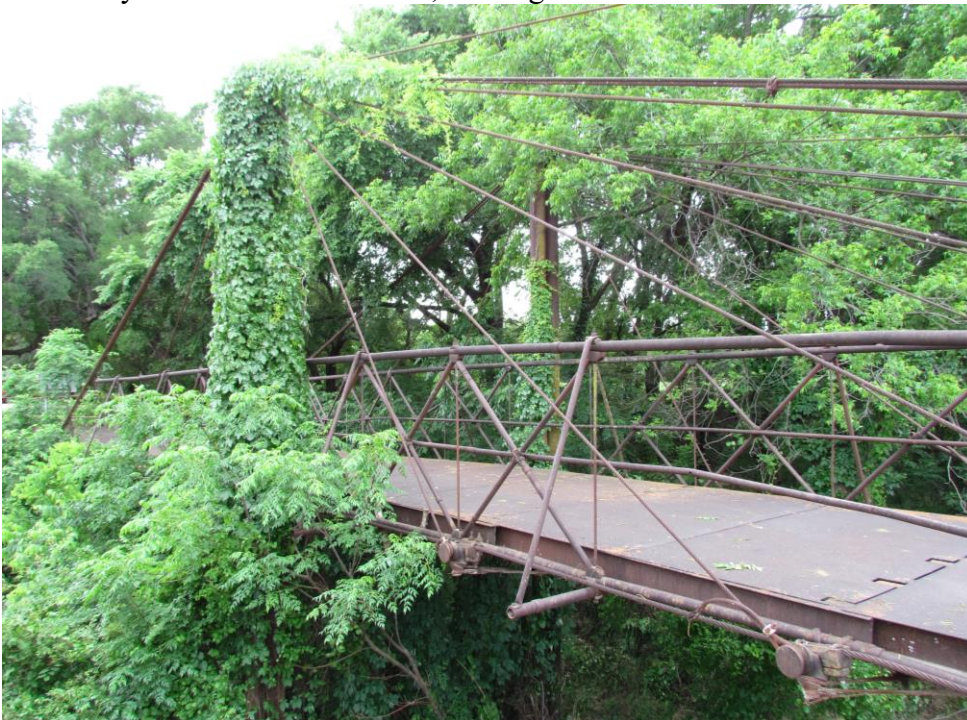
TX_Erath County_Bluff Dale Bridge_0009.tif Cable stays and deck connections, looking southwest
