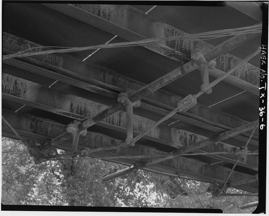
Figure 12: HAER TX-36 Photograph by Joseph E. B. Elliot (1996). 3/4 view floor beam.
