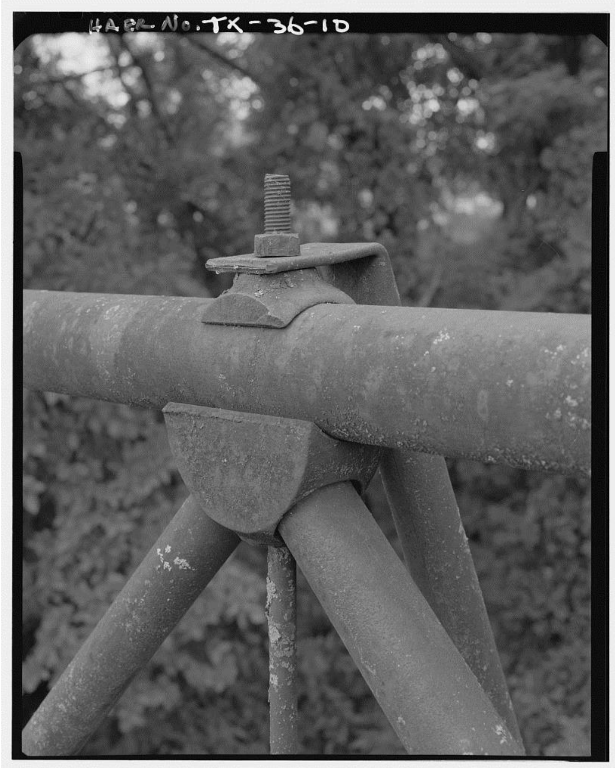
Figure 17: HAER TX-36 Photograph by Joseph E. B. Elliot (1996). Detail of typical railing support.
