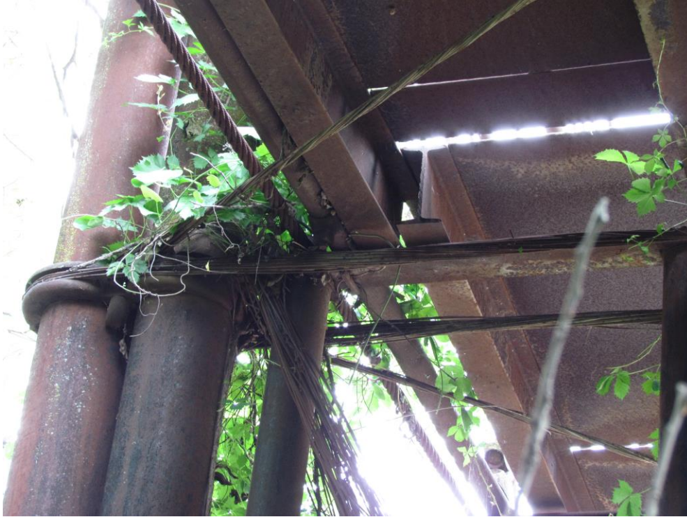
TX_Erath County_Bluff Dale Bridge_0016.tif Patented tower and bent connections, looking northwest
