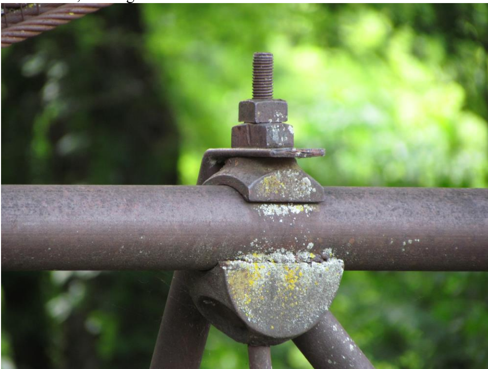
TX_Erath County_Bluff Dale Bridge_0015.tif Truss detail, looking west northwest
