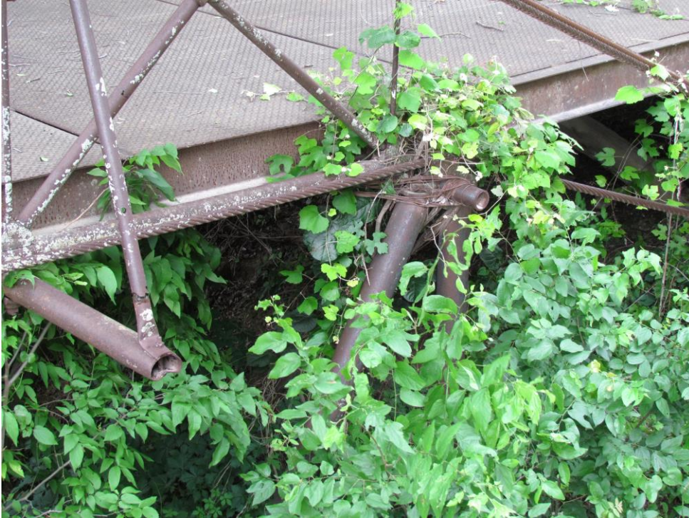
TX_Erath County_Bluff Dale Bridge_0014.tif Detail of patented deck connection, looking northwest
