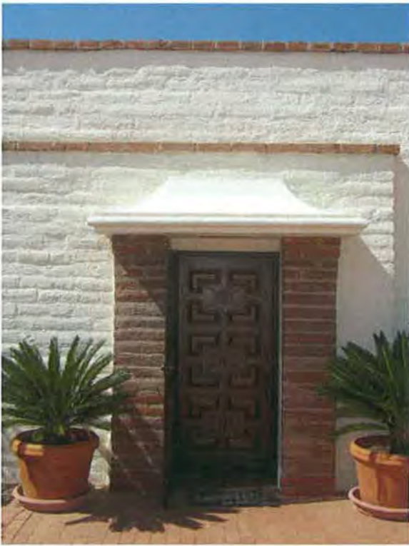
Photograph #11 (Left) Front door detail showing ornamental surround, and carved Mexican hardwood door, camera facing southeast.
