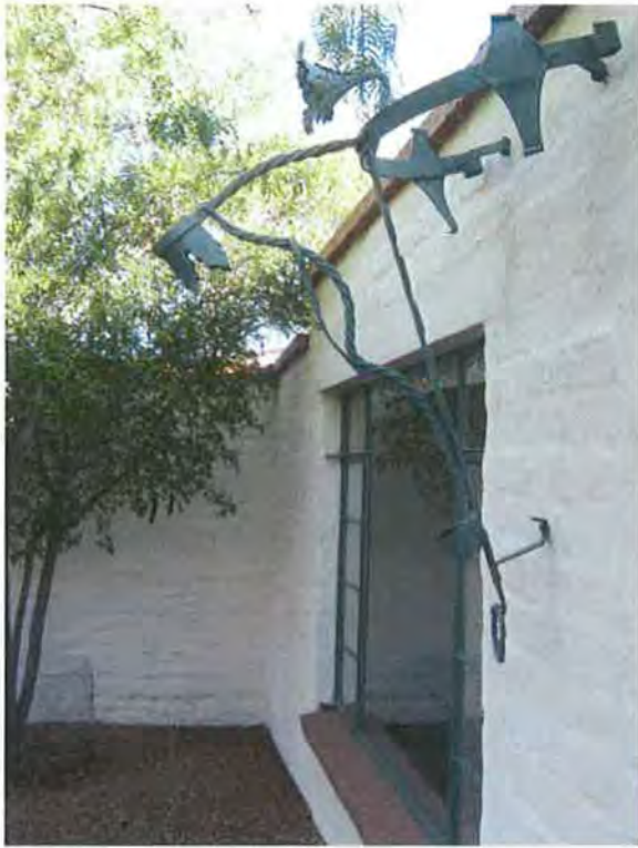
Photograph #9 (Left) Detail of ornate decorative wrought iron flag pole stanchion mounted on wall of original garage (converted to interior living space 1964), camera facing southeast.
