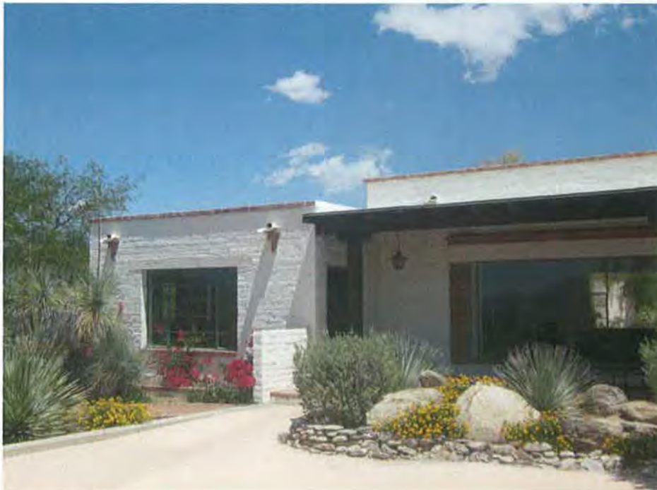
Photograph #18 Compatible dining room addition (Norvelle 1964) in footprint and location of portion of former rear porch; 8-foot window floods room with light and dramatic views; camera facing north.
