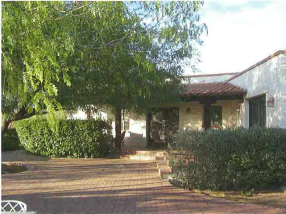
Photograph #21 South façade west end, camera facing northwest.
