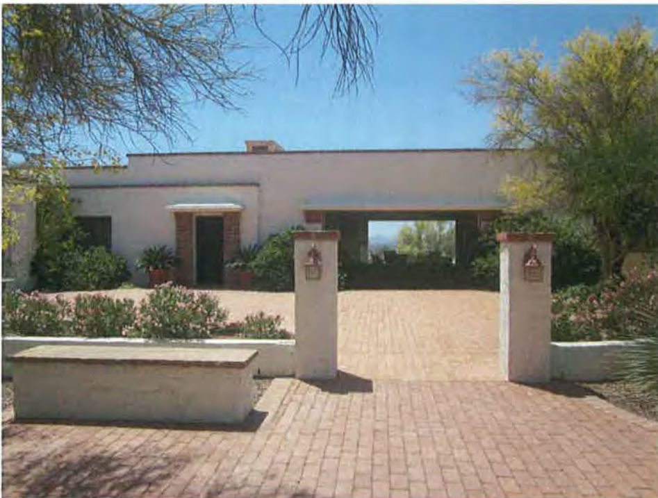
Photograph #6 View of front façade looking through north and south living room windows to desert and city in the distance, camera facing southwest.
