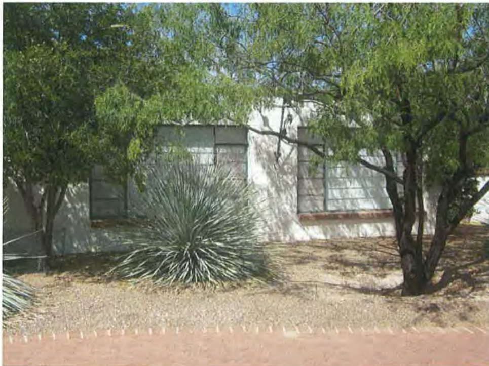
Photograph #8 Garage conversion (1964) detail of large casement windows (inspired by north living room window) in original garage door openings, camera facing southwest.
