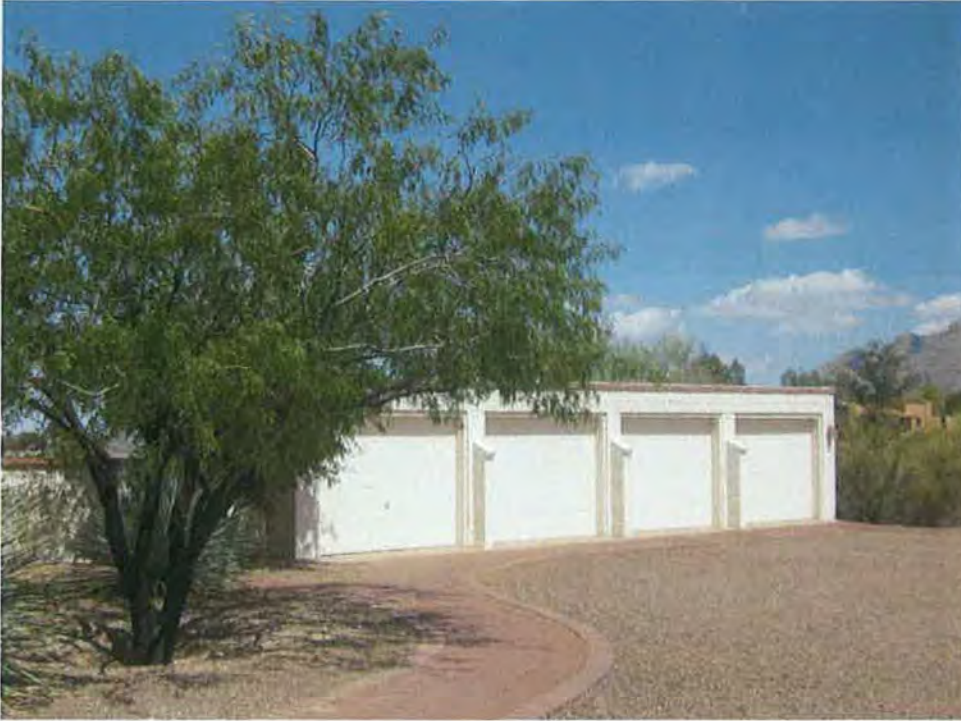
Photograph #27 Compatible free-standing garage (1964), camera facing northwest.
