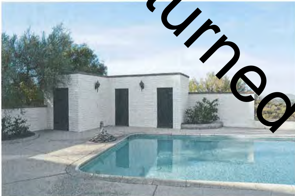
Photograph #28 Pool and compatible bath house(1970), camera facing southeast.
