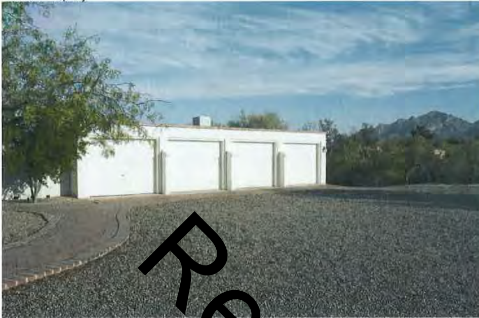
Photograph #27 Compatible free-standing garage (1960s), camera facing northwest.
