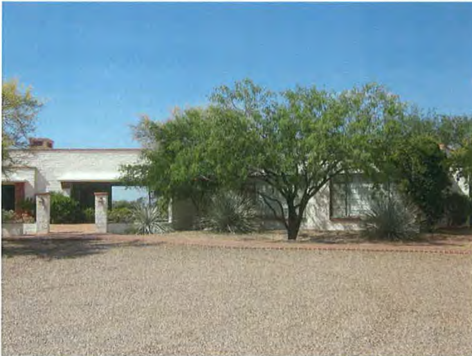
Photograph #7 Front façade, garage conversion (1964), camera facing southwest.
