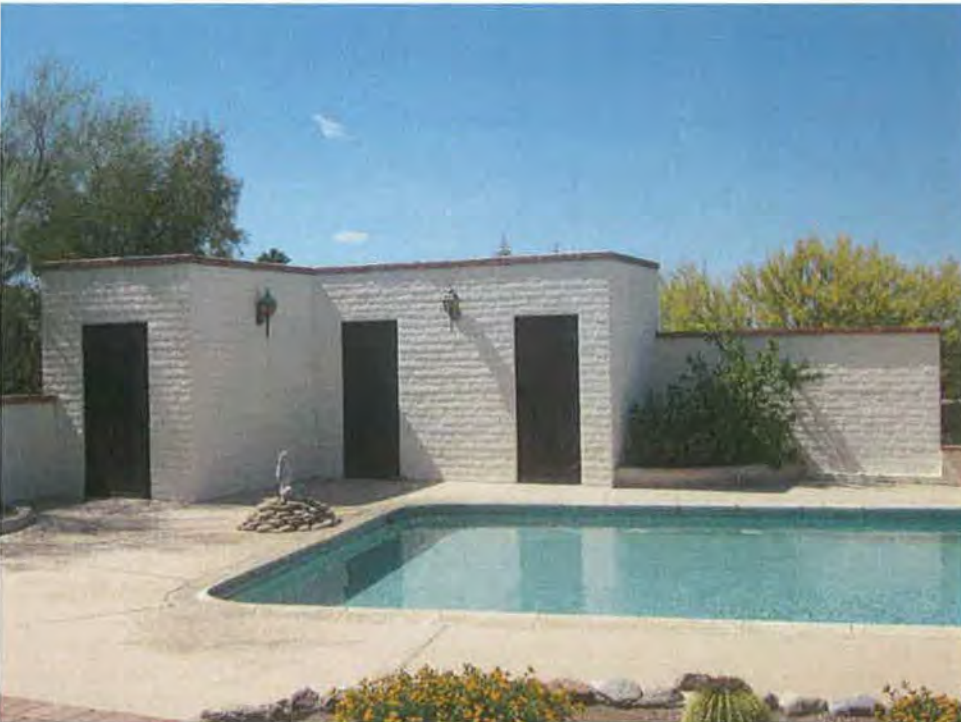
Photograph #28 Pool and compatible bath house(1970), camera facing southeast.
