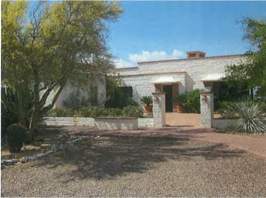
Photograph #5 Front (north) façade showing compatible Connector (1958) on east side bedroom wing, camera facing south.
