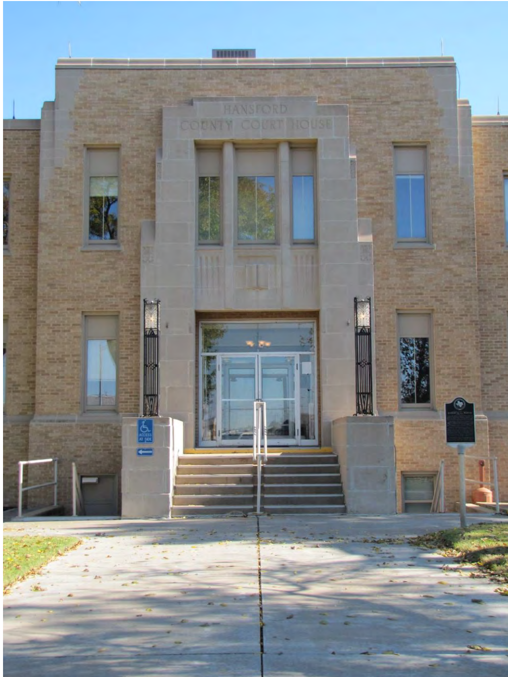
Photo 3: View of central entrance bay on primary (northwest) elevation. Camera facing southeast.
