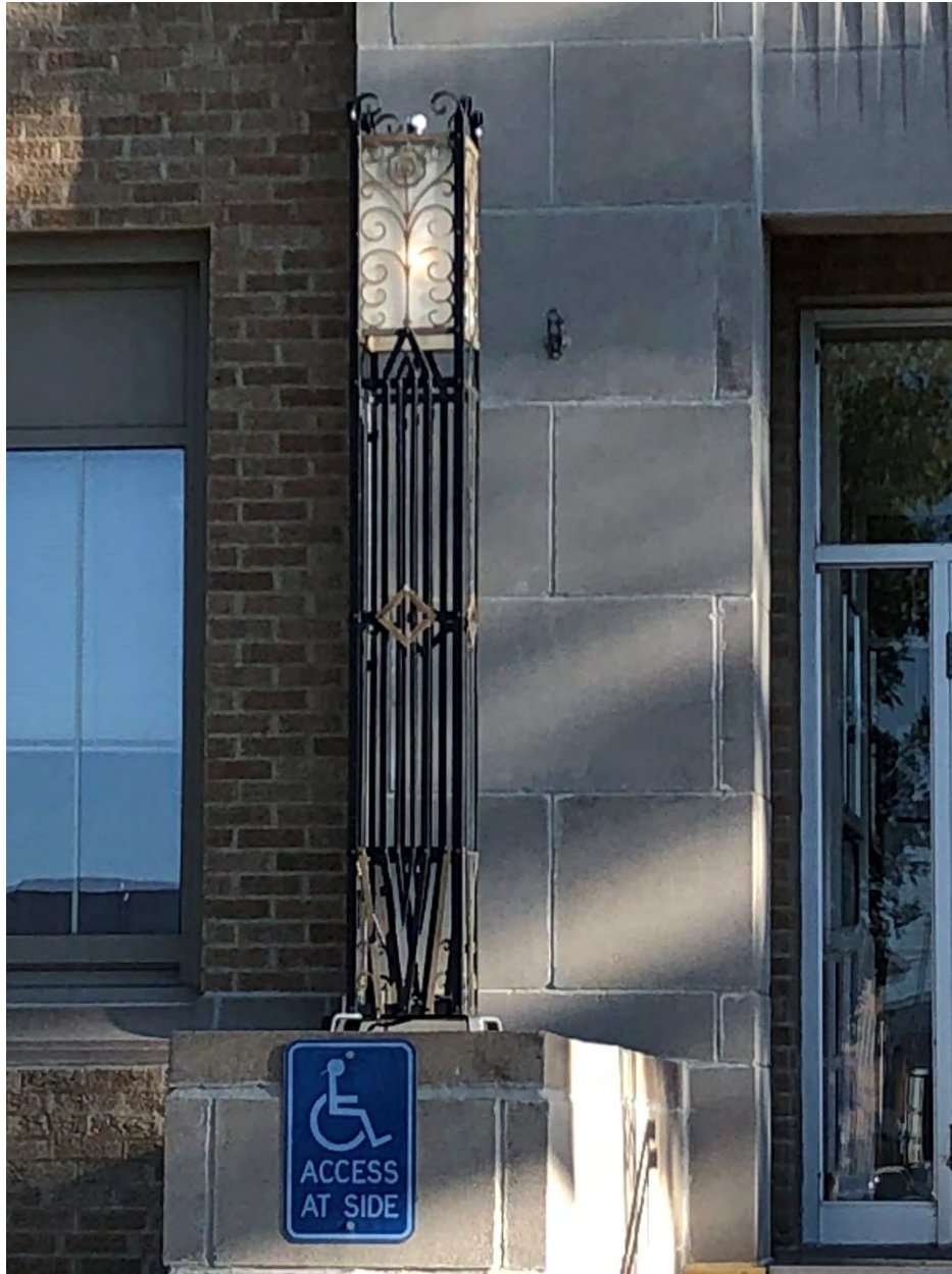
Photo 10: Decorative lamp post near main entrance.
