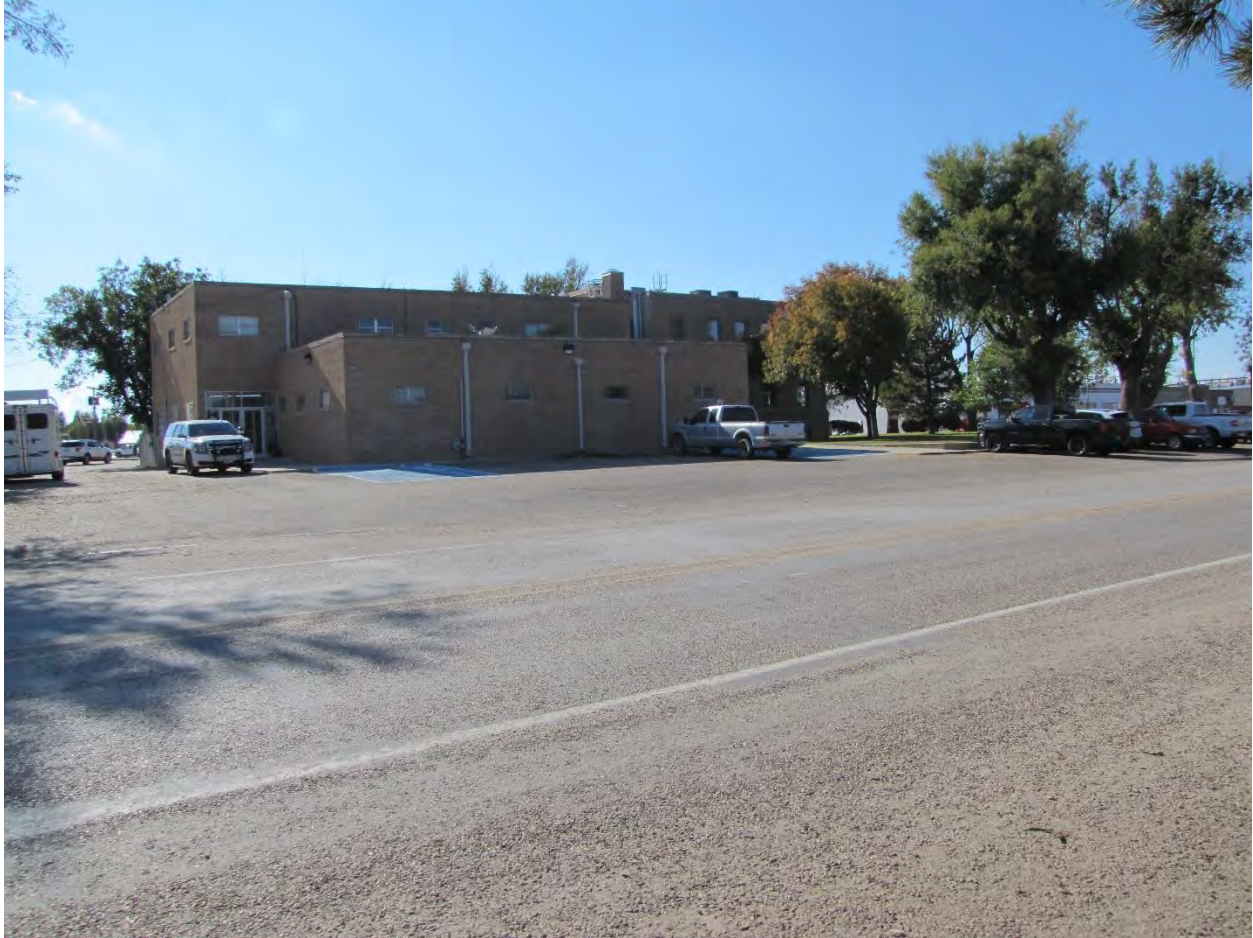
Photo 8: View of northeast elevation of the 1958 addition and the 1931 courthouse. Camera facing southwest.
