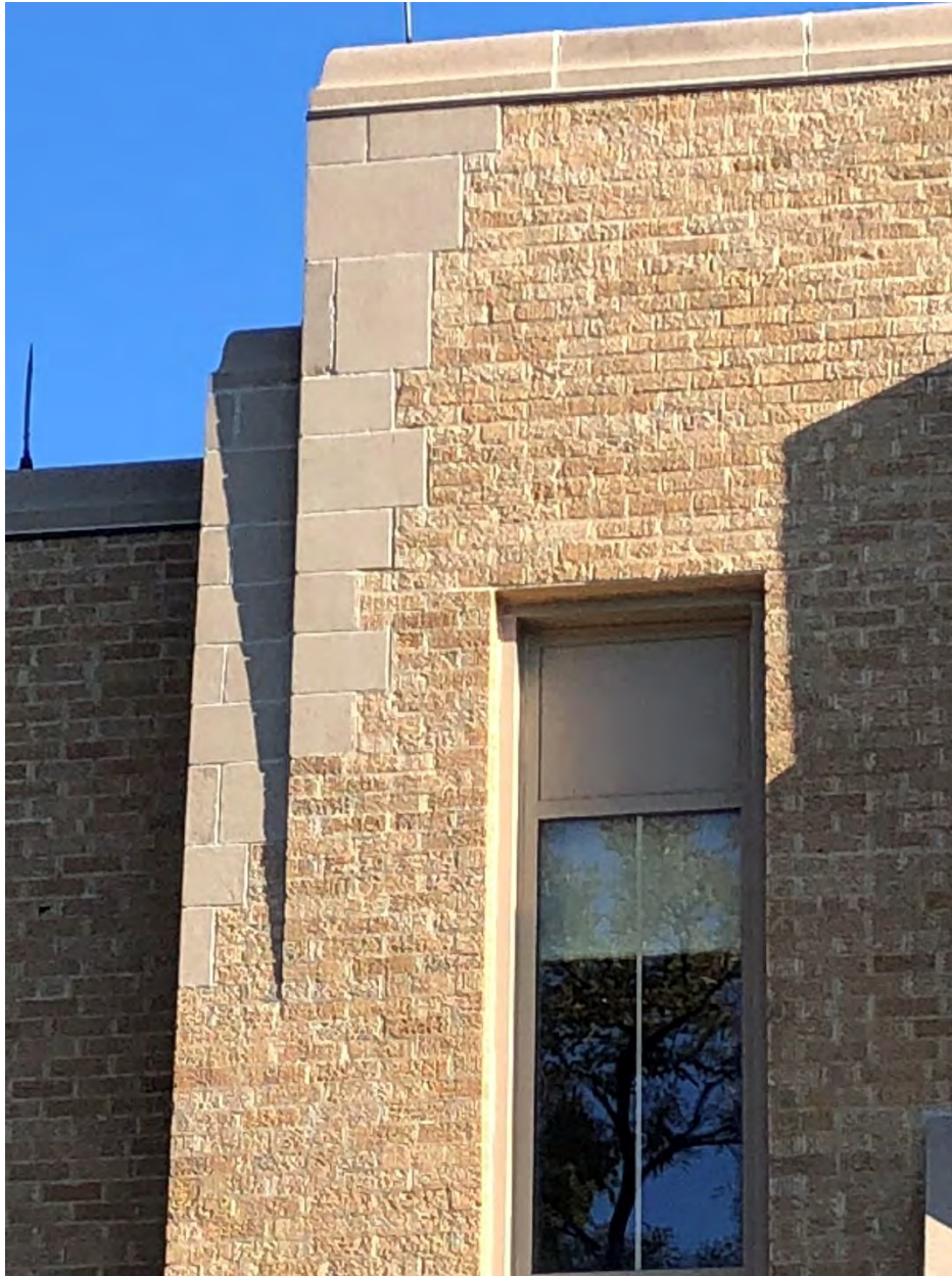
Photo 11: Stepped quoin detail on primary (northwest) elevation.
