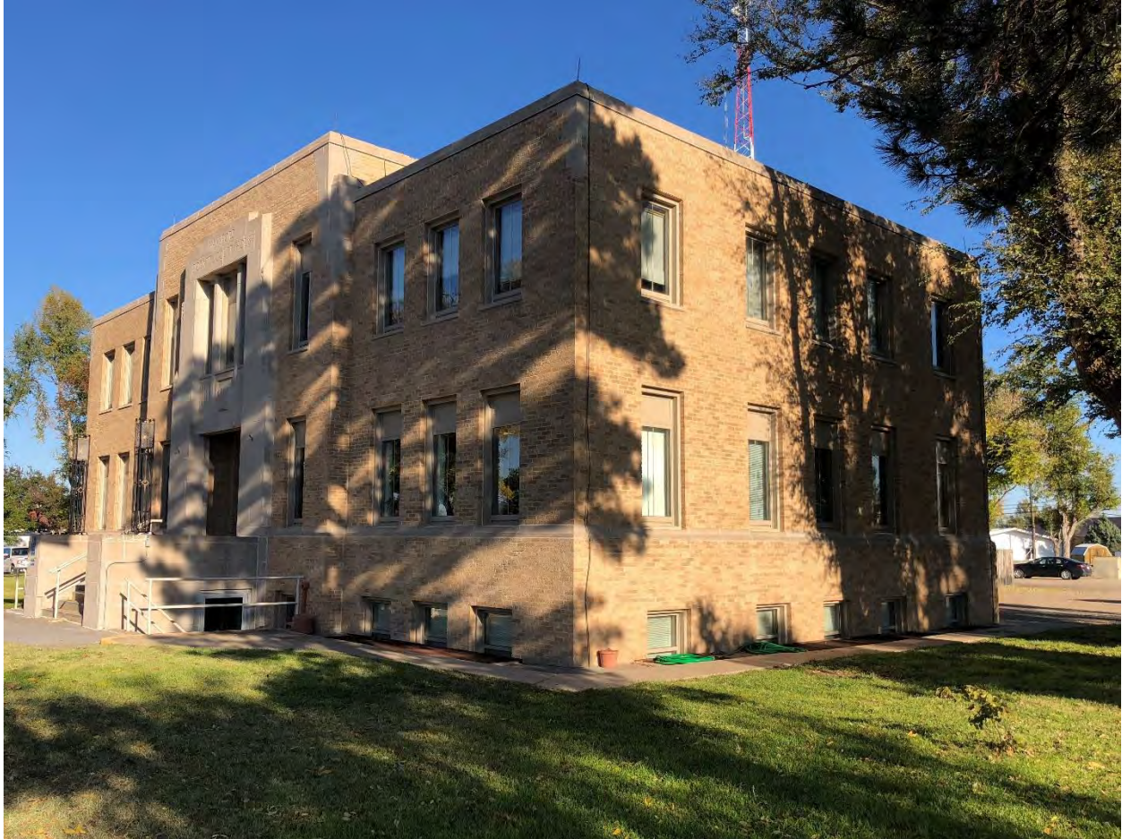
Photo 4: View of northwest and southwest elevations of 1931 courthouse. Camera facing east.
