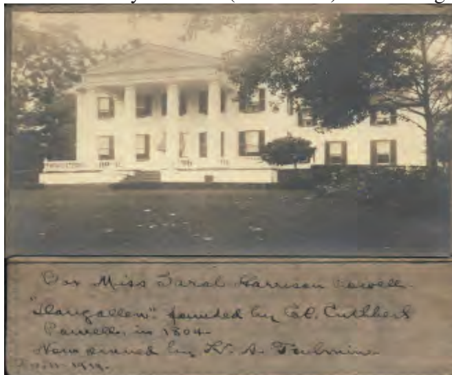
“Llangollen ... Now owned by A H Toulmin,” courtesy VDHR archives, showing double-story front porch addition; the Whitney south wing has not yet been built. The 1804 date of establishment has not been verified
