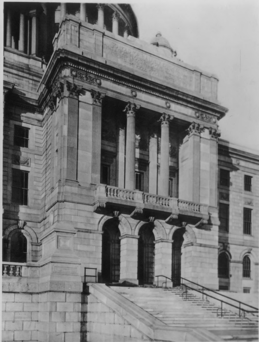
DETAIL OF MAIN ENTRANCE
