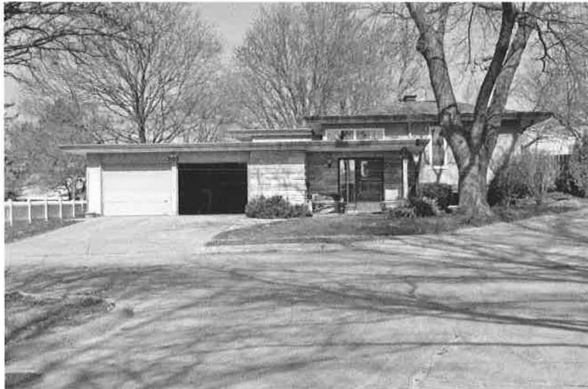
Waite Residence - Iowa City, Iowa Flat roofs at several levels, clearstory windows, articulated fascia
