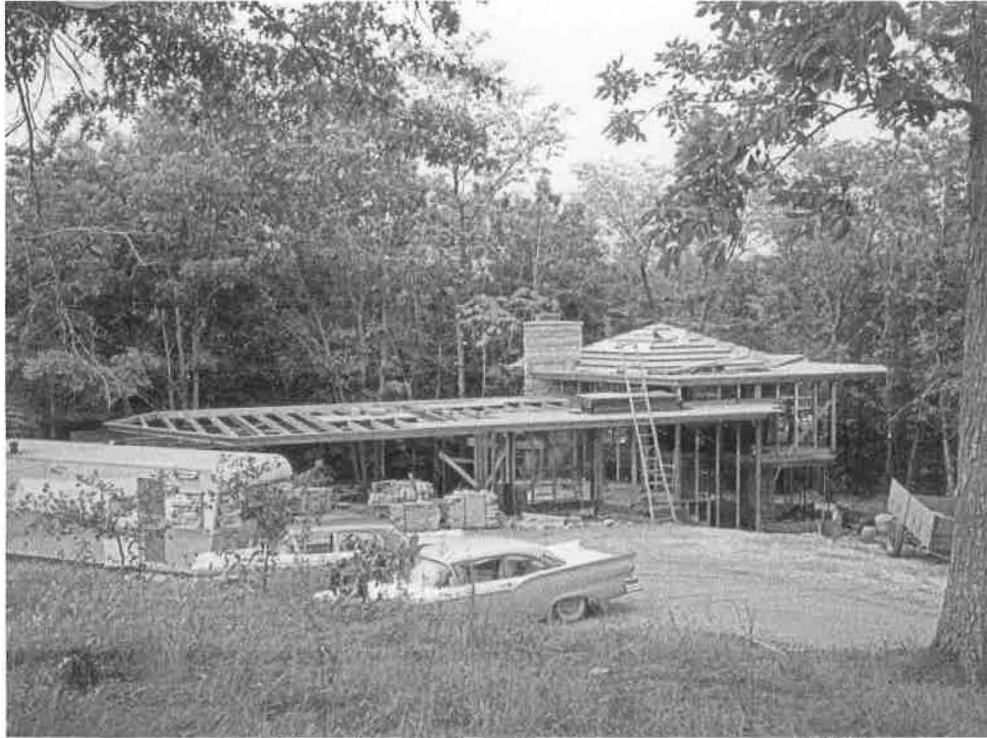
Summer, 1959. Carport is underway and Bermuda metal roof is being installed
