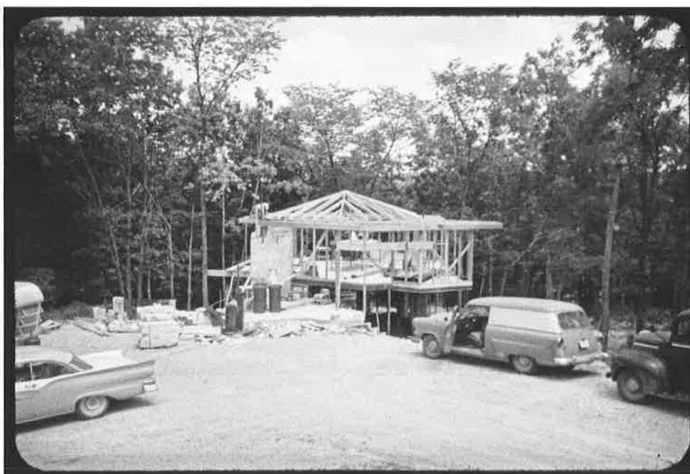
Summer, 1959, looking east. Framing for upper level underway.
