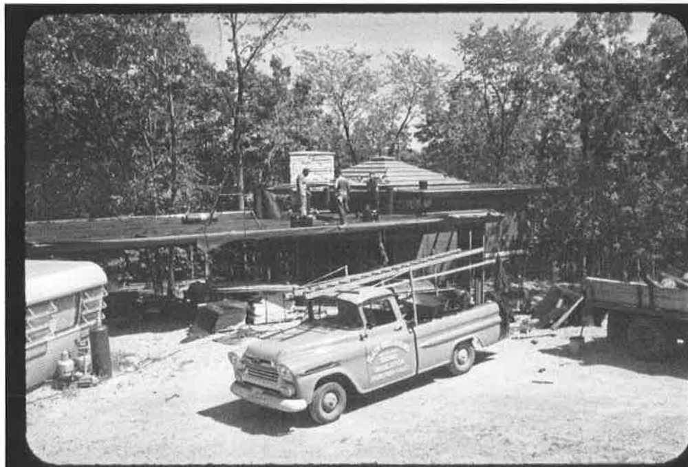
Summer, 1959. Bermuda roof and limestone chimney are complete, carport's tar and gravel roof underway.
