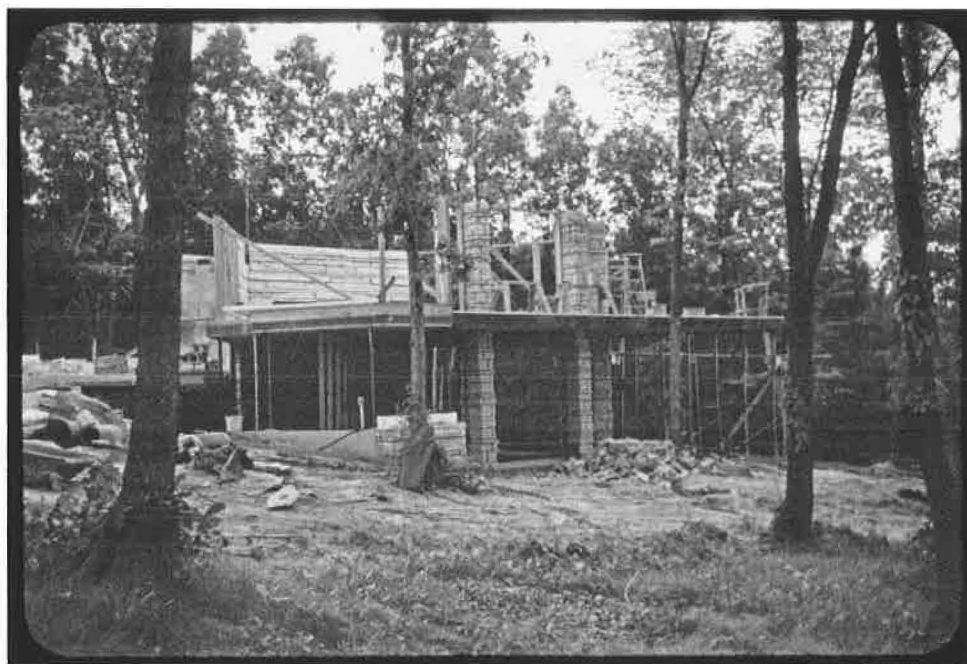
Summer, 1959, photo of south side, looking north. Upper level floor is finished, north wall is well underway, as is the fireplace box and chimney.
