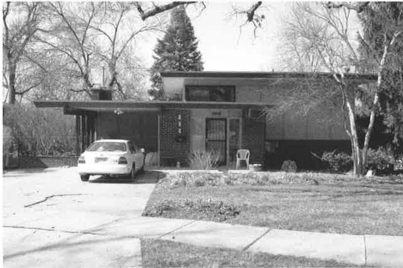
Doderer Residence - Iowa City, Iowa Flat roofs, clearstory windows, articulated fascia
