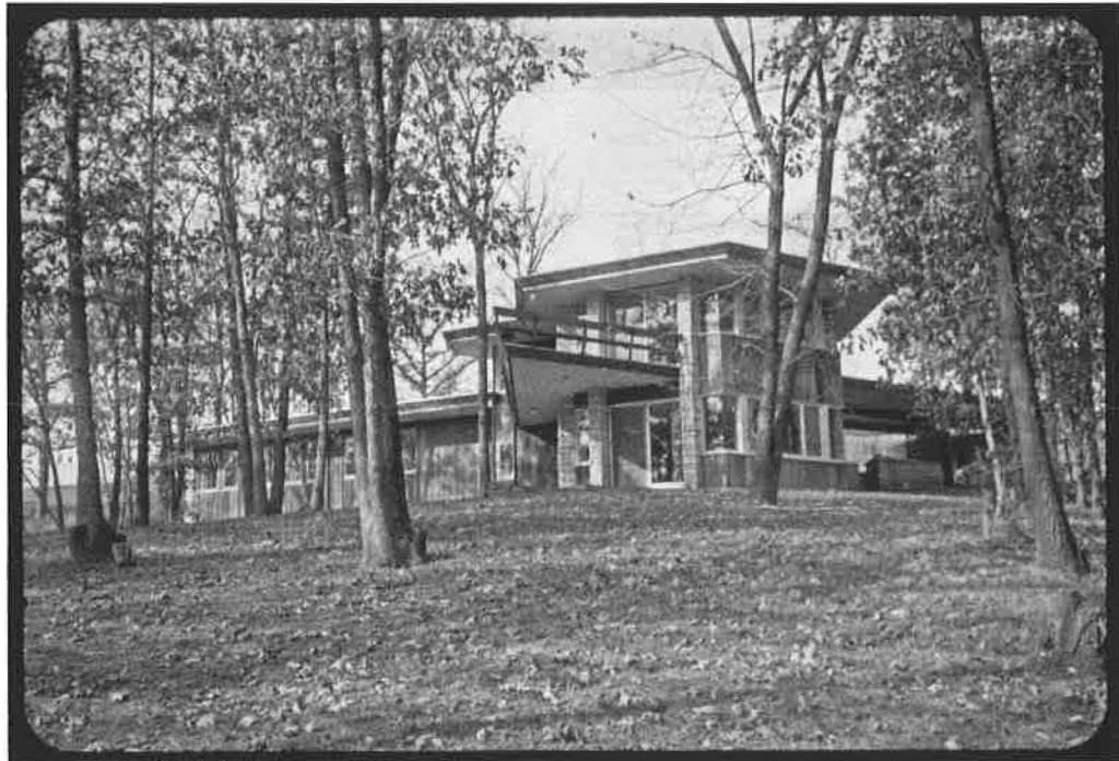
Fall, 1965, east side looking west. The living pavilion with its cantilevered deck is in the center; the carport to the right and the bedroom wing to the left.
