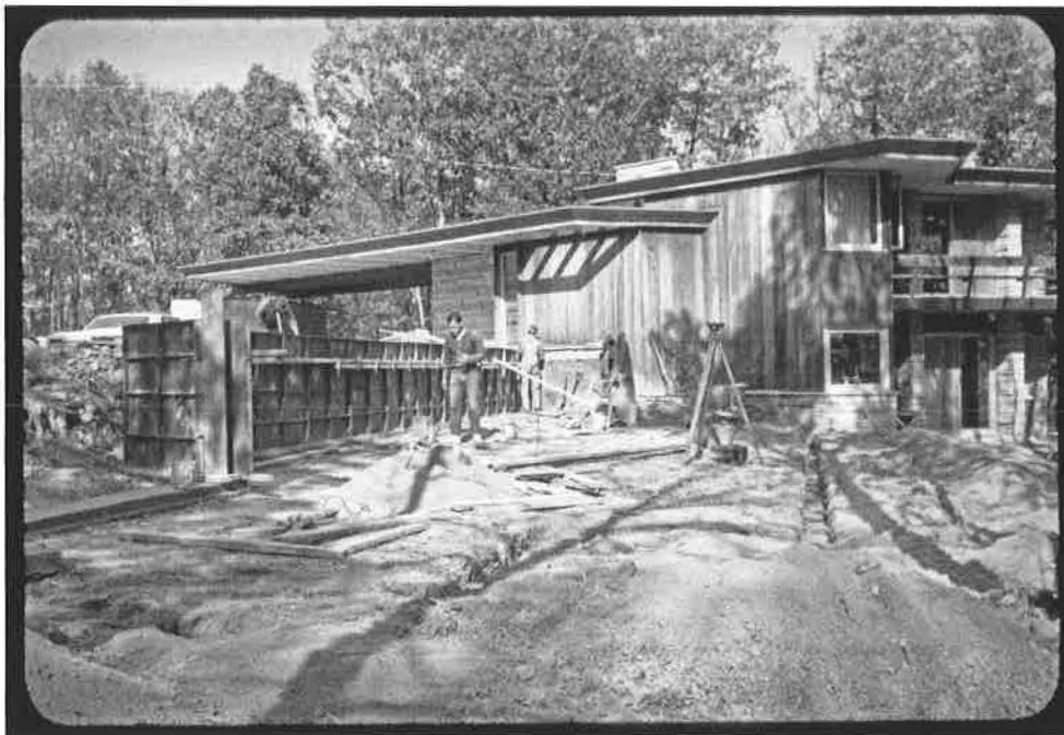
Fall, 1964, looking north at the bedroom wing foundation walls under construction.
