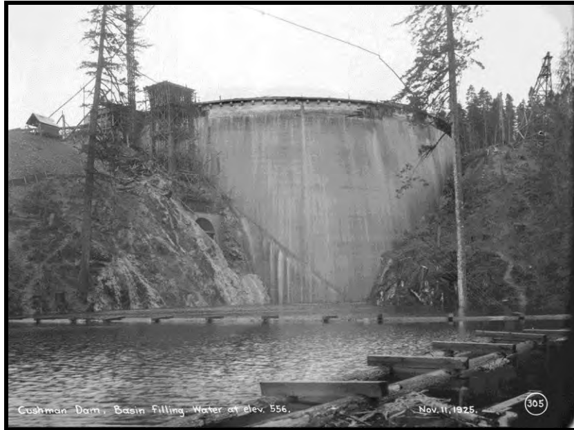
Figure 5. Cushman No. 1 dam and power intake, November 11, 1925. Image courtesy of Tacoma Power.
