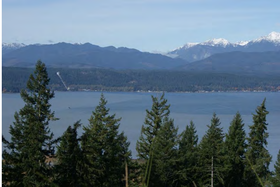
Photo 44. Cushman No. 2 as viewed west across the Hood Canal. Note the surge tank and penstocks clearly visible on the landscape.
