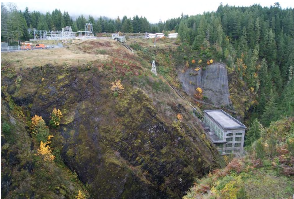
Photo 2. Viewing east from the Cushman No. 1 dam parapet to other resources at the site, including (from left to right) the substation and switchyard, tram house, tram, modern tram warehouse/garage, storage garage, and Cushman No. 1 powerhouse.
