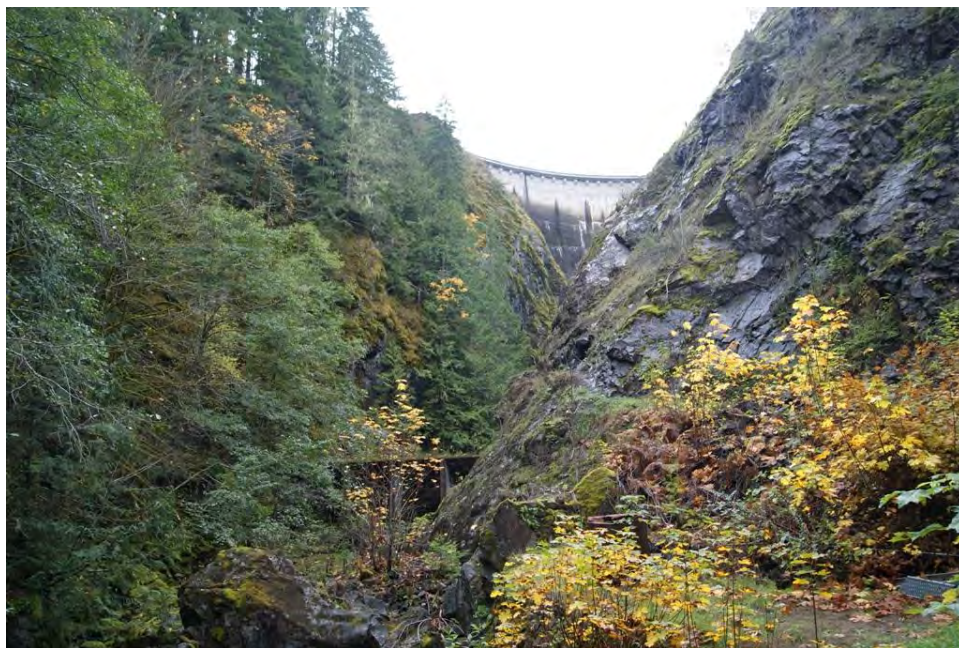
Photo 14. Cushman No. 1 dam, downstream face and buttress dam (center foreground), viewing west.
