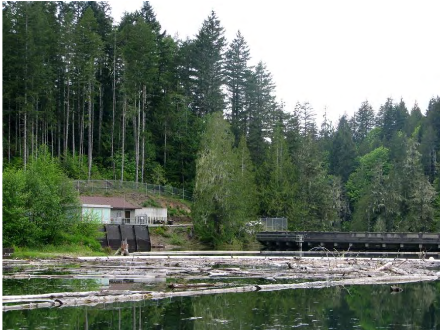
Photo 27. Cushman No. 2 resources, from left to right: Intake gate house, modern service house, and Cushman No. 2 dam, viewing west.
