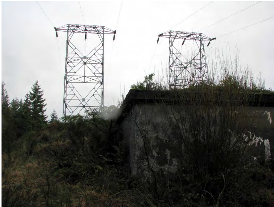
Photo 25. Concrete reservoir and transmission towers at Cushman No. 1, viewing east.
