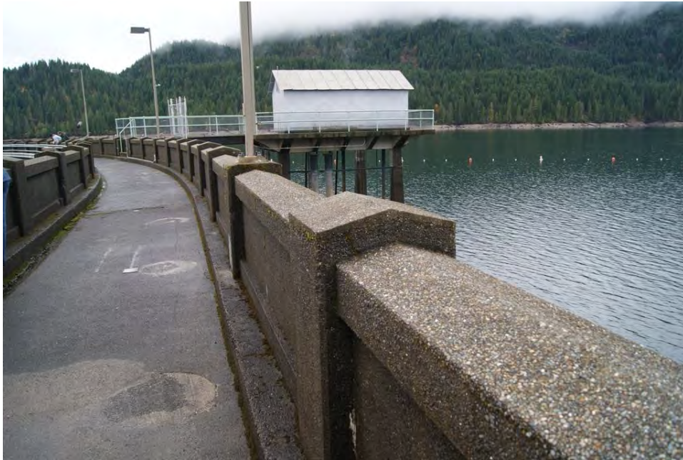
Photo 9. Cushman no. 1 dam parapet and intake house, viewing south.
