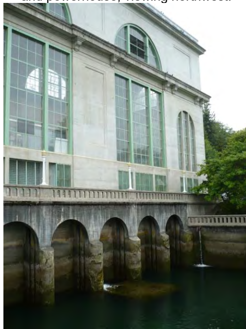
Photo 41. Cushman No. 2 powerhouse, viewing northwest.
