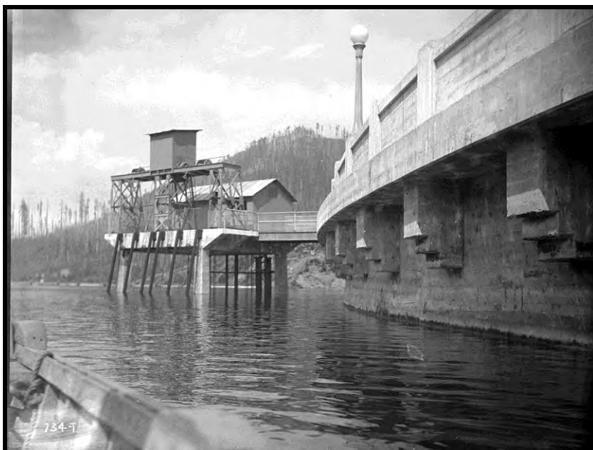
Figure 6. Cushman No. 1 intake gate house and platform, 1927. Image courtesy of Tacoma Power.
