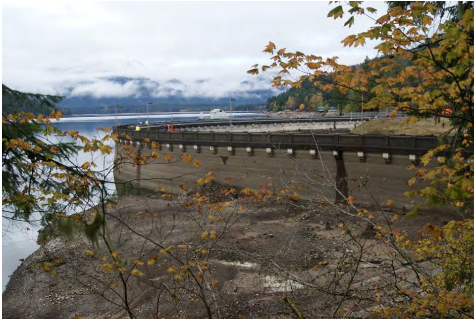
Photo 1. Cushman No. 1 dam, viewing north.
