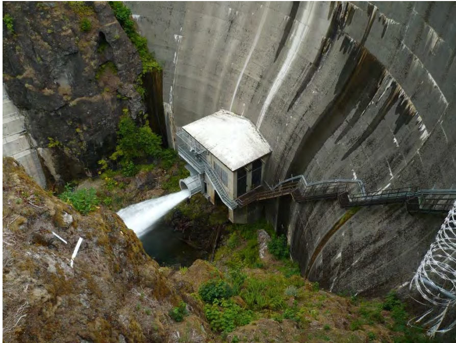
Photo 34. Cushman No. 2 valve house at base of dam.
