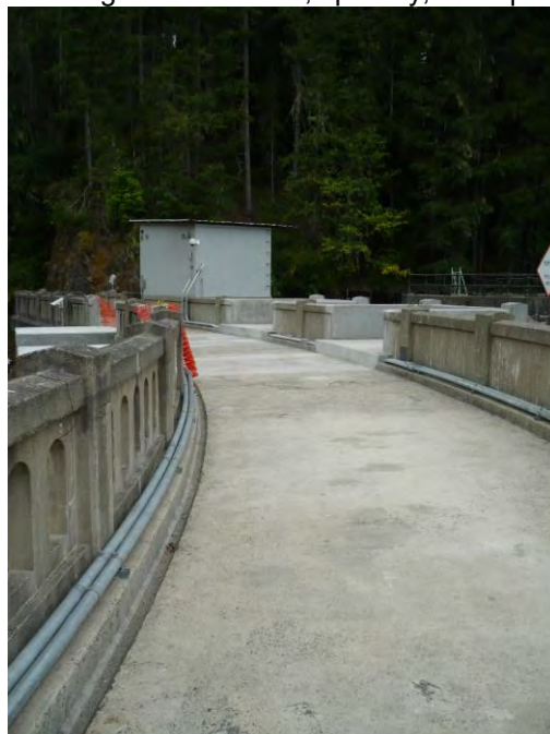
Photo 31. Cushman No. 2 dam parapet and spillway gatehouse, viewing north.
