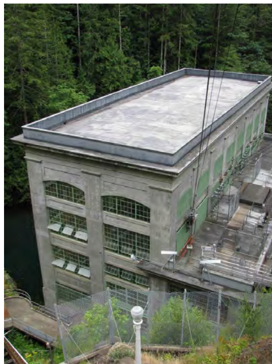
Photo 6. Cushman No. 1 powerhouse, viewing southwest.
