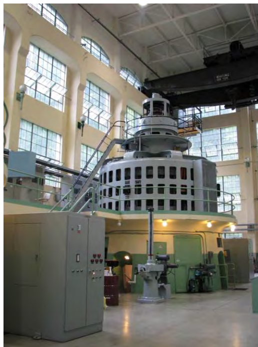
Photo 8. Cushman No. 1 powerhouse, interior.
