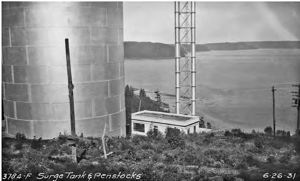
Figure 15. Cushman No. 2 surge tank and penstock gatehouse, June 26, 1931. Image courtesy of Tacoma Power.
