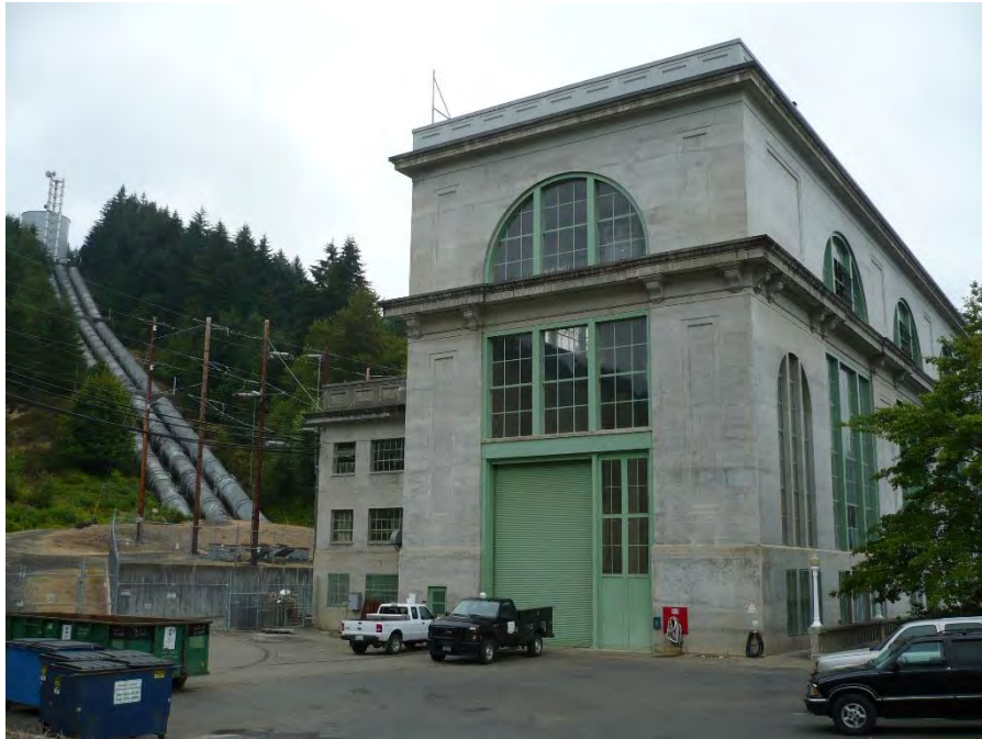
Photo 40. Cushman No. 2 resources, from left to right: Surge tank, vent pipes, penstocks, and powerhouse, viewing northwest.
