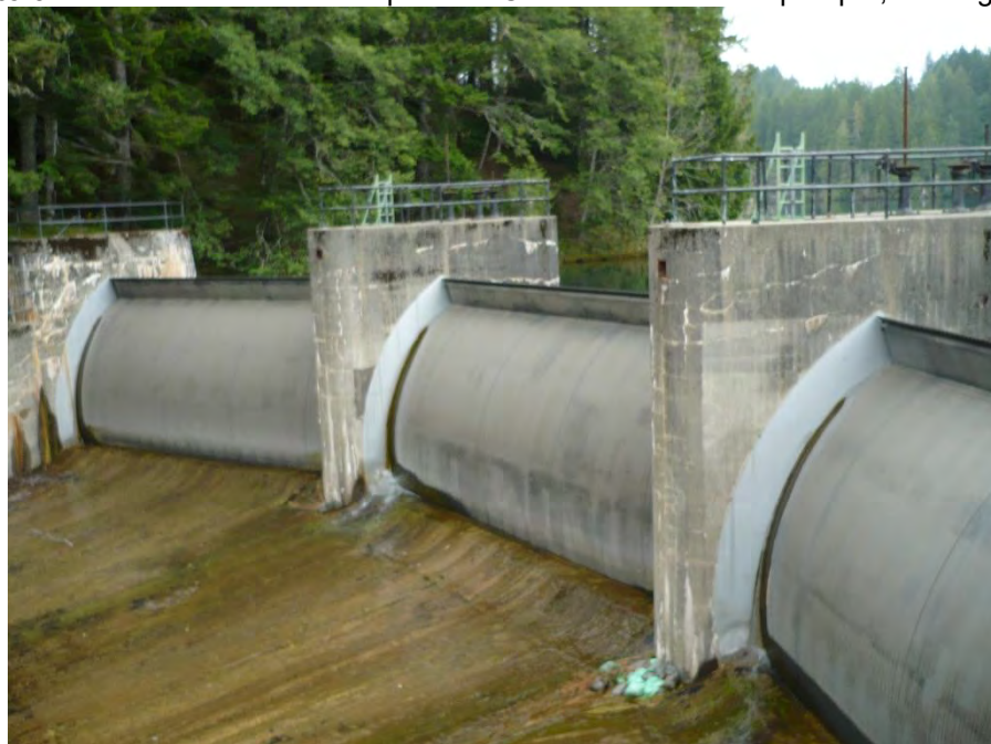
Photo 33. Cushman No. 2 spillway gates, viewing north.
