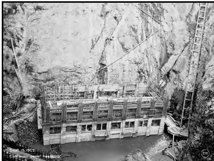
Figure 10. Cushman No. 1 powerhouse under construction, September 15, 1925. Image courtesy of Tacoma Power.
