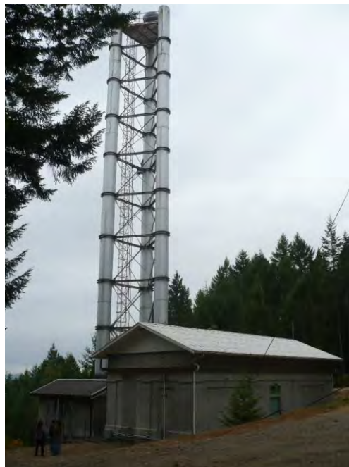
Photo 39. Cushman No. 2 valve gate house, vent pipes, and emergency generator building, viewing south.
