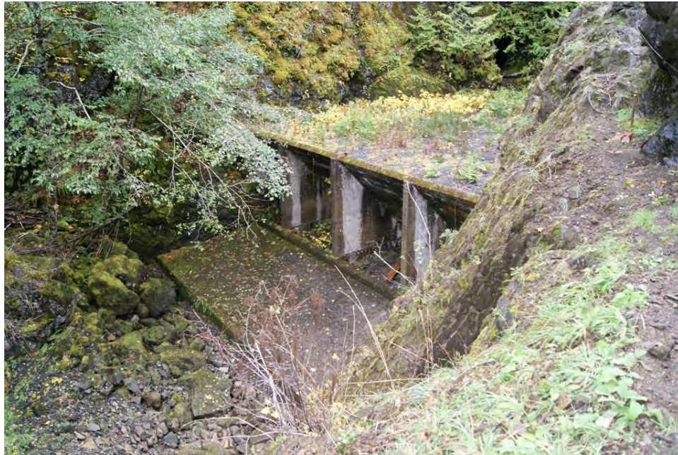
Photo 15. Buttress dam at base on Cushman No. 1 dam, viewing southwest.
