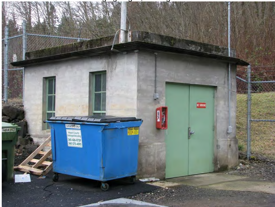
Photo 43. Cushman No.2 yard storage building, viewing south/southwest.
