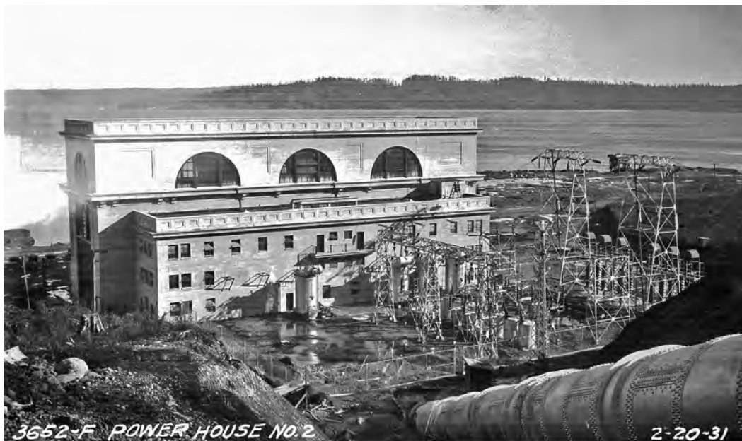
Figure 16. Cushman No. 2 powerhouse, February 20, 1931. Image courtesy of Tacoma Power.
