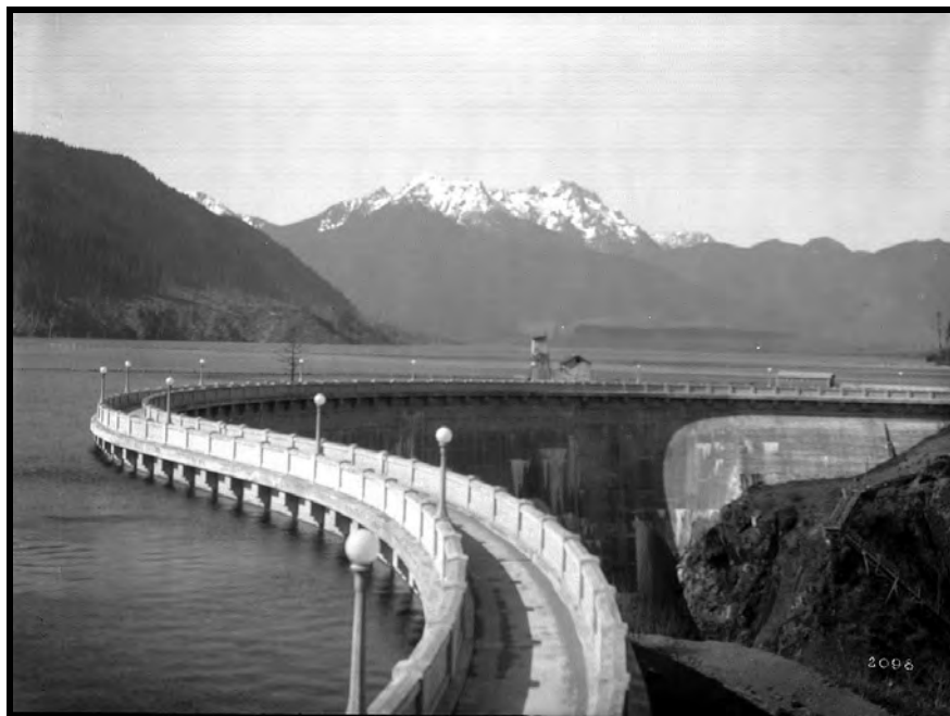
Figure 4. Cushman No. 1 dam, 1931. Image courtesy of Tacoma Power.
