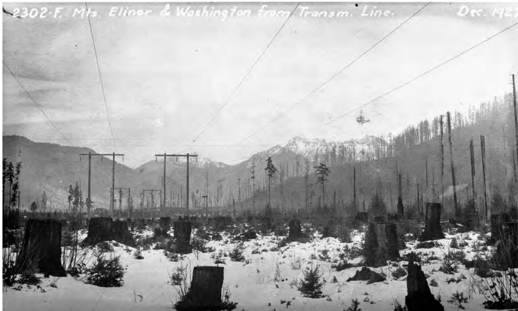
Figure 19. Potlatch (Cushman) Transmission Line, December 1927. Image courtesy of Tacoma Power.
