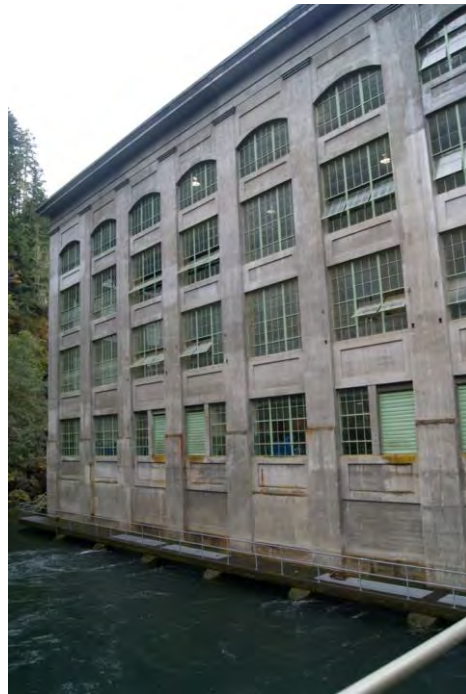
Photo 7. Cushman No. 1 powerhouse, viewing northwest.
