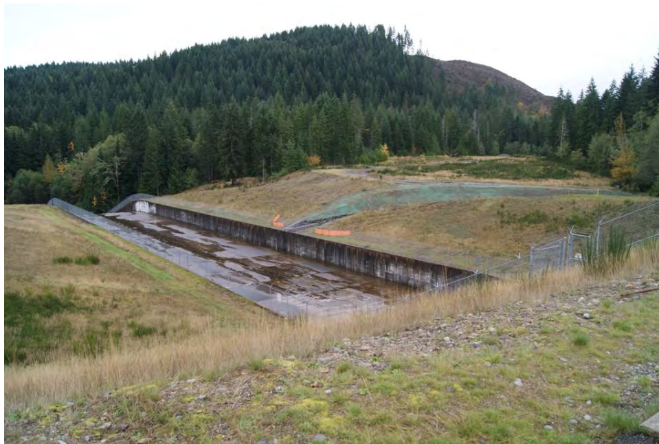
Photo 18. Viewing south, the modern spillway at Cushman No. 1.
