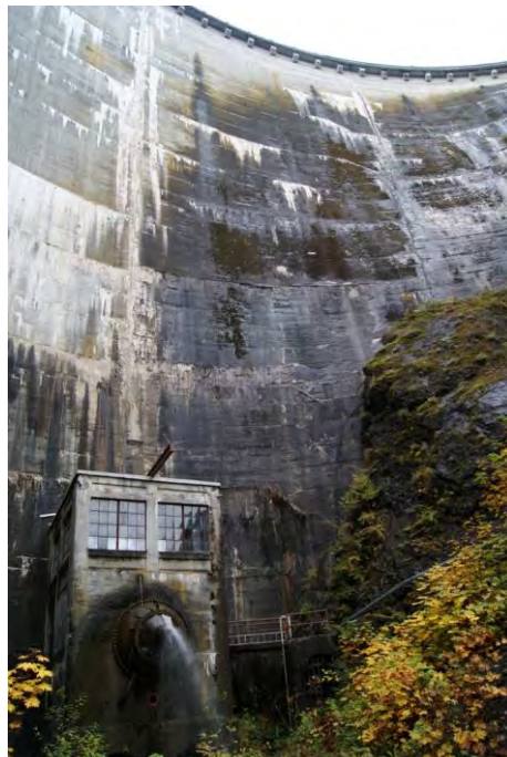
Photo 12. Cushman No. 1 valve house, viewing west.
