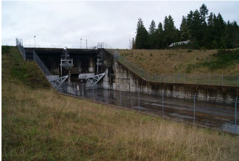
Photo 17. Downstream face of modern spillway at Cushman No. 1 Dam, viewing west/northwest.
