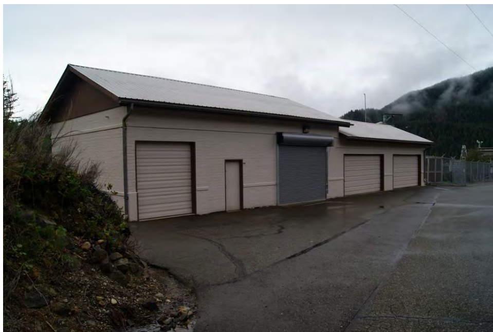
Photo 22. Cushman No. 1 warehouse/garage, viewing southwest.
