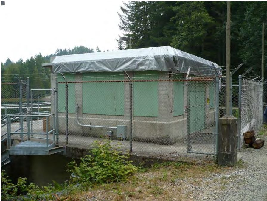
Photo 36. Cushman No. 2 Intake Gate House, viewing northeast.
