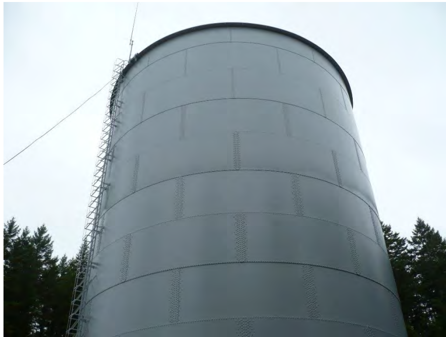
Photo 38. Cushman No. 2 surge tank.
