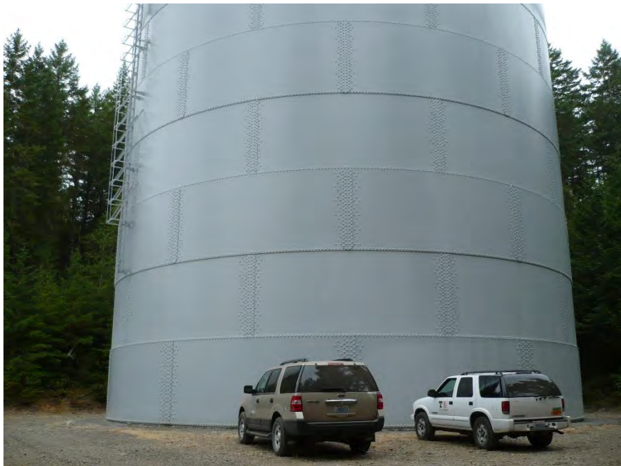
Photo 37. Cushman No. 2 surge tank, viewing southeast.
