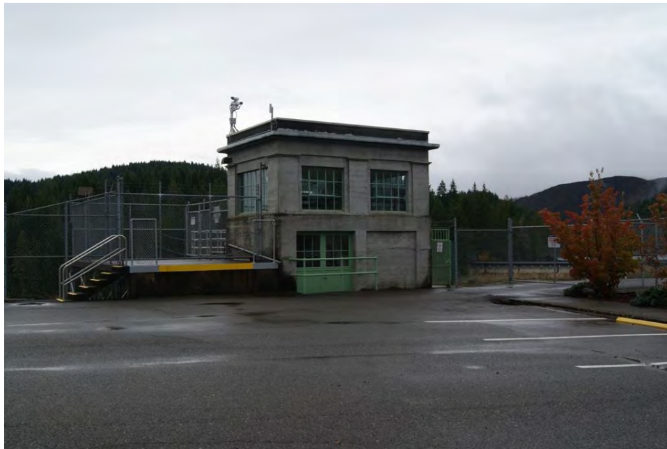
Photo 3. Cushman No. 1 tram house, viewing southwest.
