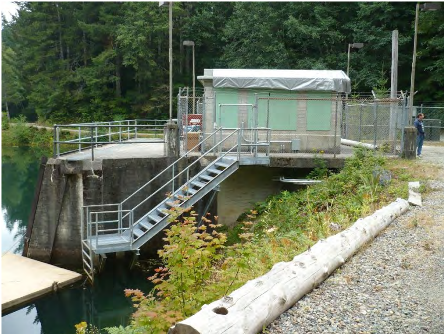
Photo 35. Cushman No. 2 Intake Gate House, viewing east.
