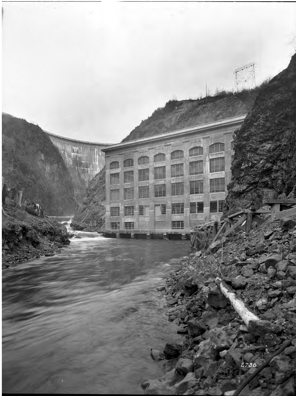
Figure 13. Cushman No.1 dam and powerhouse, 1933. Image courtesy of Tacoma Power.
