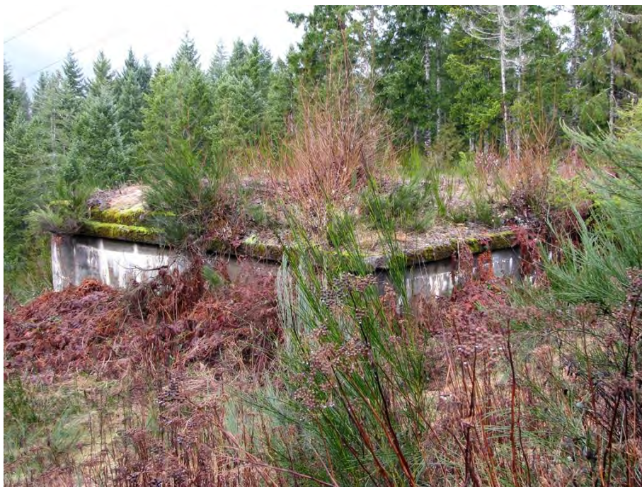
Photo 26. Concrete reservoir at Cushman No. 1, viewing northeast.
