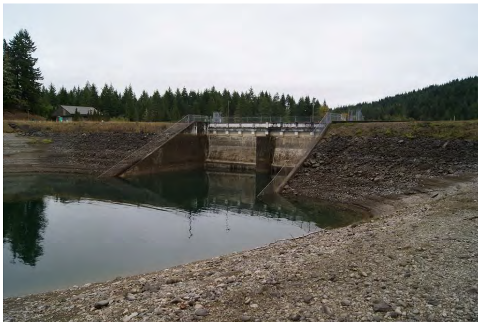
Photo 16. Upstream face of modern spillway at Cushman No. 1, viewing southwest.
