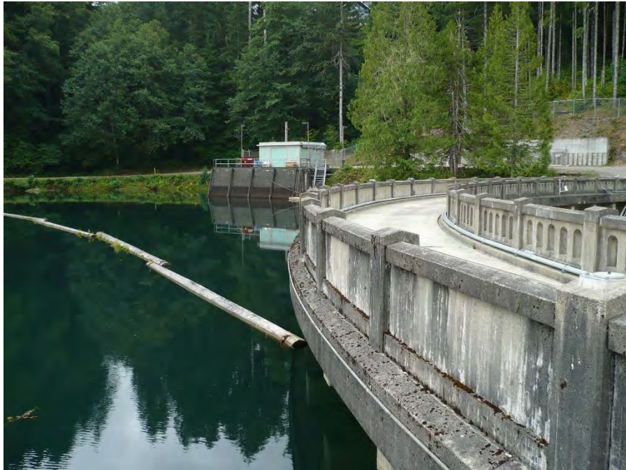
Photo 28. Cushman No. 2 dam parapet and intake house, viewing south.
