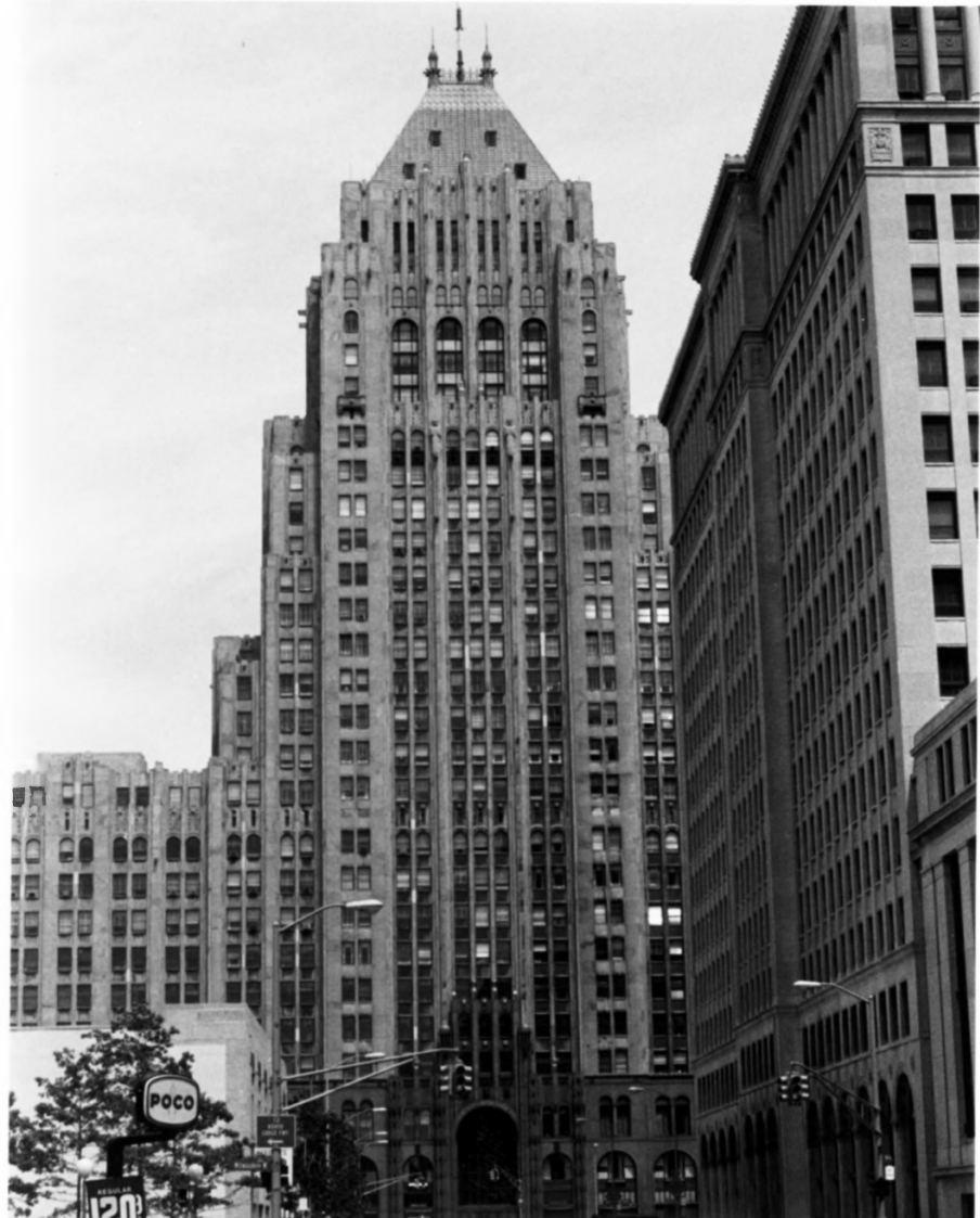
FISHER & NEW CENTER BUILDINGS, 3011 West Grand Blvd. and 7430 Second Avenue, Detroit, Wayne County, MI.
