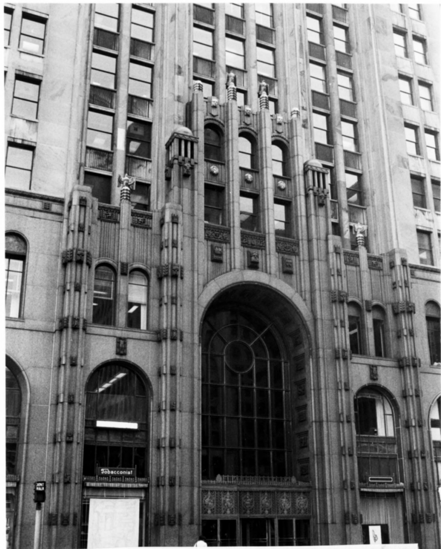
FISHER & NEW CENTER BUILDINGS, 3011 West Grand Blvd. and 7430 Second Avenue, Detroit, Wayne County, MI.
