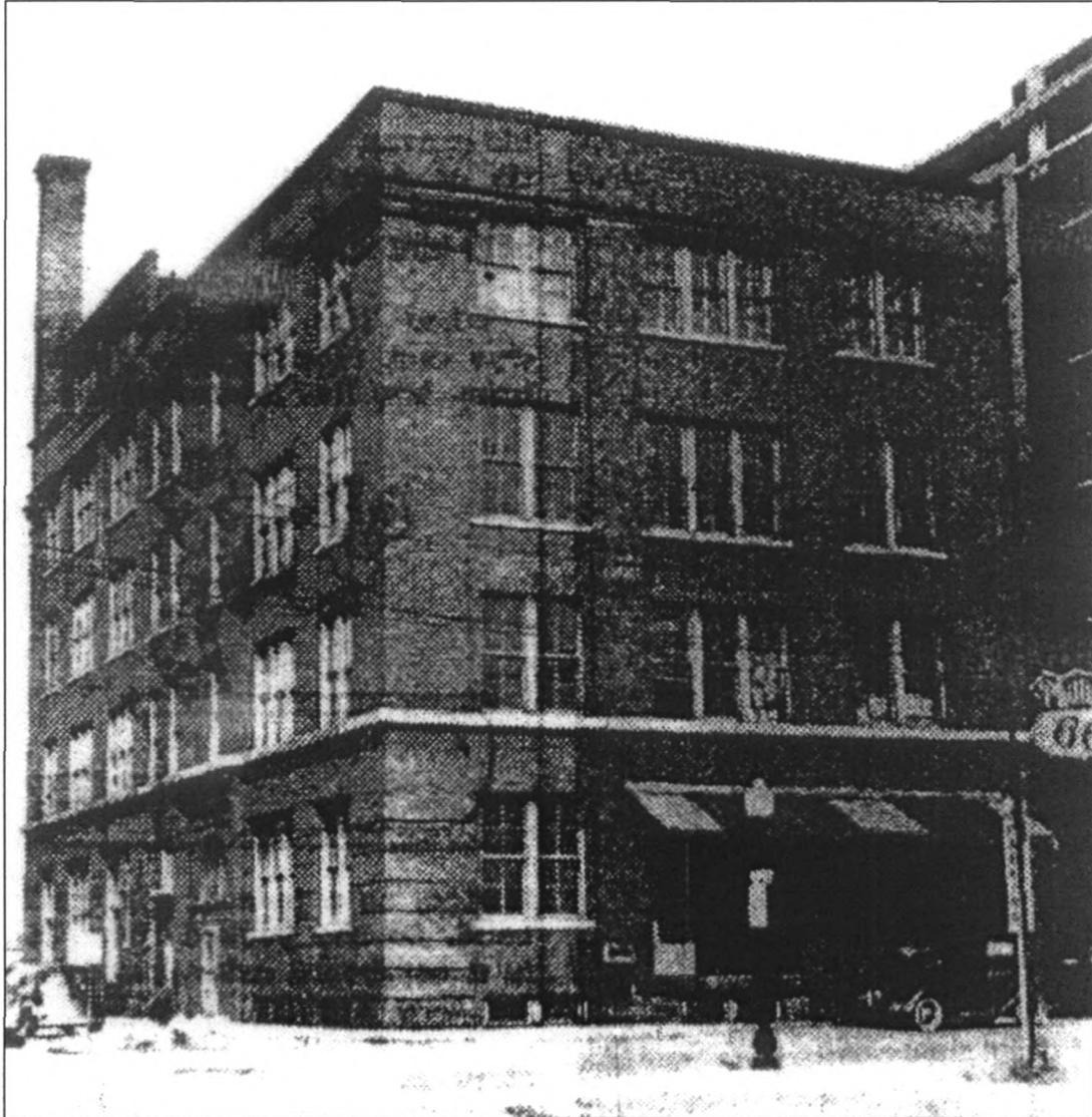
Figure 18: The building as it appeared when the Boyt Company purchased it, 1942, view west (Des Moines Tribune , June 16, 1942)
