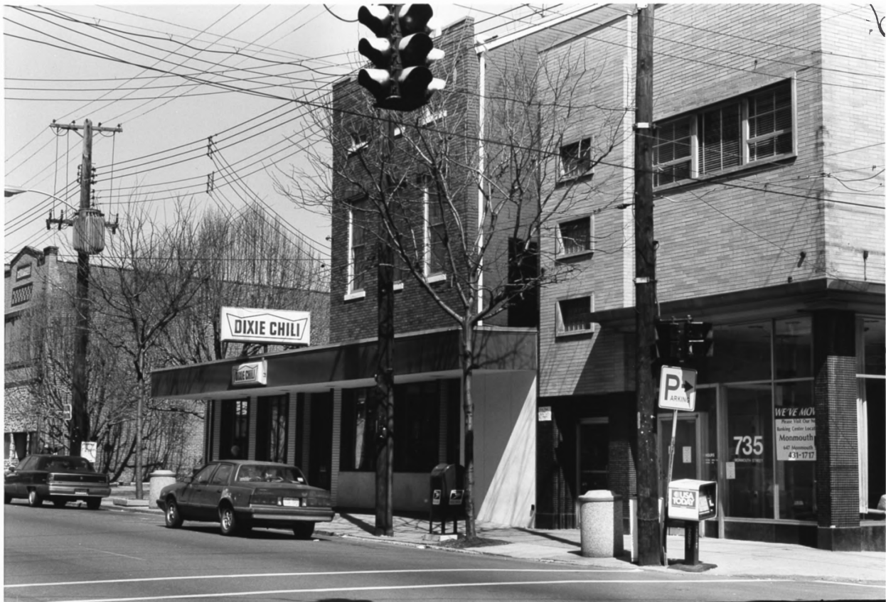
Monmouth St. Historic District Campbell Co., KY photo
