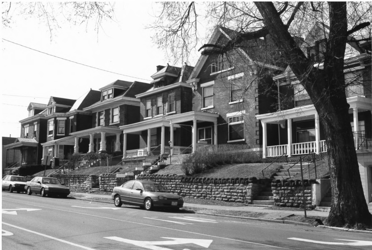
Monmouth St. Historic District Campbell Co., KY photo 1
