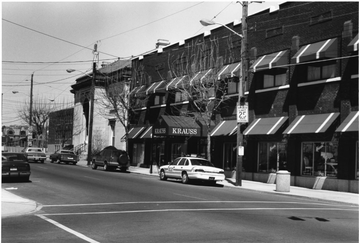
Monmouth St. Historic District Campbell Co., KY photo 2
