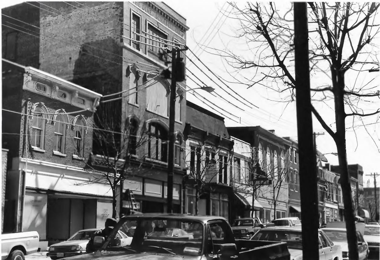
Monmouth St. Historic District Campbell Co, KY photo 6
