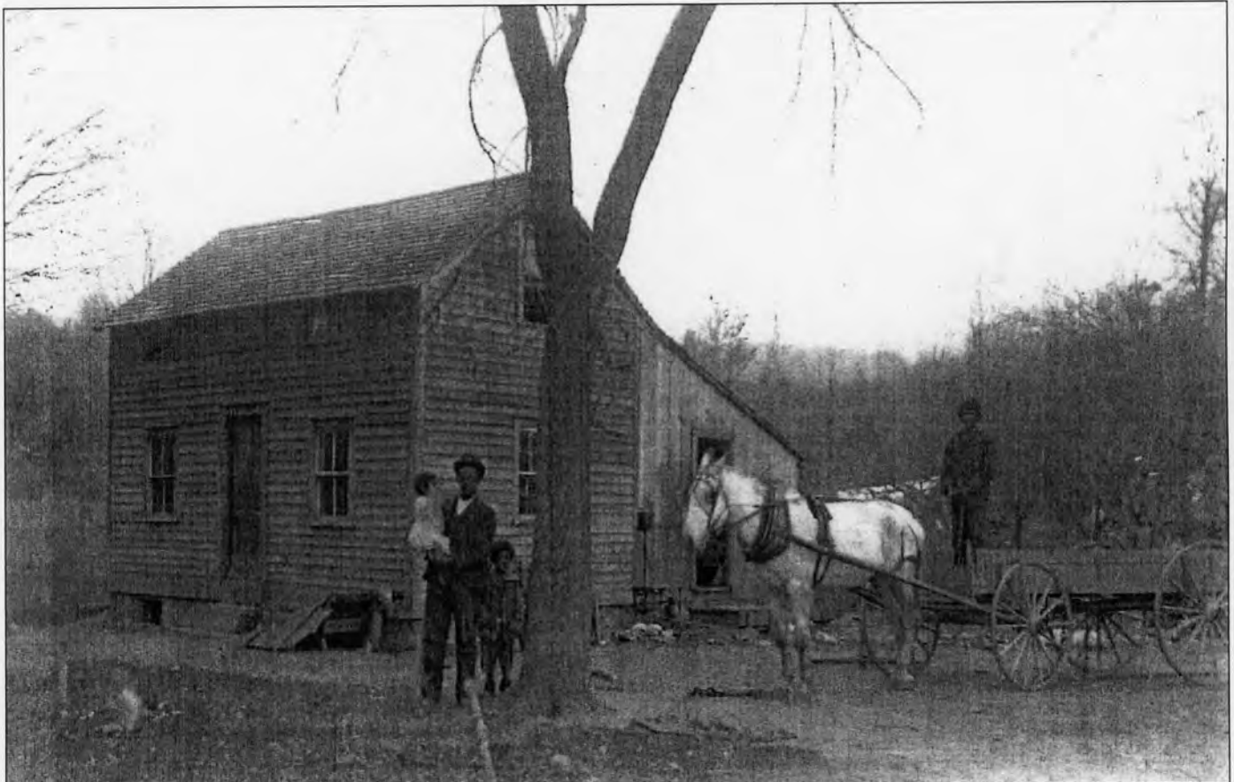
Fig.1: View of Fitch-Hoose House from southeast, c. 1900. Source: Ashfield Historical Society Photograph Collection.
