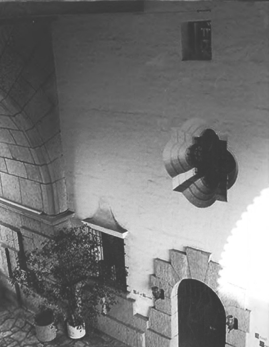
SANTA BARBARA COUNTY COURTHOUSE Santa Barbara, California Interior of main arch looking towards Service Annex Photo by Robert Ooley, 10/03
