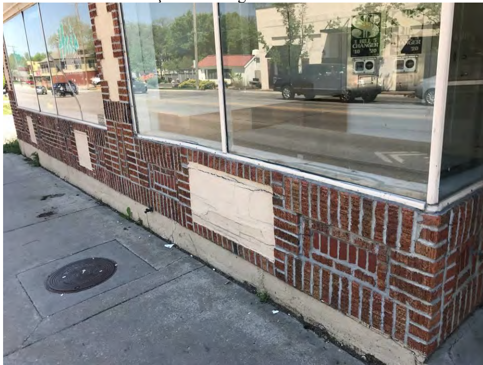
Photo 15: North Façade Looking Southeast at Storefront Brick Bulkhead
