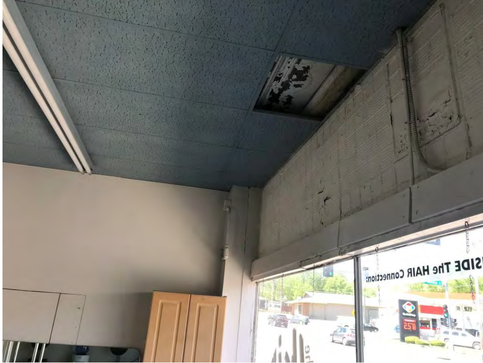
Photo 10: First Story Transom Over East Storefront and Tin Ceiling Above Modern Ceiling
