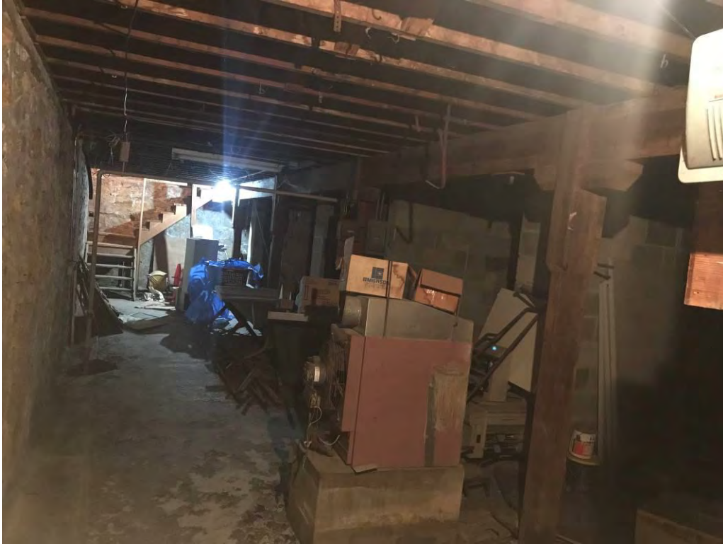
Photo 12: Basement East Area Looking South
