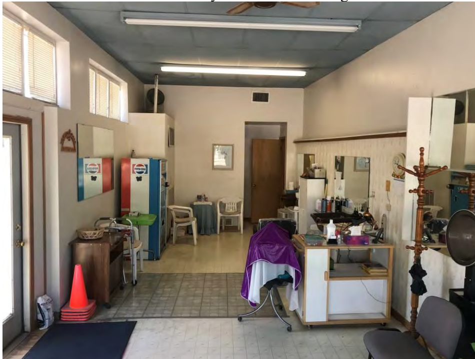
Photo 9: First Story East Area Looking South
