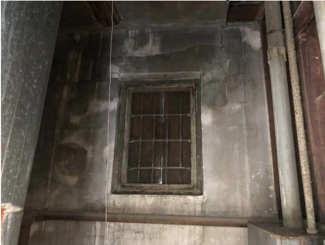
Photo 13: First Story at Southwest Corner Looking West
