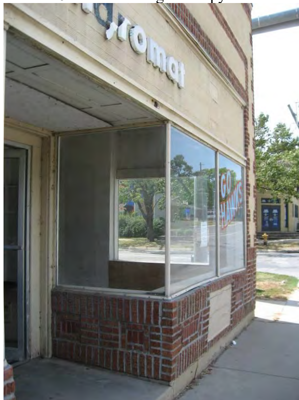
Photo 7: North Façade Recessed Entry Looking West-Southwest
