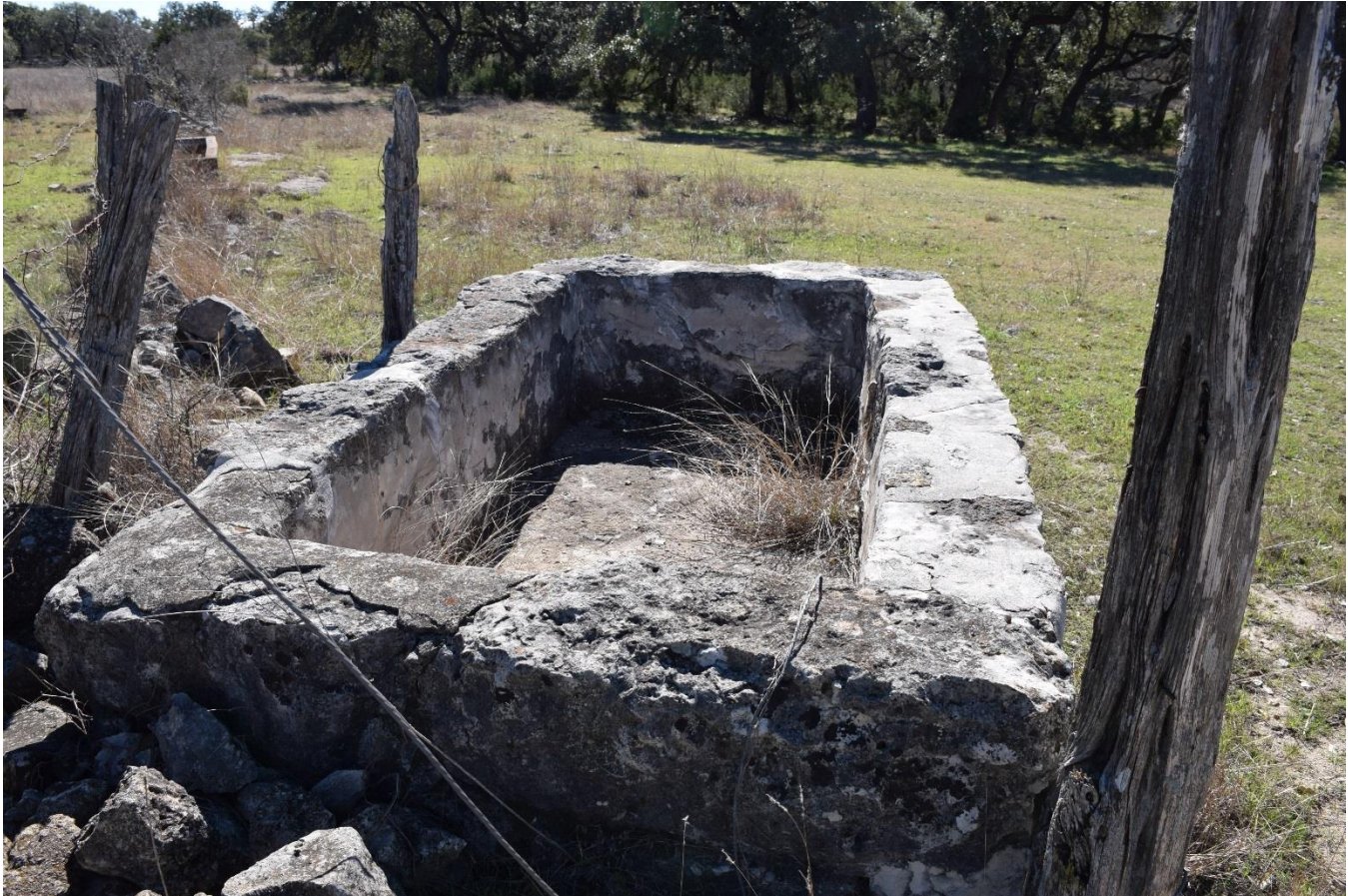
Photo no. 17. View of stone dipping vat (RID aa) on Kneupper Homestead. View facing southwest.
