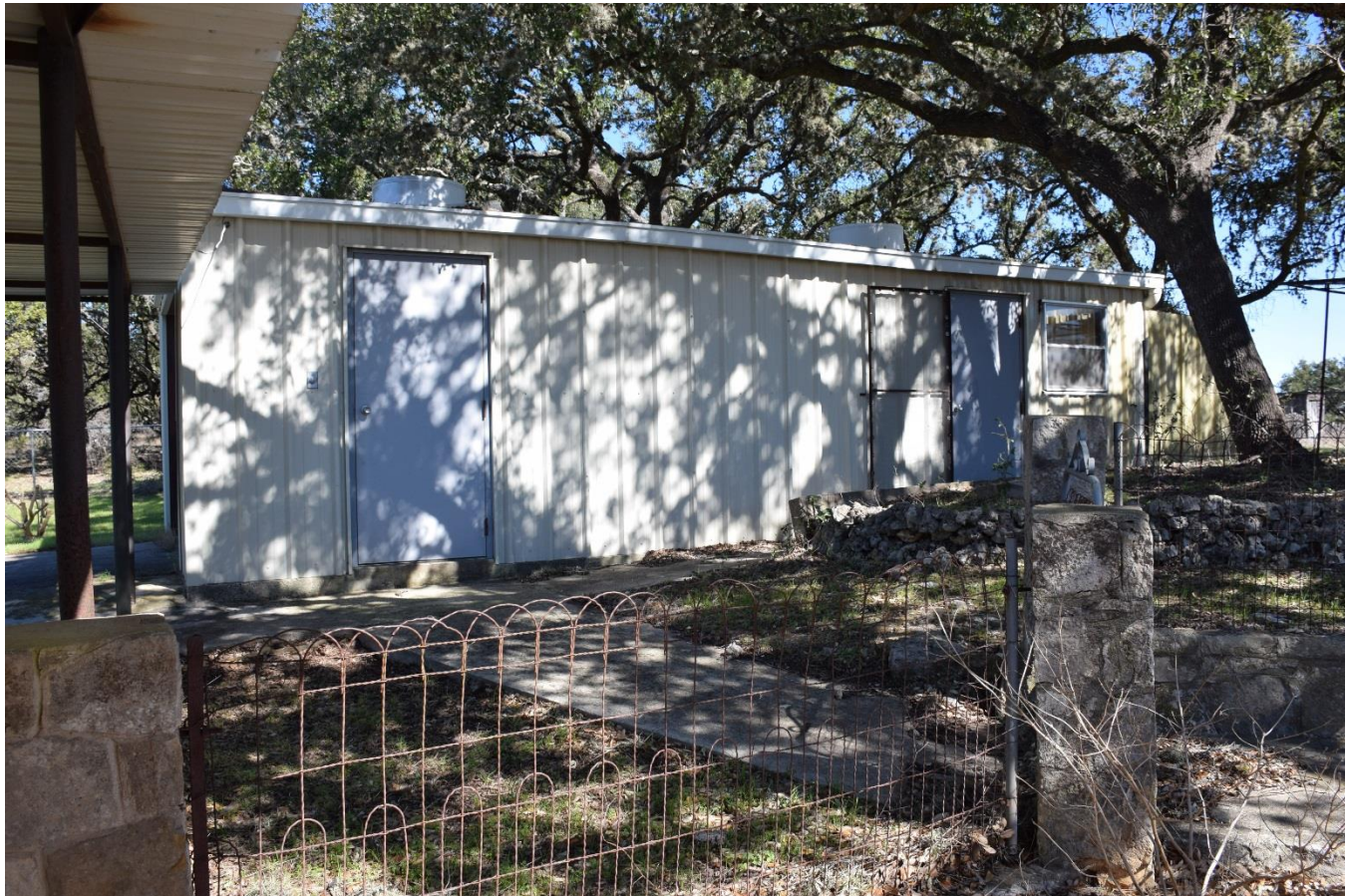
Photo no. 34. View of non-contributing garage (RID d) on Kunz Homestead. View facing northeast.
