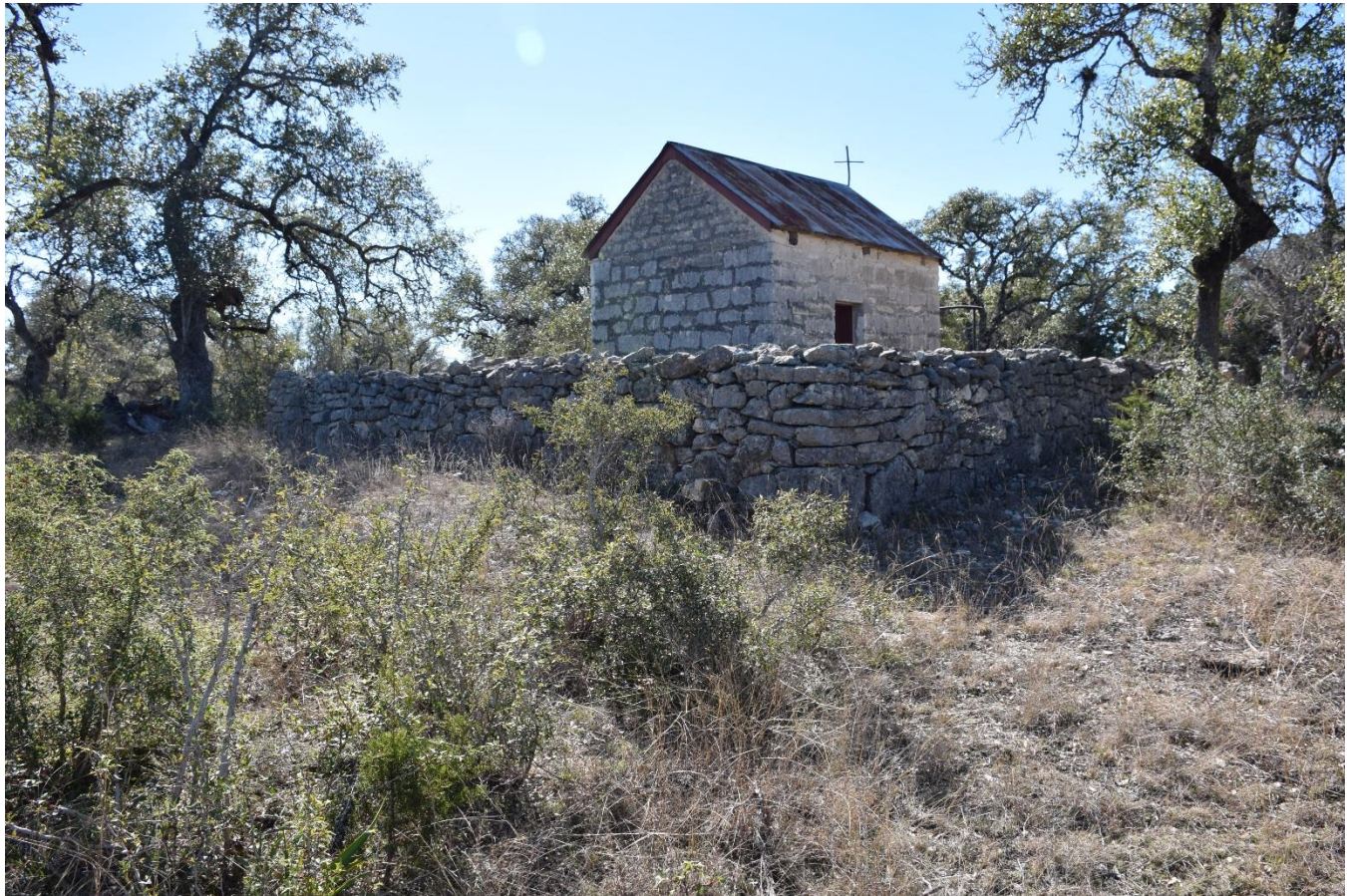
Photo no. 29. Contextual view of Kneupper Chapel (RID ff) and stone fencing (RID ii). View facing southeast.
