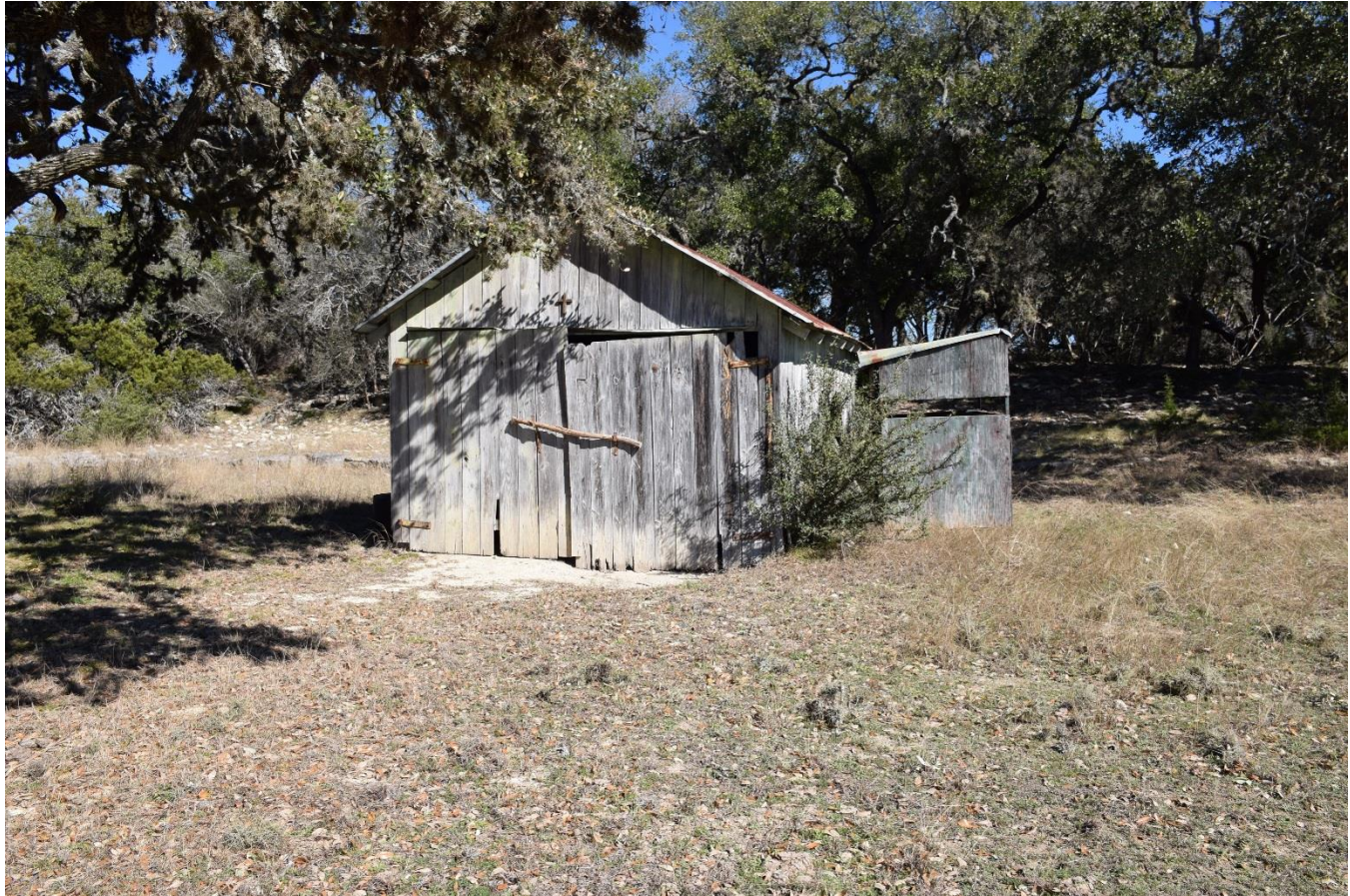
Photo no. 16. View of shed (RID ee) on Kneupper Homestead. View facing east.
