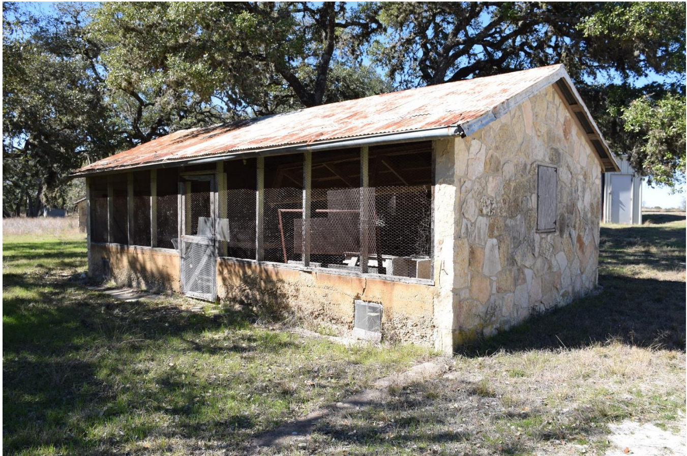
Photo no. 28. Oblique view of chicken house (RID n) on Kunz Homestead. View facing northwest.
