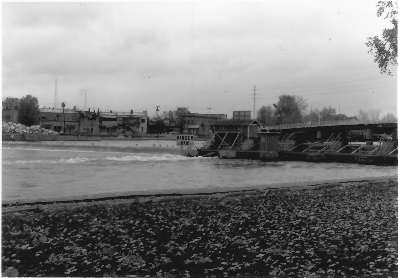
Menasha Dam, Menasha, Winnebago County, Photo #1 of 1
