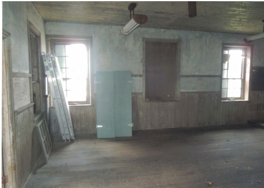
Photo #10—This interior photo view is looking west across the interior classroom. Note the full survival of the 1859 flooring, wainscoting, coat and hat racks, plaster, and wood ceiling. Two of the original 9 over 6 window sash still survive, however, the central window opening is missing its original 9 over 6 window sash.
