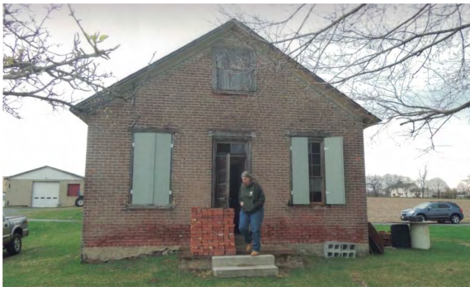
Photo #2 – This photo view records the current condition of the southern elevation. The overall design of this historic schoolhouse is of a Late Greek Revival style. The design—both exterior and on the interior—is very similar to the “Class 1, No. 1, Houses for Upgraded or Primary Rural Schools,” as shown and described in the 1855 Pennsylvania School Architecture: A Manual of Directions and Plans for Grading, Locating, Construction, Heating, Ventilation and Furnishing Common School Houses , by Thomas H. Burrowes.
