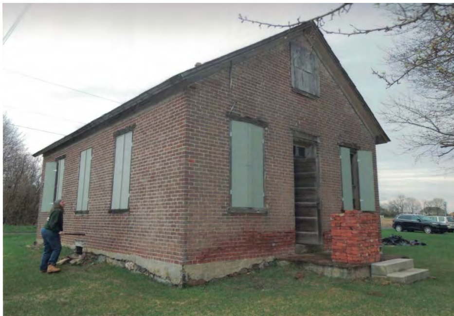
Photo #1 – This photo view shows the southwest corner elevation of the 1859 Edelman Schoolhouse. The stacked 19 th century bricks on the front steps are being used to restore the east elevation masonry. The temporary shutters over each window have been carefully installed by Moore Township to secure all windows and prevent further rain and snow penetration to the well-preserved interior.
