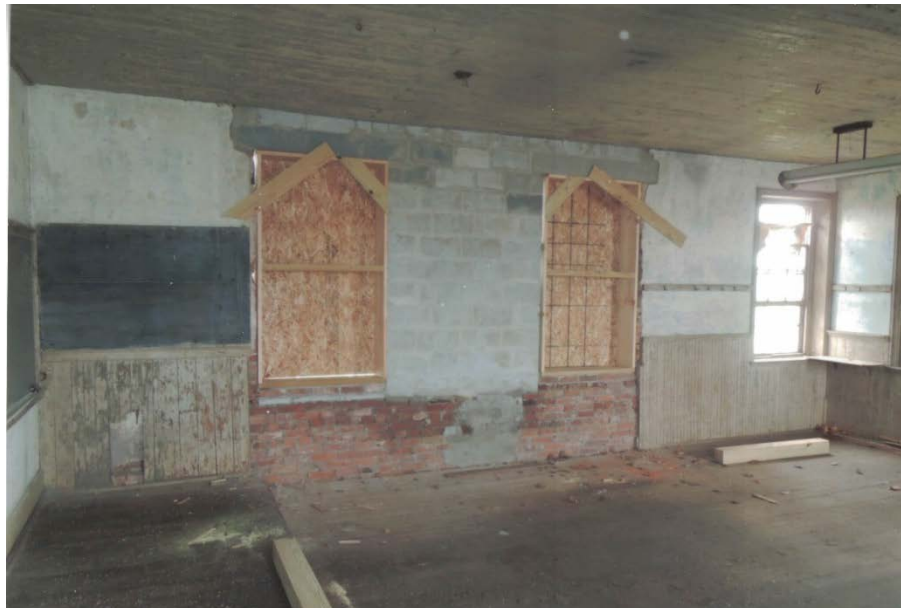
Photo #12—This interior photo view is looking east onto the interior of the east elevation wall of the main classroom. This current view shows the very recent restoration of the central portion of this wall. This effort involves the external brick masonry restoration and the two window openings that were removed after 1958 when a farmer opened up this area to allow farm vehicles to enter this space. The accurate restoration of these two windows is being planned, along with restoration of missing wainscoting and plaster work matching the original.
