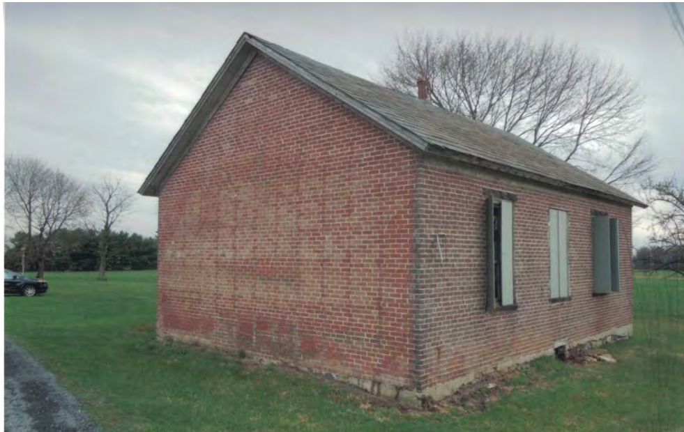
Photo #3—This photo view looks southeast onto the northwest corner elevation of the building. The roof may still retain the original slate roof, but requires final confirmation. The slate appears by its physical character to be from the once extensive slate quarries located in nearby Chapman Quarries. The paint on the roof's cornice is of a typical linseed oil based white color, and is possibly original from 1859, but this also requires final confirmation. The use of white paint color reflects an aesthetic preference of the Greek Revival style.
