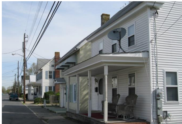
Fleming Street Streetscape east side looking north
