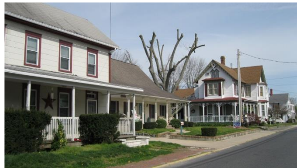
Fleming Street Streetscape west side looking north
