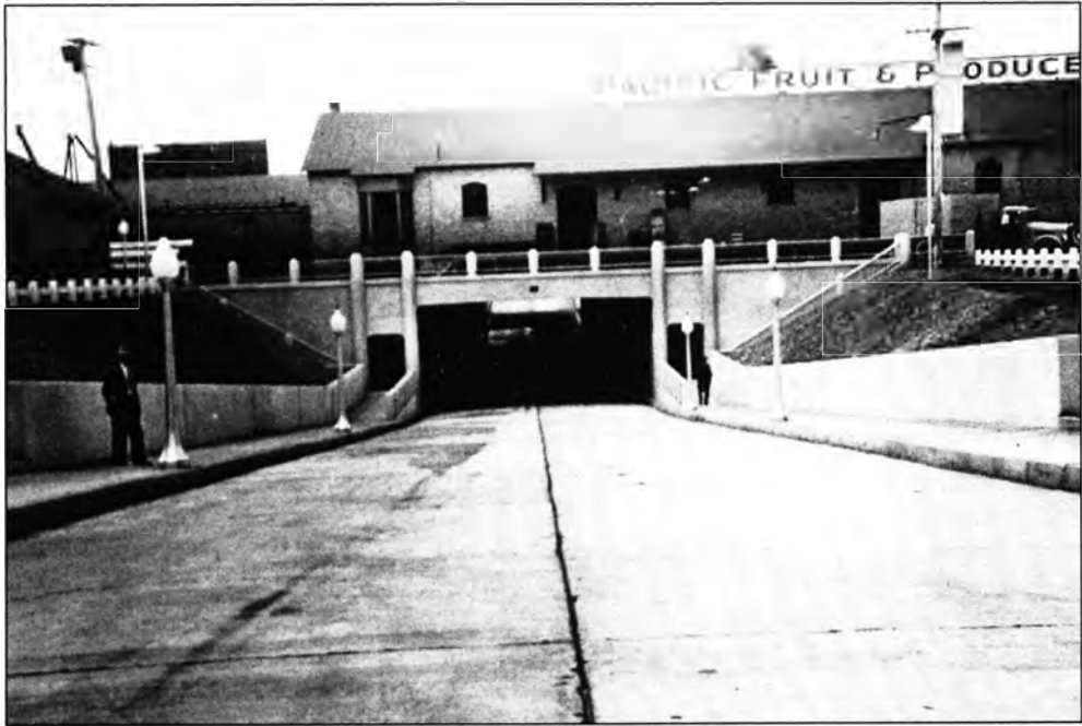
Photo 0001. Orange Street Underpass. North elevation. View to the south.
