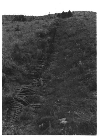
El Paso & Southwestern Railway Water Supply System (Bonito Pipeline) vicinity of Nogal, Lincoln Co., New Mexico Lane Ittelson, August, 1978 NOV 2 1979 exposed section of 1908 flat steel wrapped pipe; photo looking south Photo #293 SEP 18 1979
