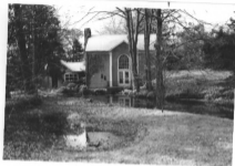
Studio building, looking W. neg. file # 19844-23 slide
