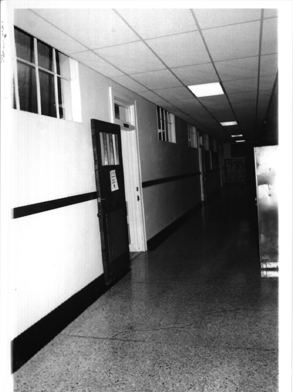
PROTECTION HIGH SCHOOL, COMANCHE COUNTY, KANSAS #12
