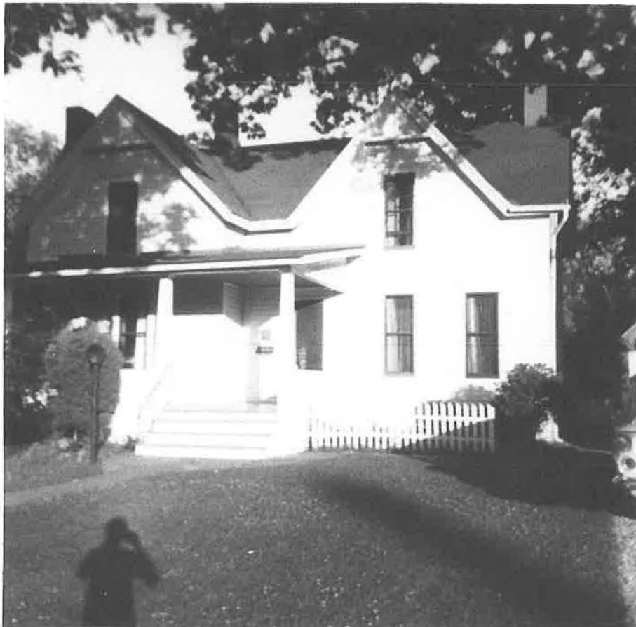
Figure 11. HISTORIC IMAGE – 1551 B Avenue NE – Ashel & Alice Moore House - ca.1971
