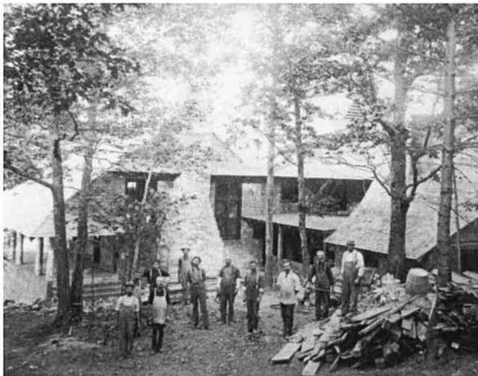
Fig. 14: The Ledge (#6) under construction, 1901. Courtesy Laura Nash
