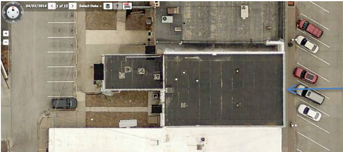
Figure 2: Aerial pictometry photograph showing the subject building (arrow), 218 Fifth Street, West Des Moines. (Polk County Assessor's Office map, 2015-16)
