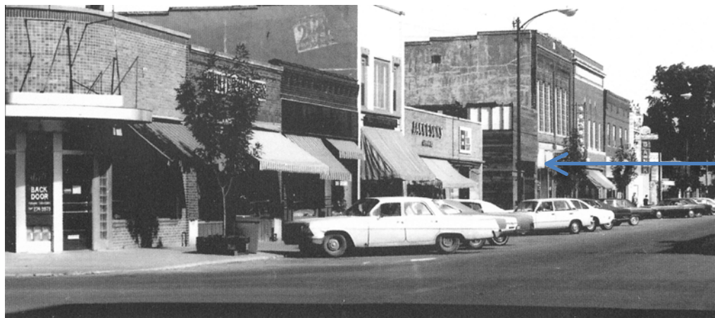
Figure 12: 1975 view of west side of Fifth Street from Maple looking north to Elm. Arrow points to the subject building. Note the Masonic Lodge to the right is now in its reduced two-story configuration. South elevation of subject building appears to show cracking in stucco/parging. (McCue: 107)
