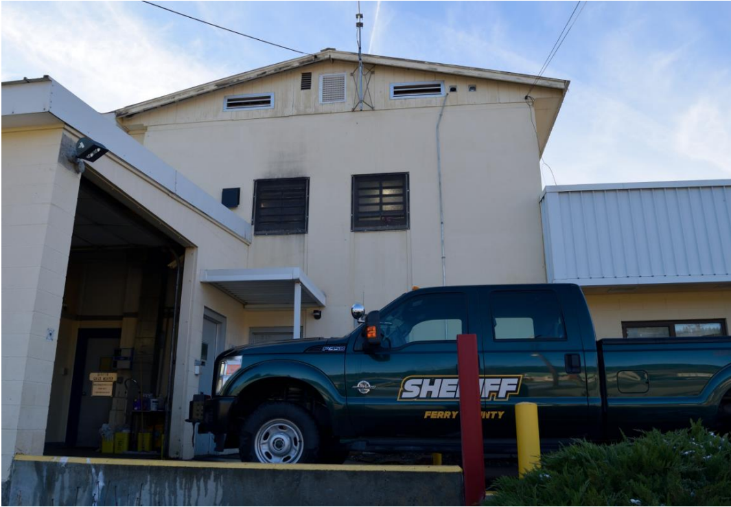
24 of 30: East wall of the jail (2). The highest section is the original 1939 structure.
