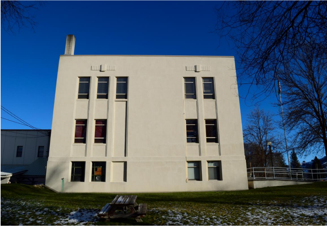
2 of 30: West façade of Ferry County Courthouse,(1) boiler room and 1973 additions on the left
