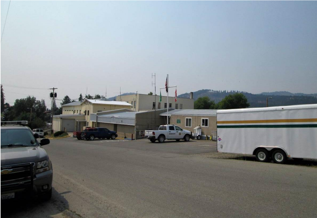
26 of 30: Sheriff's office (3) and jail (2) from the northeast.
