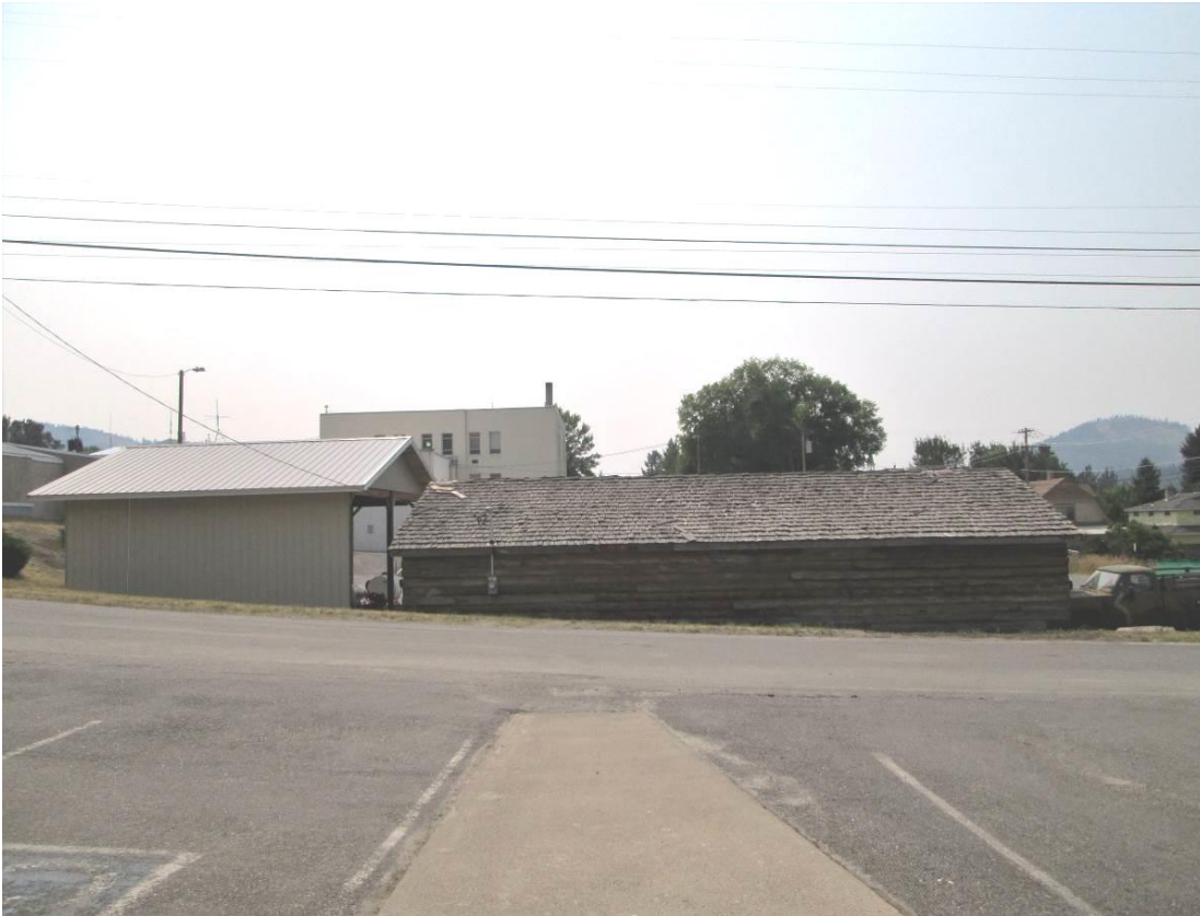
30 of 30: Rear of structures 6 on the left and 7 on the right
