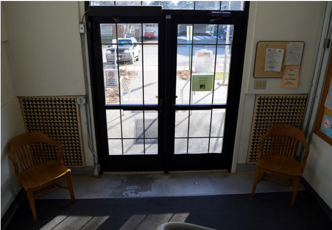
6 of 30: Looking out the main (S) door of the Ferry County Courthouse. The radiator grilles on either side correspond to the architect's drawings in the margin of the 2nd floor drawing.
