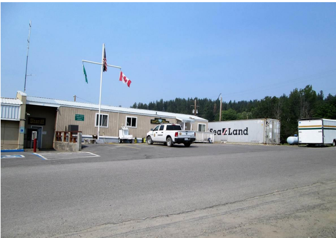
27 of 30: Junction of the Sheriff's office on the left and the 911 center on the right. Originally separate buildings, they make up building 3.
