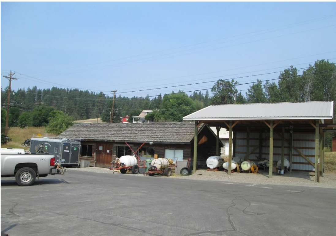
29 of 30: Open sided shed (6) on the right and former Historical Society (7) on the left.
