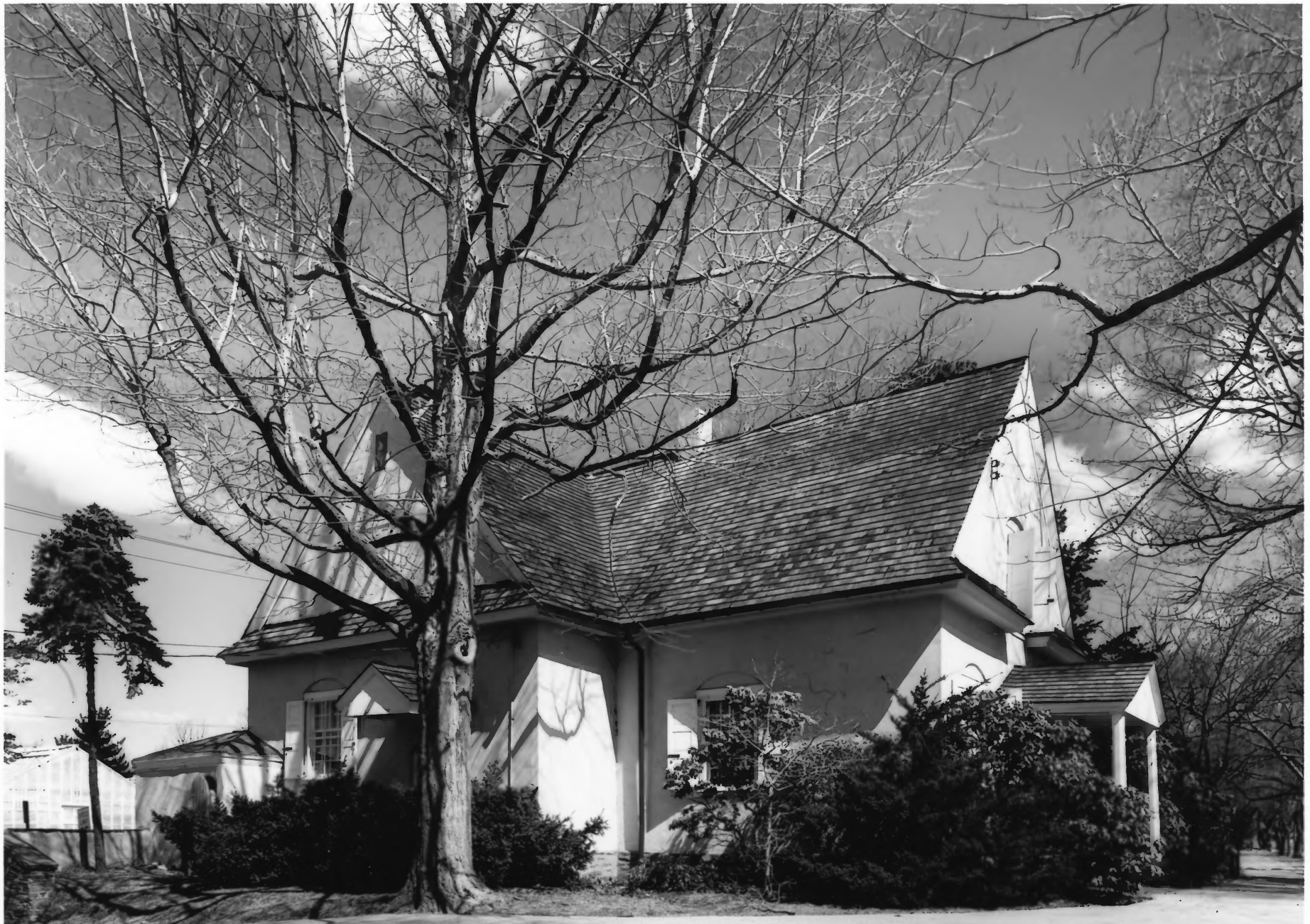
Photo #2 Merion Friends Meeting House Montgomery County, Pennsylvania South and west elevations Anthony S. Bley, 1987
