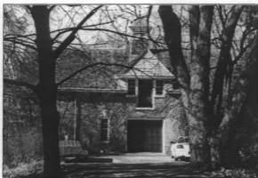
Carriage House, 325 Alpine, view west (Photo by J. Jacobsen, 2003)
