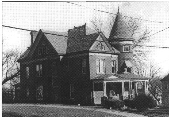
1045 West Third, view northeast (Photo by J. Jacobsen, 2003)
