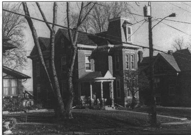
1057 West Third, view northeast (Photo by J. Jacobsen, 2003)
