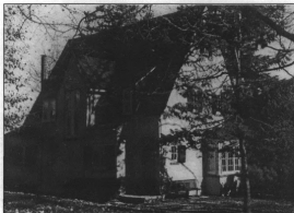
1087 West Third, view northeast (Photo by J. Jacobsen, 2003)
