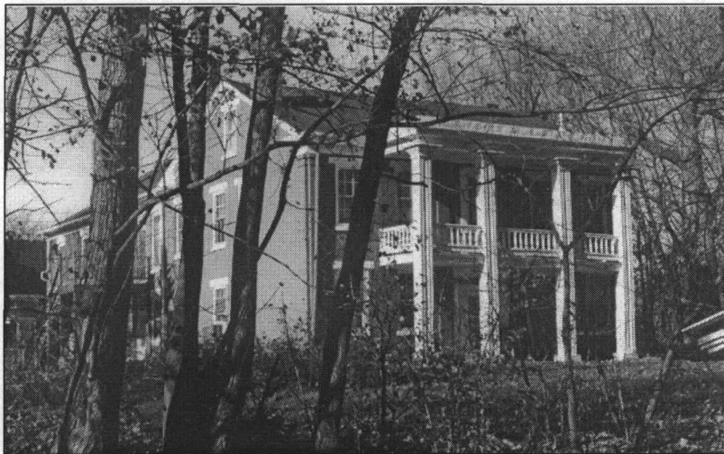
264 Alpine, original façade, view northwest (Photo by J. Jacobsen, 2003)
