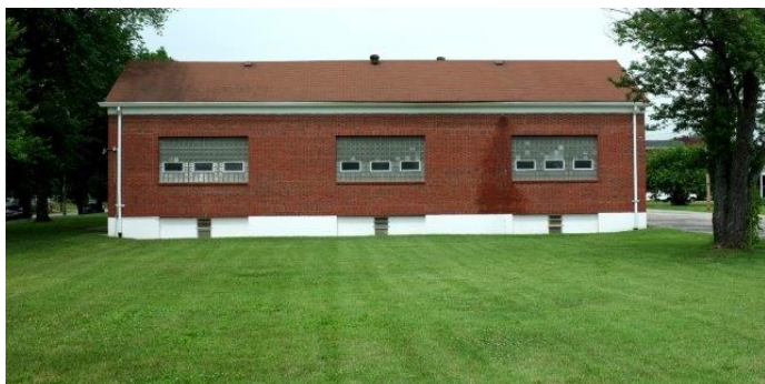
East End wall
