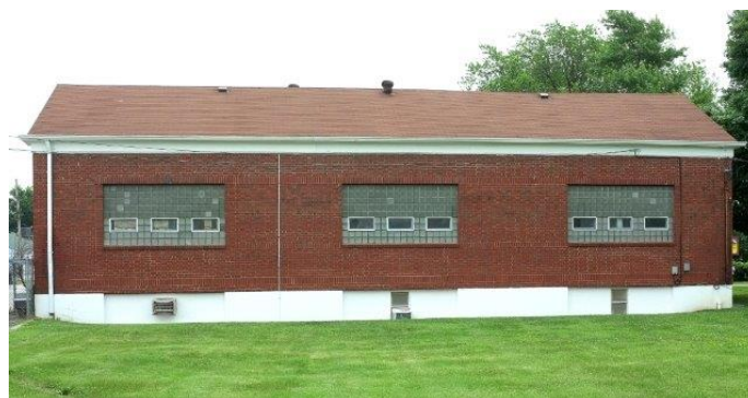
West End wall
