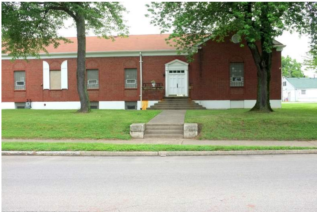
East End facade
