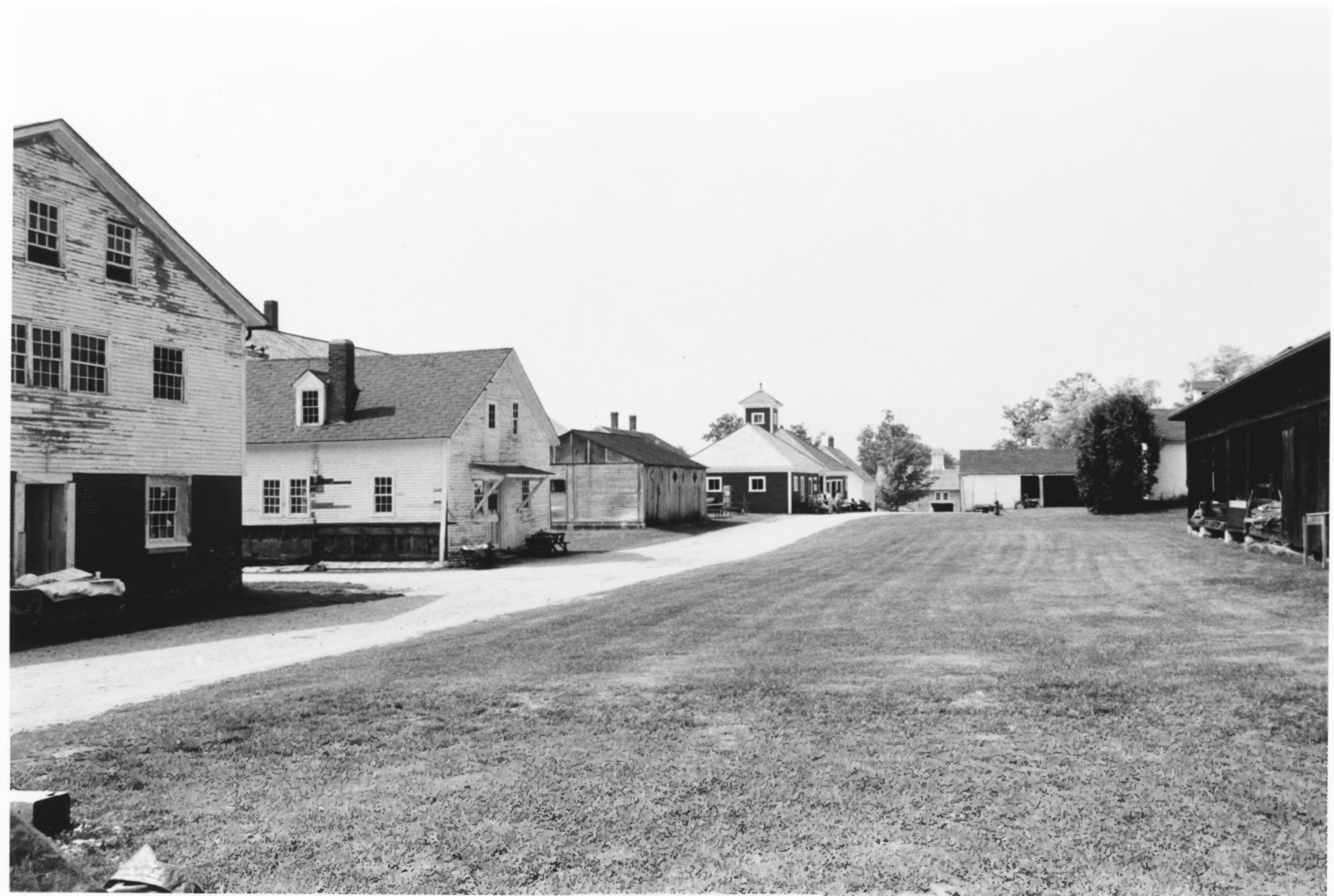
Canterbury Shaker Village Canterbury, N.H. Utility Buildings Photo: Lisa Mansolf, 1992
