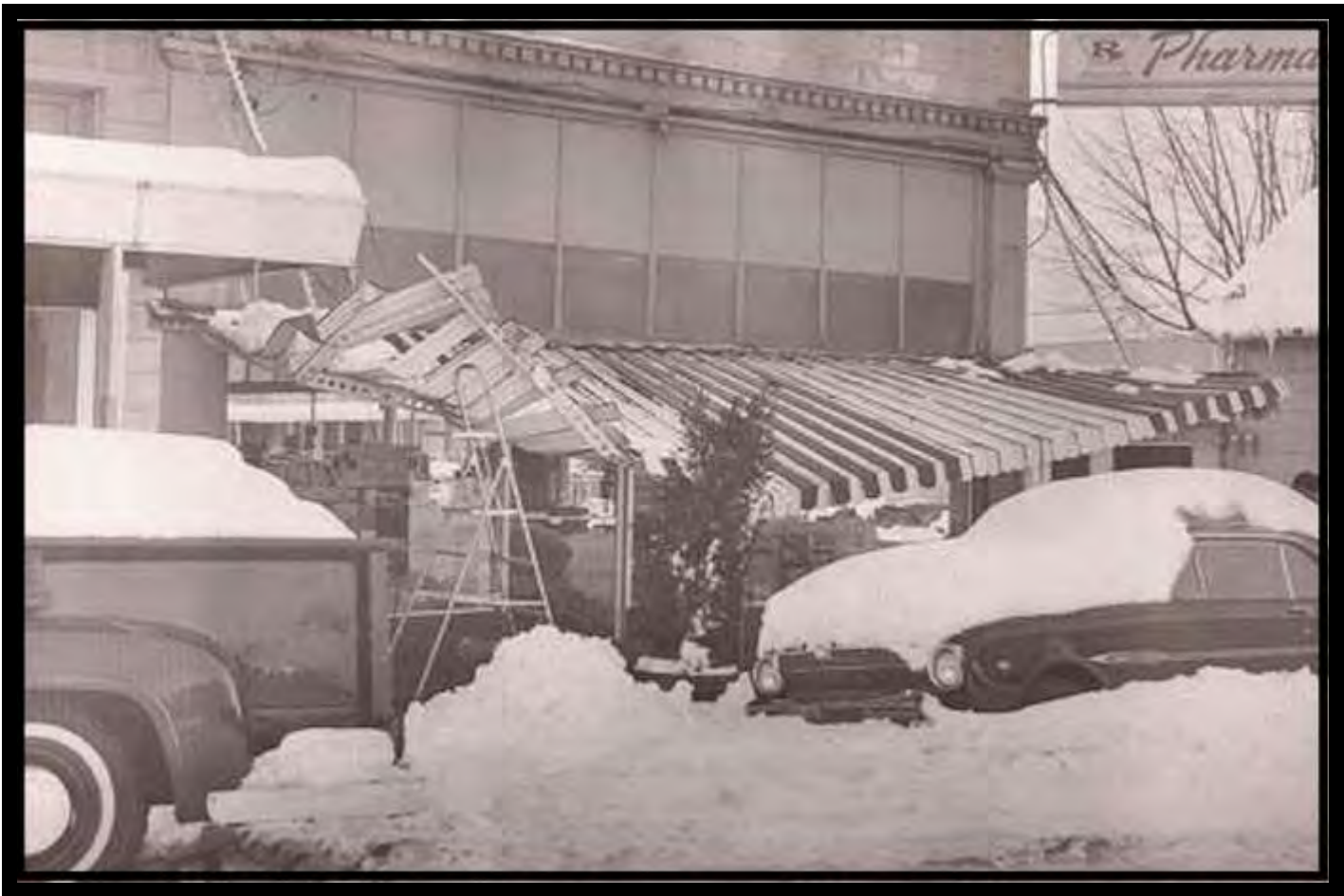
Figure 22: This photo shows the transoms painted and the dentil frieze sill in tact. View is the east side of Third Ave looking north, northwest.
