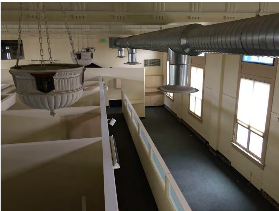
45. View from the mezzanine of the office partition infill at the center of the third floor. Painted gypsum wallboard has been applied over original plaster perimeter wall.
