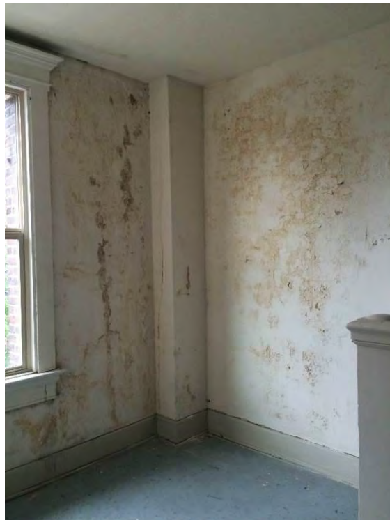
35 & 36. West stair hall and adjacent water-damaged plaster at southwest corner. Note also the partition, left, fitted against an original window frame.
