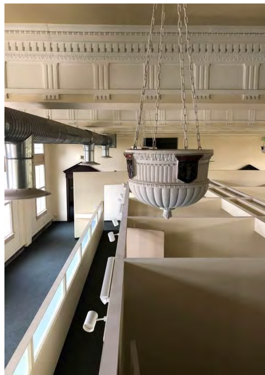
42. Looking east at the inserted office partitions and portion of the north perimeter wall, showing an example of the chain-suspended light fixtures featuring a Knights of Columbus seal.
