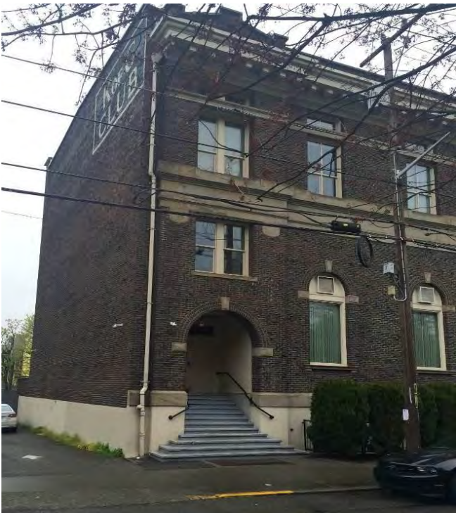
7 Looking north at the southwest corner and KOC members only entry, south facade (RAG).
