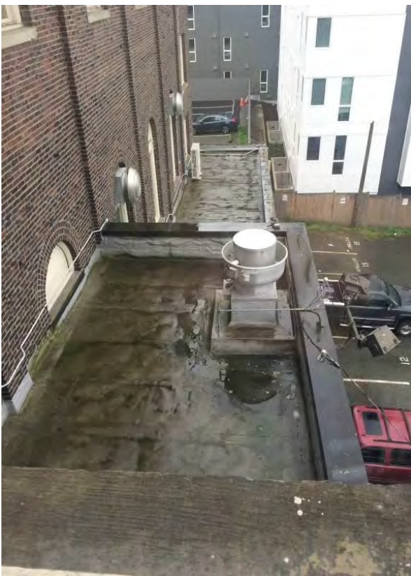
14. Below right, northwest setback and roofs.
