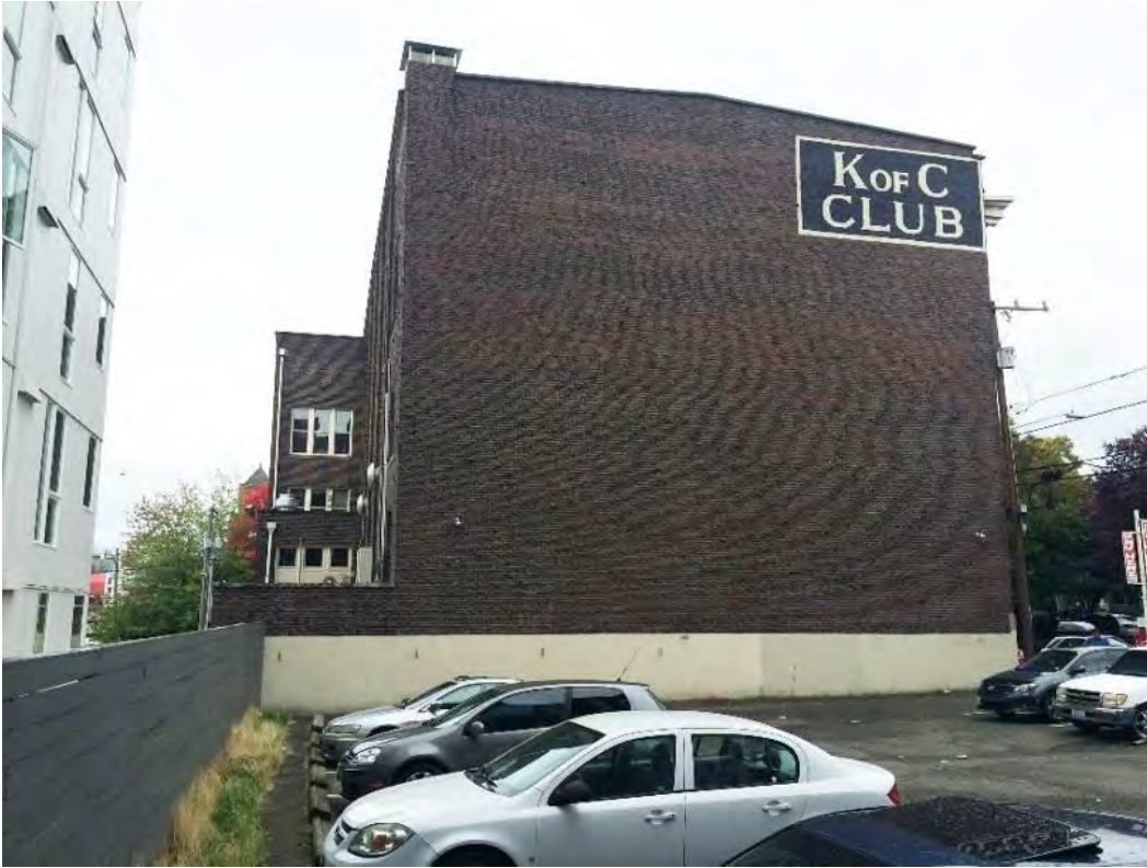
6. Below, looking east at the west facades.
