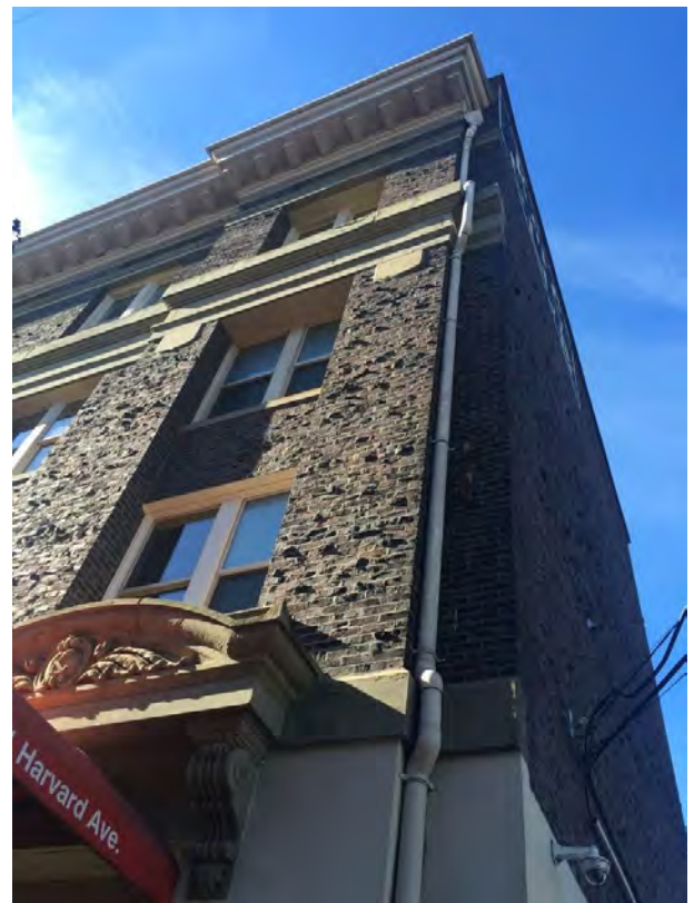
15. Above left, a detail view of the clinker brick at the northeast facade corner and portion of east facade.
