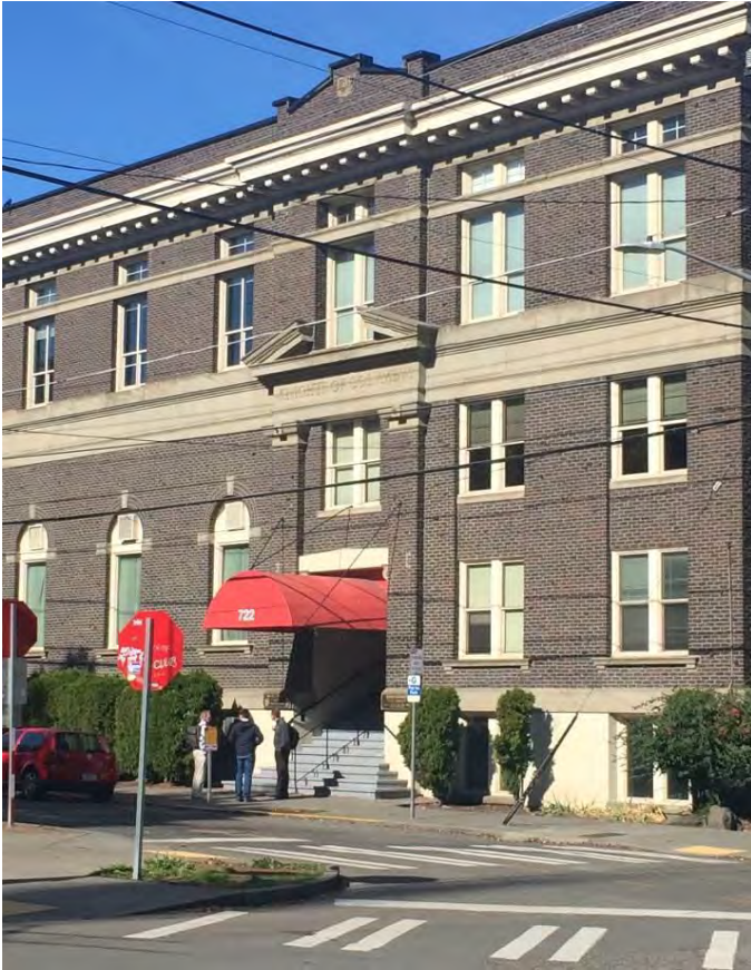
2. Above, the primary entry on the south facade.
