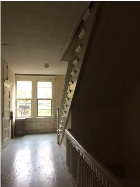
35 & 36. West stair hall and adjacent water-damaged plaster at southwest corner. Note also the partition, left, fitted against an original window frame.
