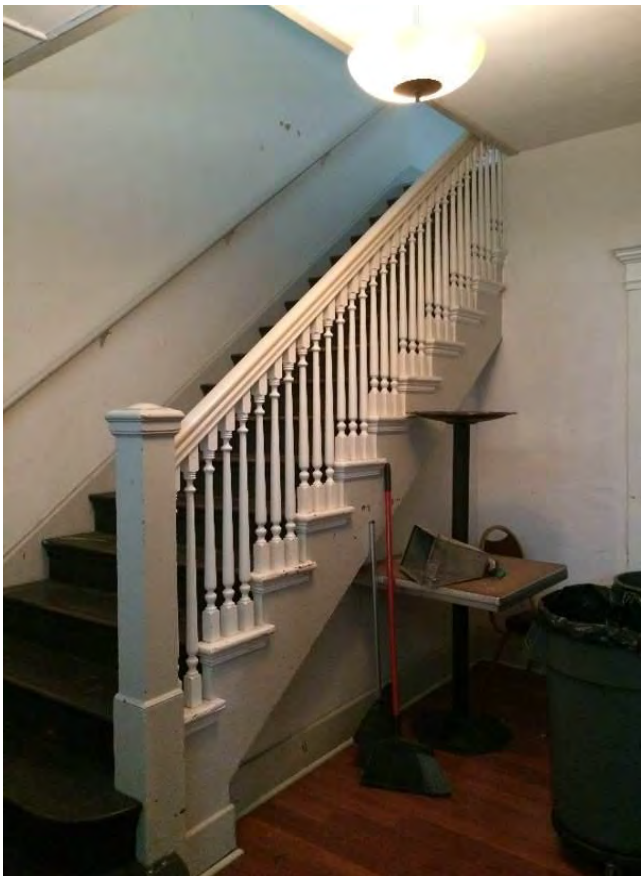
32. West stair from second to third floors.
