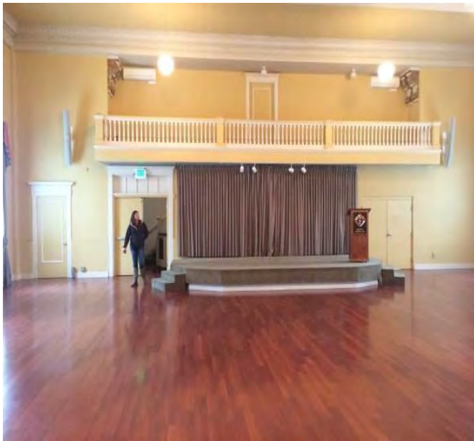
28. Left, a detail view showing the enclosed mezzanine and northwest doors at the west end of the ballroom, and original window openings in the south (left) and infilled semi-circular transom windows in the north and south perimeter walls.
