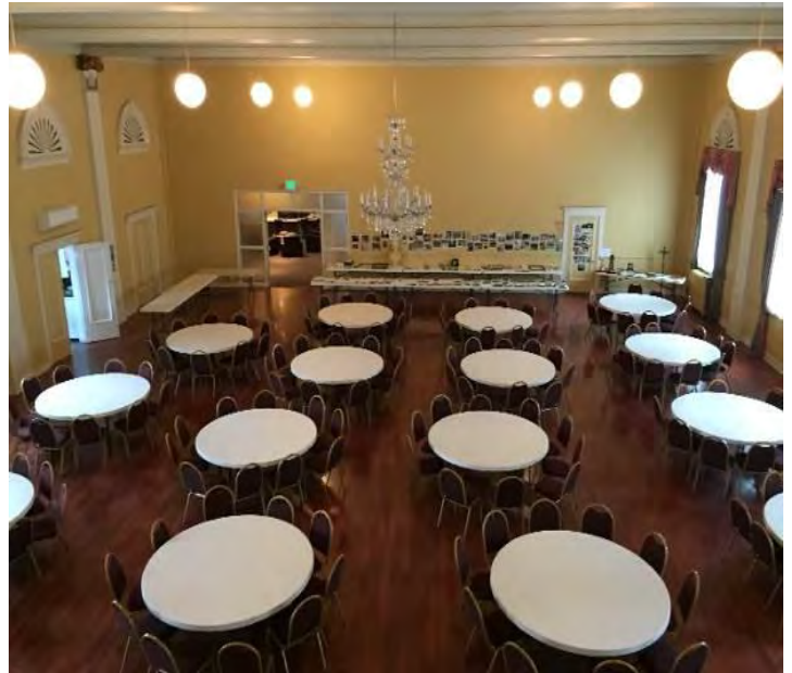
28. Left, a detail view showing the enclosed mezzanine and northwest doors at the west end of the ballroom, and original window openings in the south (left) and infilled semi-circular transom windows in the north and south perimeter walls.
