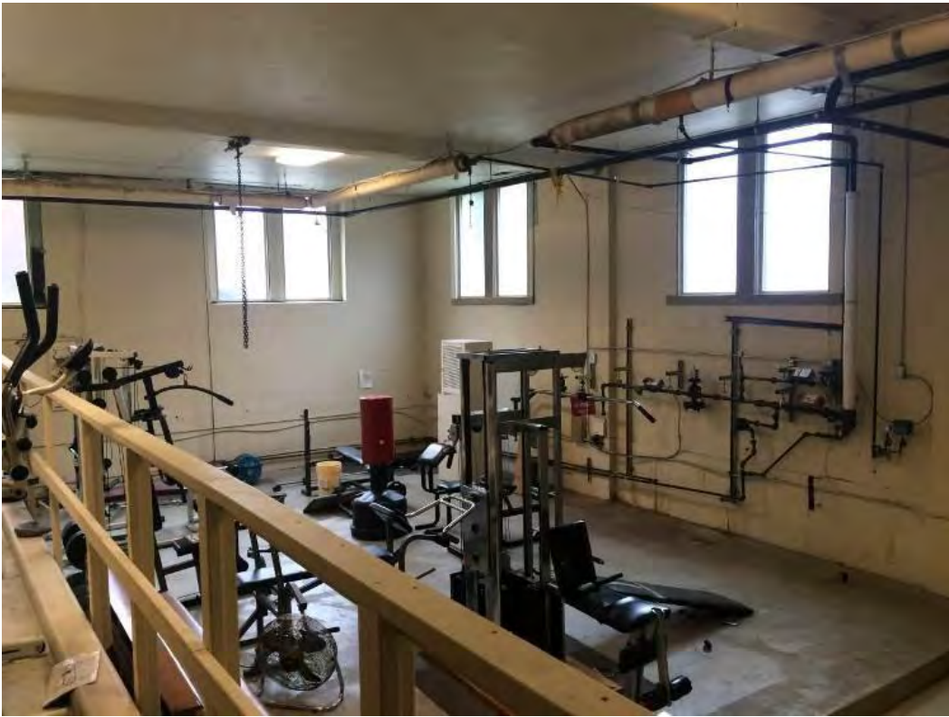
20. Below right, former swimming pool room in the southeast corner of the basement, which was filled in the 1940s, and used subsequently as an exercise room.
