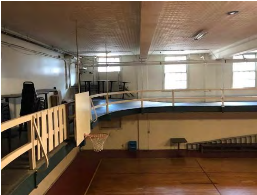
18. Looking south. The gym and running track in the basement gym.
