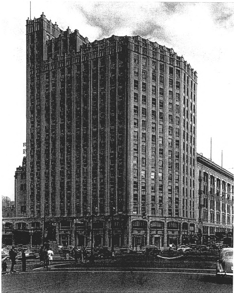
Historic Preservation Certification Application – Part I MEDICAL DENTAL BUILDING, 509 Olive Way, Seattle, King County, Washington 98101
