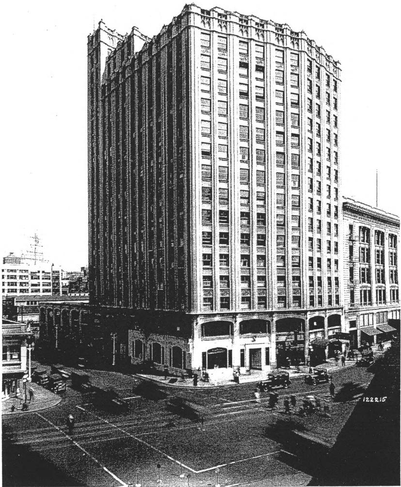
Historic Preservation Certification Application – Part I MEDICAL DENTAL BUILDING, 509 Olive Way, Seattle, King County, Washington 98101
