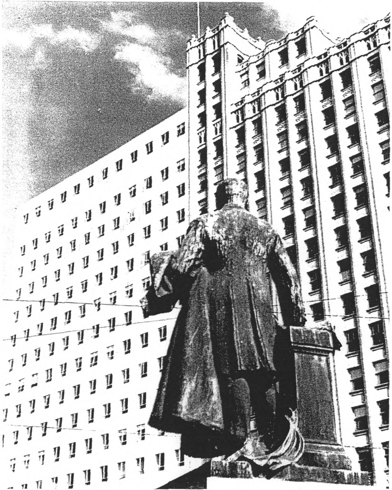
Historic Preservation Certification Application – Part I MEDICAL DENTAL BUILDING, 509 Olive Way, Seattle, King County, Washington 98101
