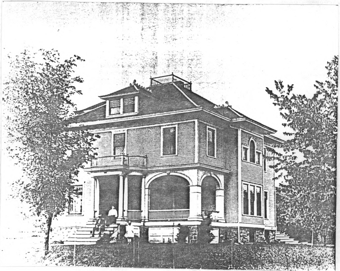
Original appearance of Alfred Hanson House, undated photo, view to west.
