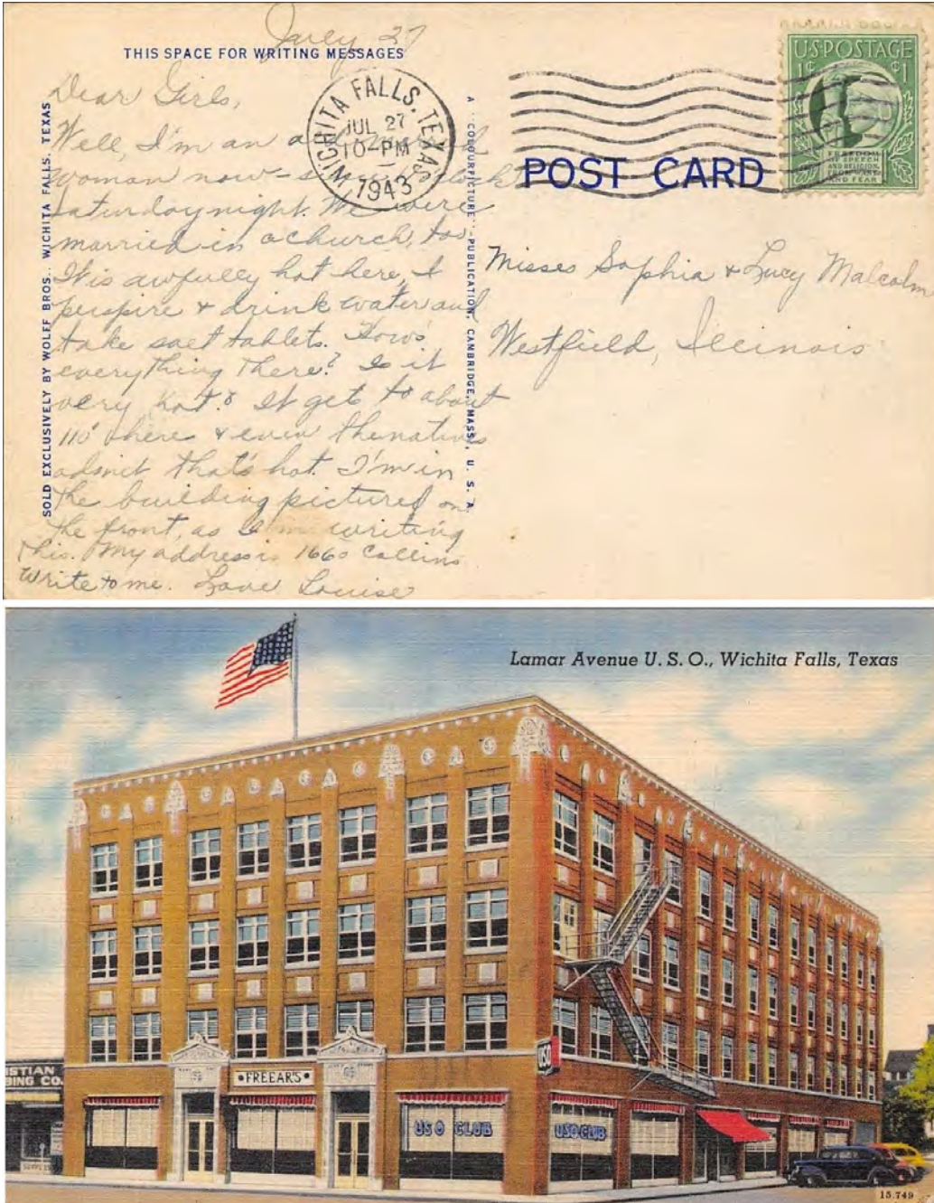
Figure 2: 1943 Post Card Image of the Freear Building
