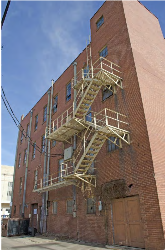
Photo 5 - Southwest (Rear) Elevation, view north.
