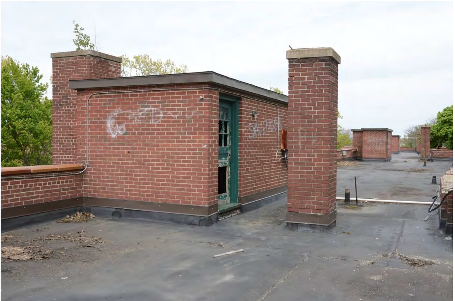
Roof access for Units 3-4-5.
