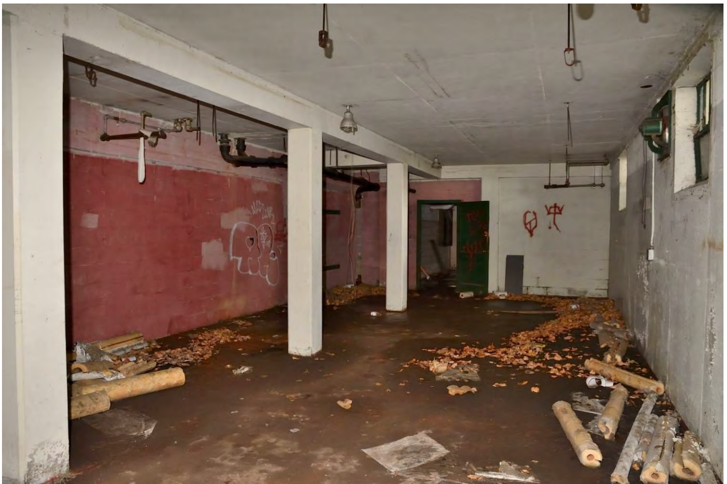
Basement craft room, unit 3.
