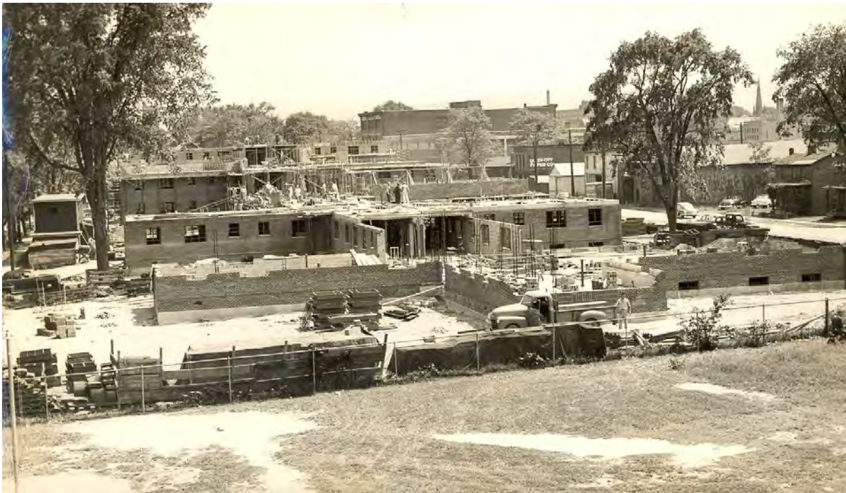
Construction photograph, ca. 1952.
