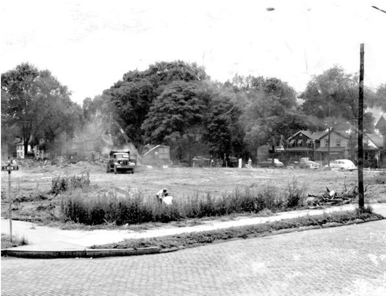
Demolition of Zion AME Church, Slabtown block, 1951.
