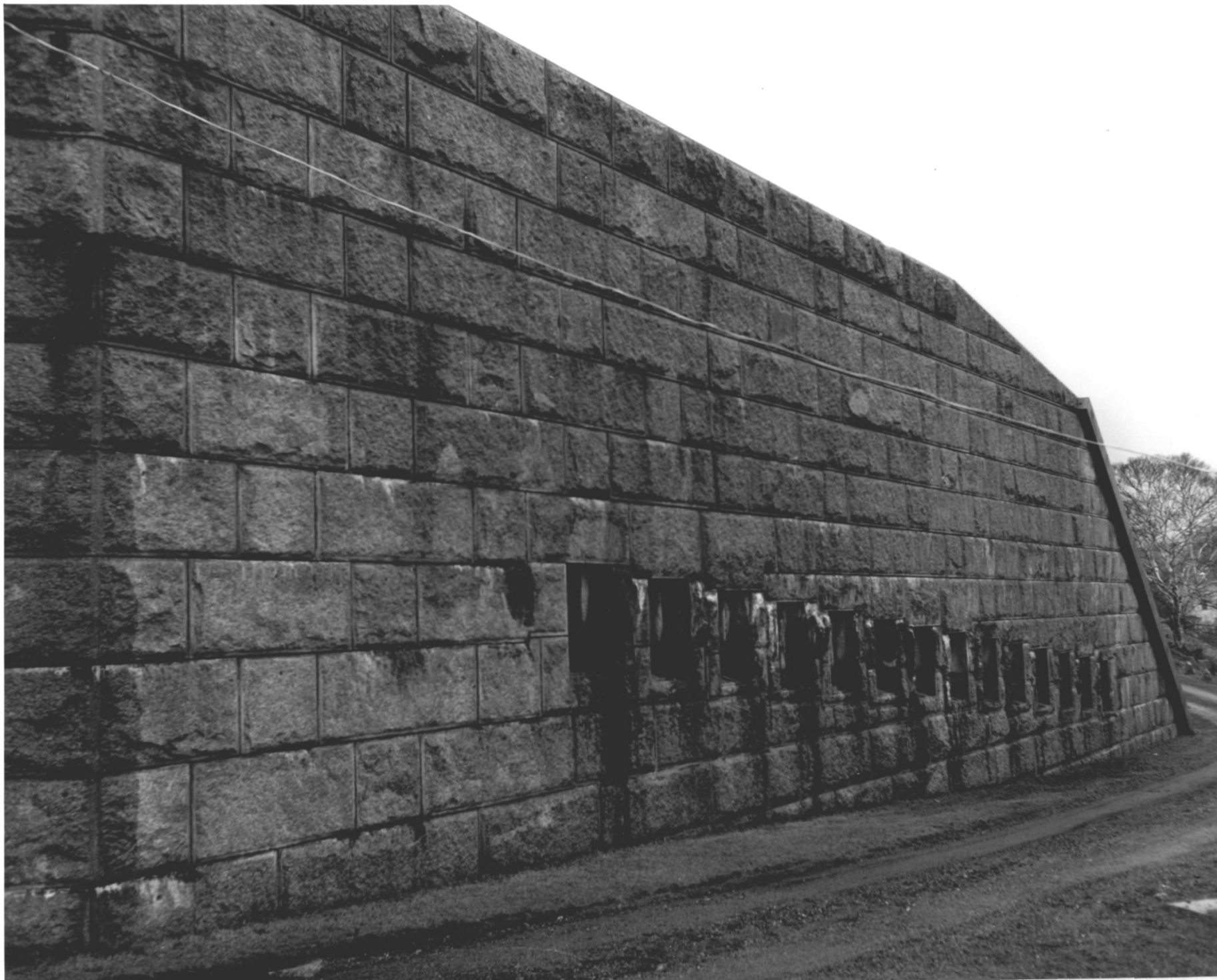
Fort Knox, Maine. Granite faced end of outer earthen wall.
